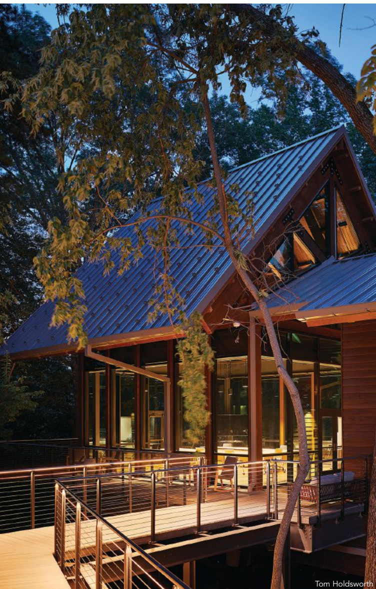
The treehouse and the rest of the buildings are connected by broad, steel-supported walkways that “float” above the forest floor.
