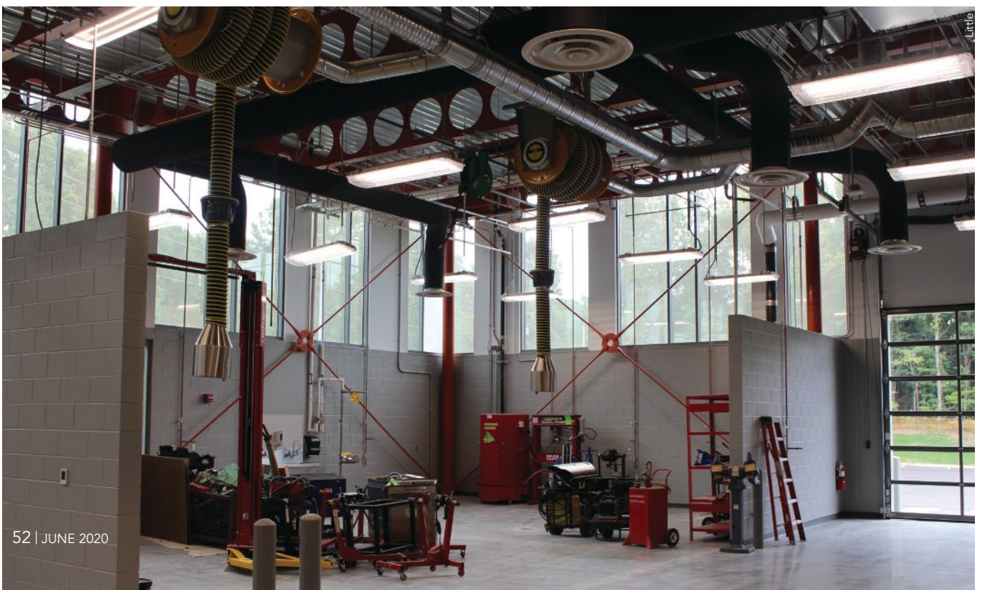
below: Rod X-bracing, round column isolation joints, and circular connection plates are all used to reinforce a round/cylinder design concept.
