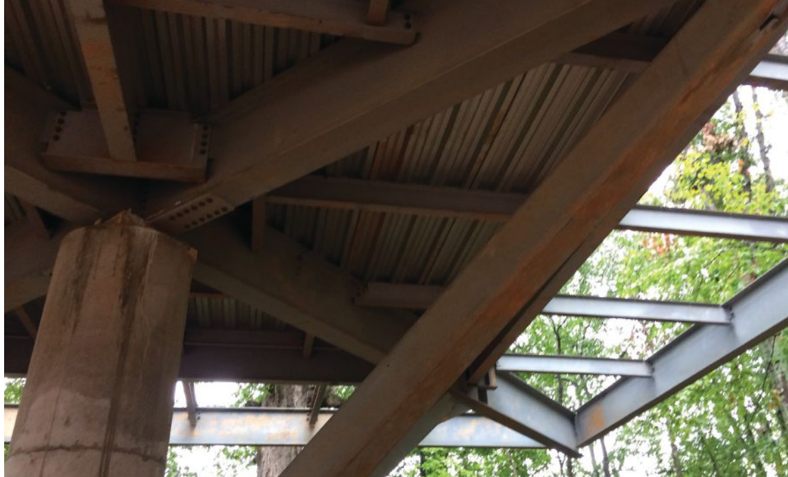
above: The support system for the treehouse is a single, central concrete column with steel braces that cantilever to the edges, allowing the forest floor below to remain exposed and undisturbed.
