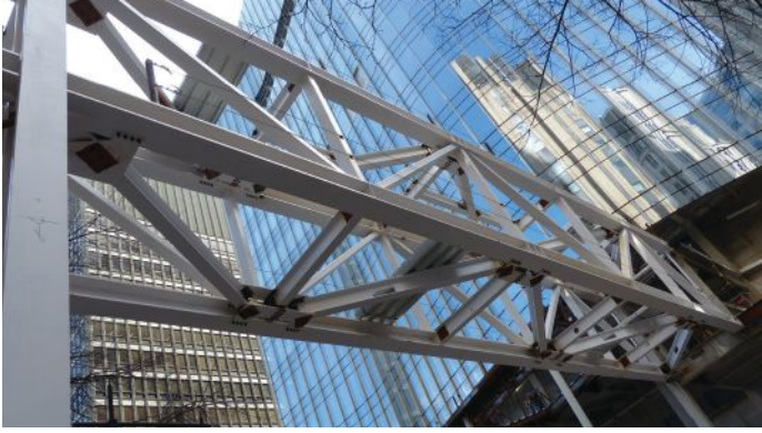
above: The long-span pedestrian bridge provides a direct connection from the new facility to an existing research building.
