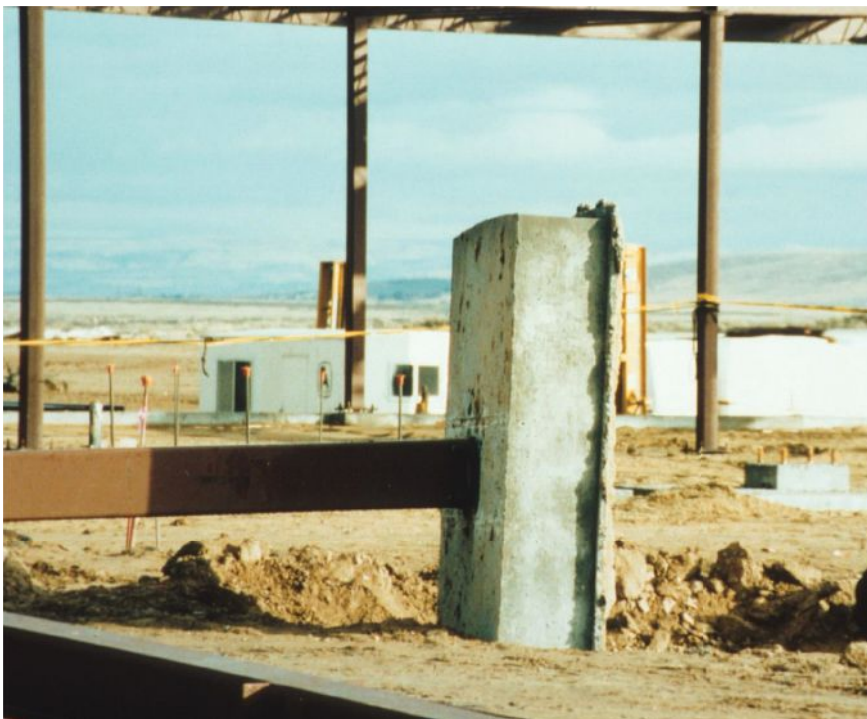
Fig. 1. An erection collapse due to the footing overturning and a lack of bracing.
