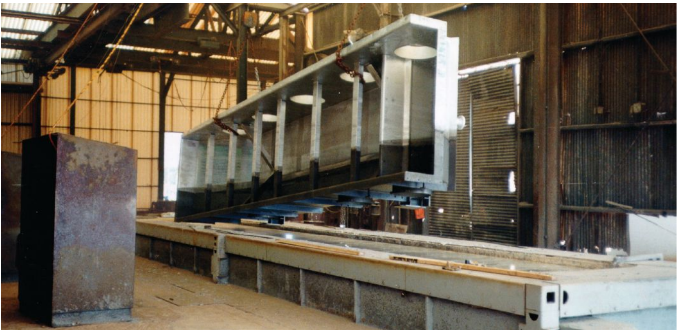
A large steel element going in for its second zinc dip.
