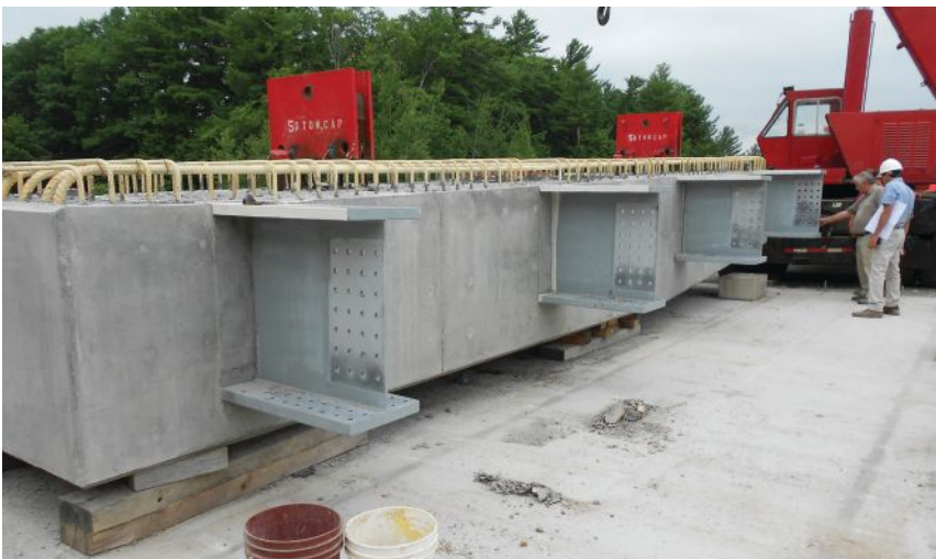
above: The full 103-ton steel superstructure.
