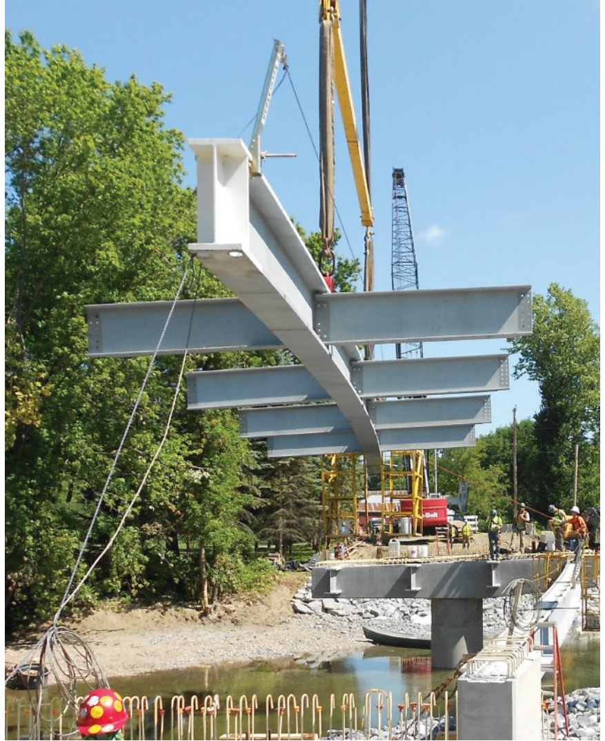
above: Erecting the steel superstructure.
