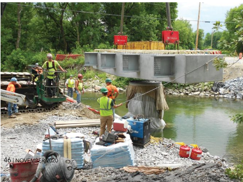
Placing the precast cap unit on the mono-shaft.
