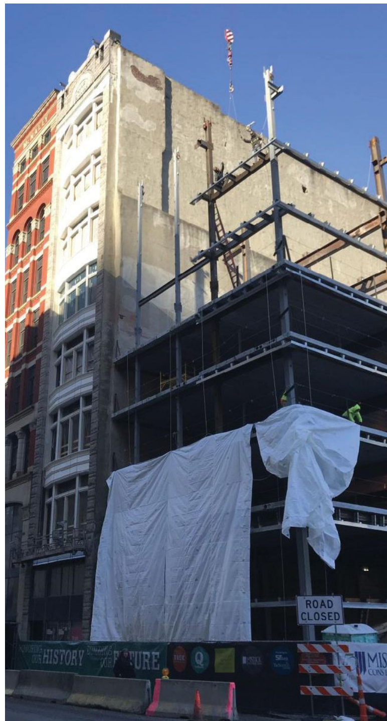
2. Erection of the 11-story addition.
