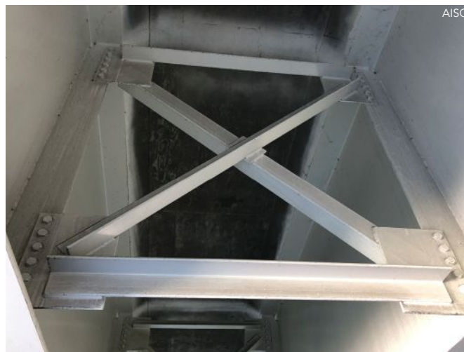
A welded member end connection (left) and an X-type cross-frame with welded member end connections (right).
