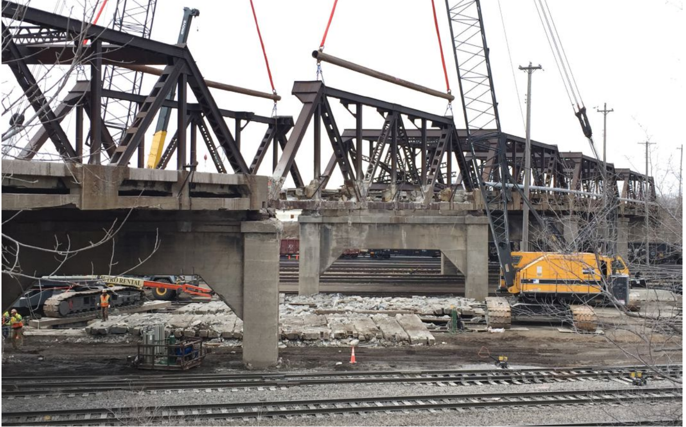
above: Removing the trusses from the original bridge, which had been used to cross the rail yard for nearly a century.
