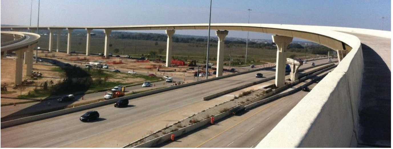
above: One of Texas' nearly 500 twin-tub girder bridges currently in service.
