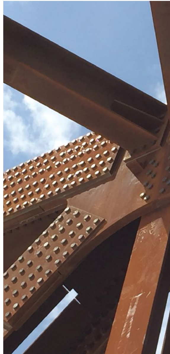
right: An upper chord node with split tension members and connections.
