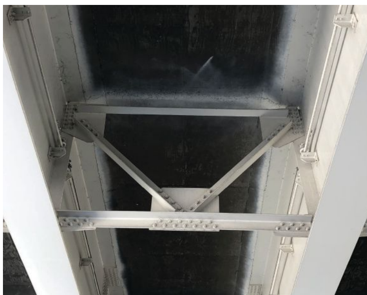
A K-type cross-frame with bolted end connections—not recommended unless absolutely necessary.
