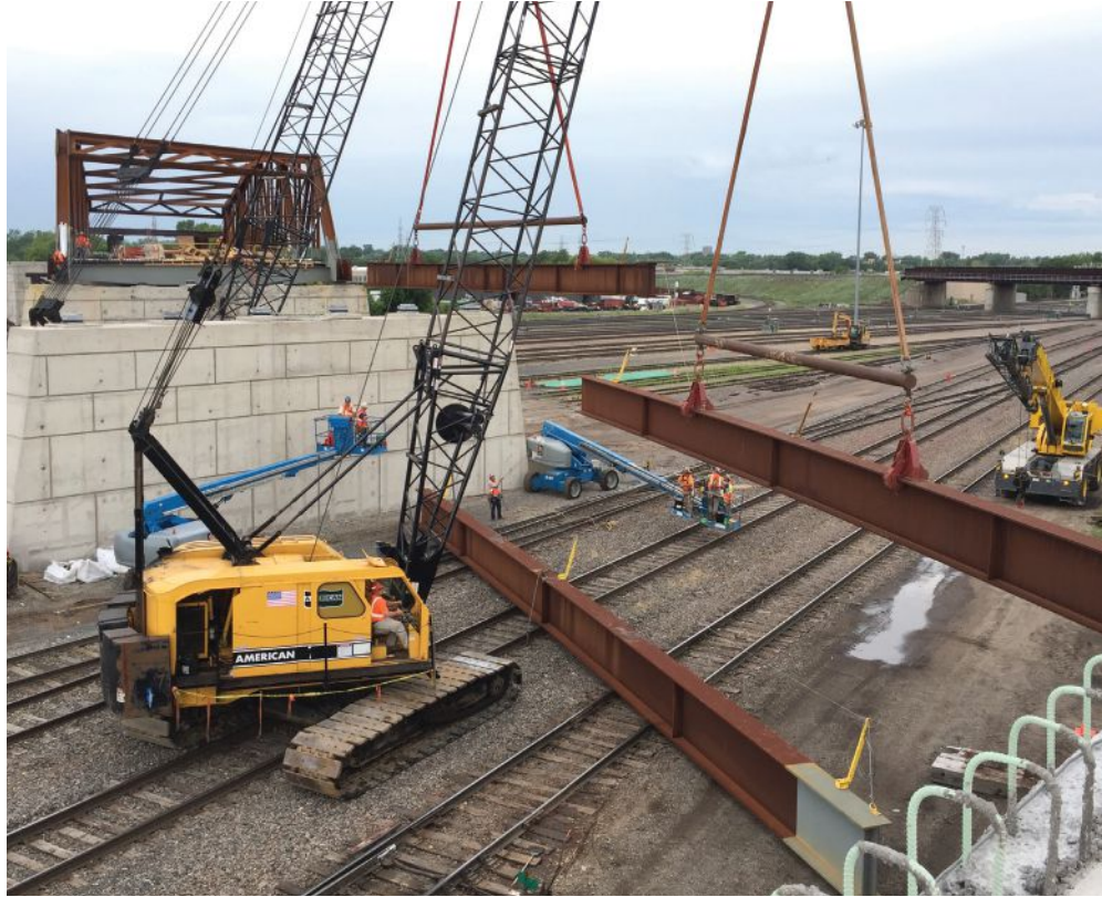
above: Erecting one of the two 127-ft-long approach spans, which are supported by conventional plate girders.
