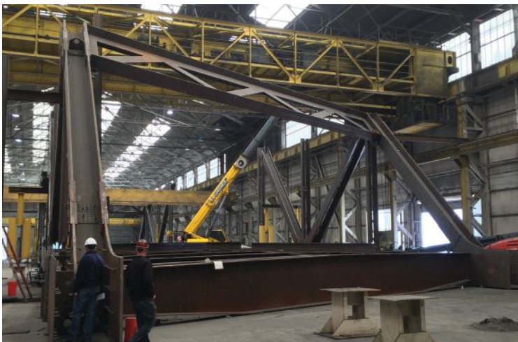
above and below: Fabricator Industrial Steel Construction, Inc. (ISC) first assembled the bridge trusses in its Gary, Ind., shop to ensure that everything fit together. The steel was then disassembled and trucked to the bridge site.
