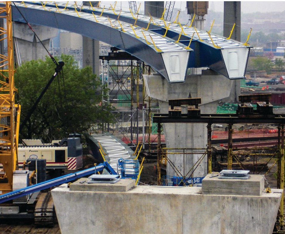
Milwaukee's Marquette Interchange twin-tub girder bridge project (to read about it, see "Steel Bridge News" in the March 2007 issue at www.modernsteel.com ).
