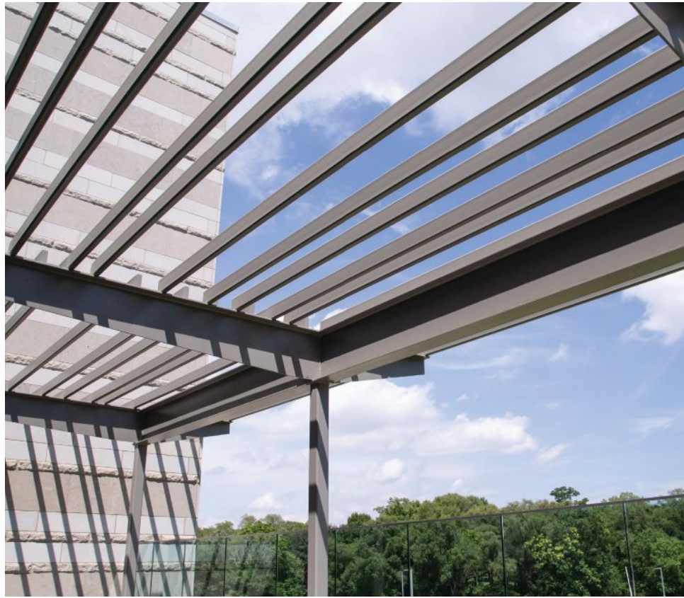
An exterior trellis adhering to AESS 1 (Basic Elements) requirements.
