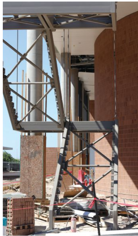
above: The exterior “spring” stair at the southeast corner of the building contains three intermediate landings that give the appearance of a coiled spring.
