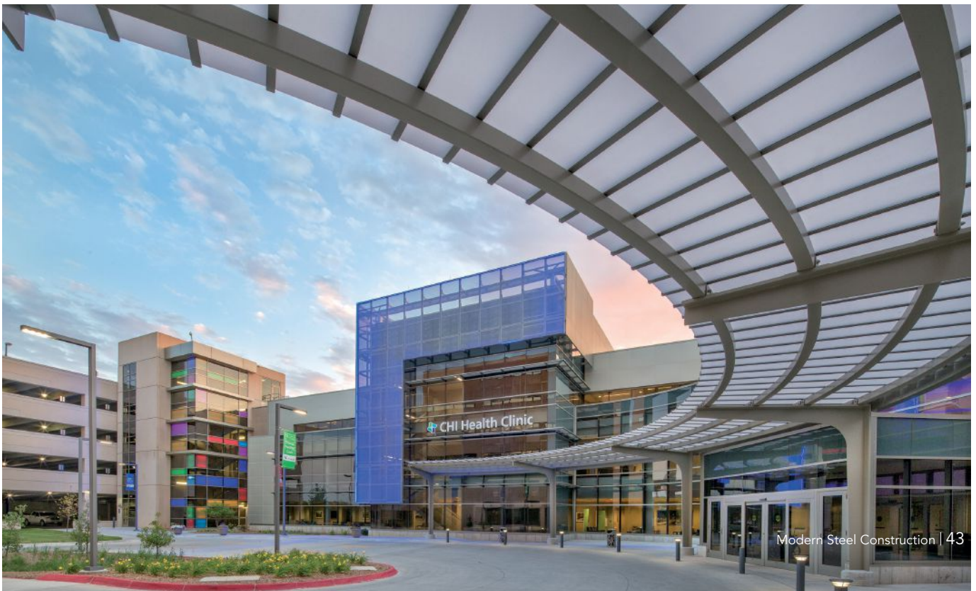
above/below: AESS using high-performance coatings in exterior applications.
