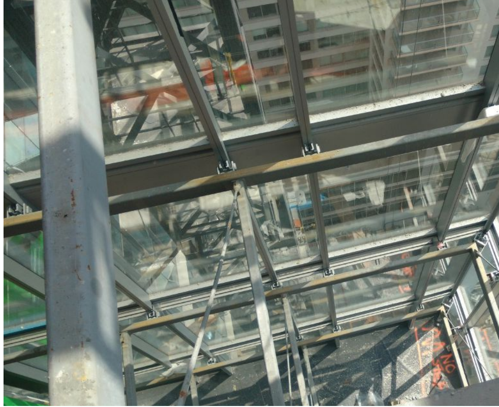
above: HSS elevator framing.
