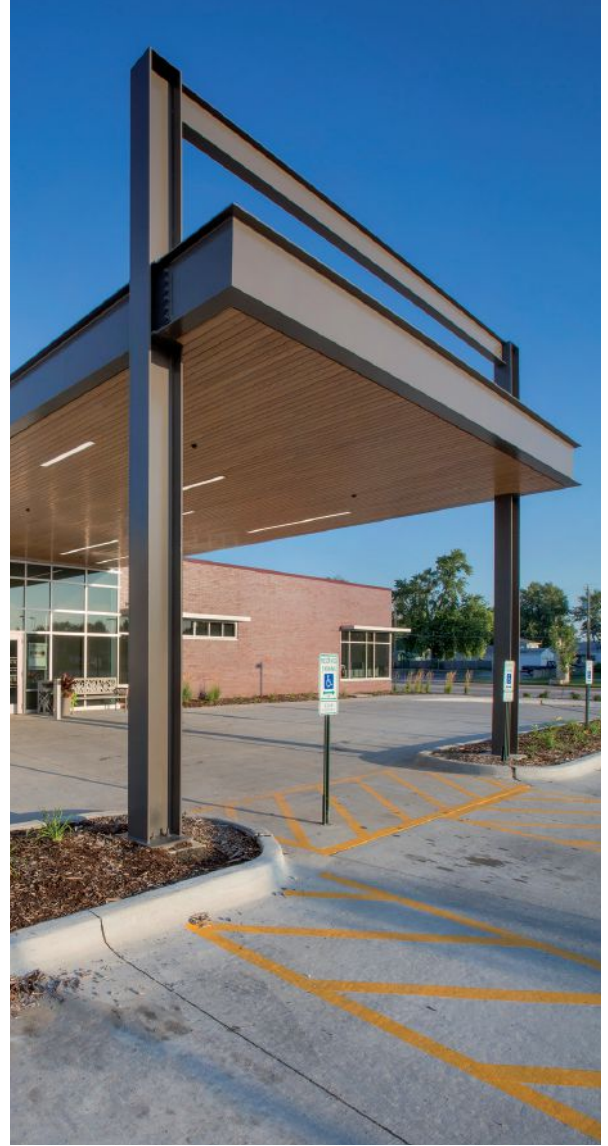
above/below: AESS using high-performance coatings in exterior applications.
