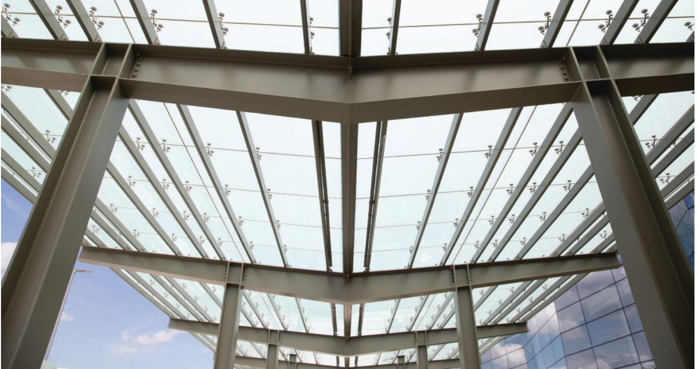
An exterior canopy structure framed with steel adhering to AESS 3 (Feature Elements in Close View) requirements.
