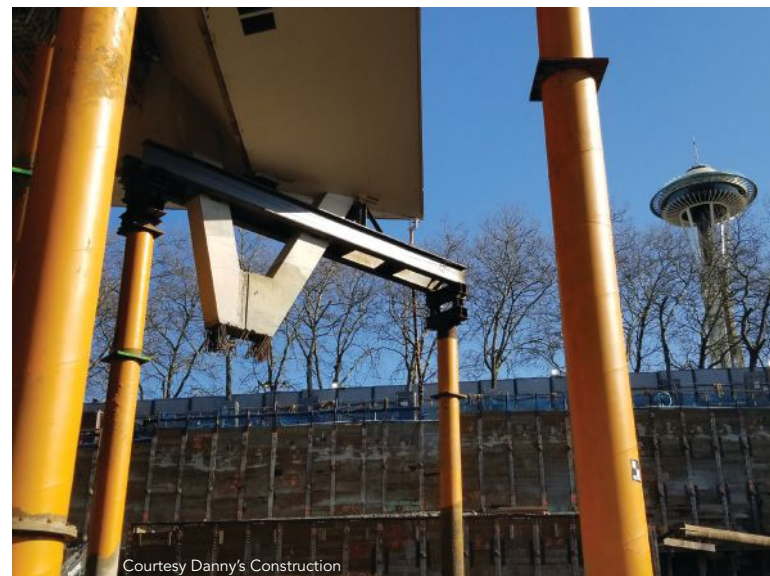
above and left: Temporary roof shoring and excavation. below: W36 beams supporting existing Y-columns.
