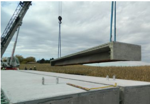
above: An FSPG bridge being installed in Nebraska.
