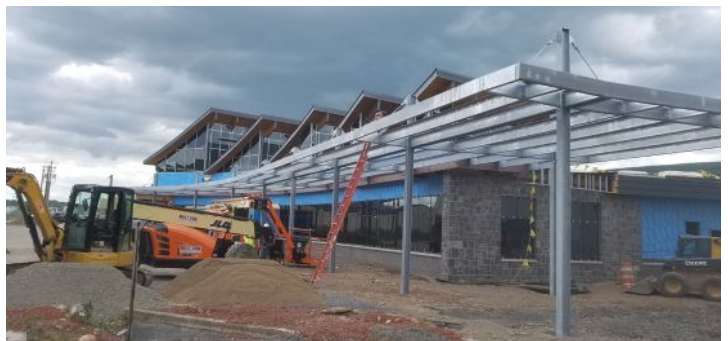
above: A new 40,000-sq.-ft passenger terminal building for the Williamsport (Pa.) Municipal Airport, a recent Standard Iron Works project.
