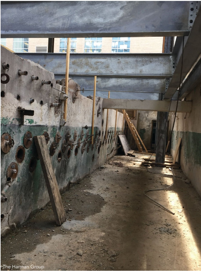
Drive aisle framing at the south end of the building. The existing tunnel walls and floor remained after demolition of the tunnel roof. New steel building columns were threaded through openings cut into the existing tunnel floor and extend to new foundations at the floor level below.
