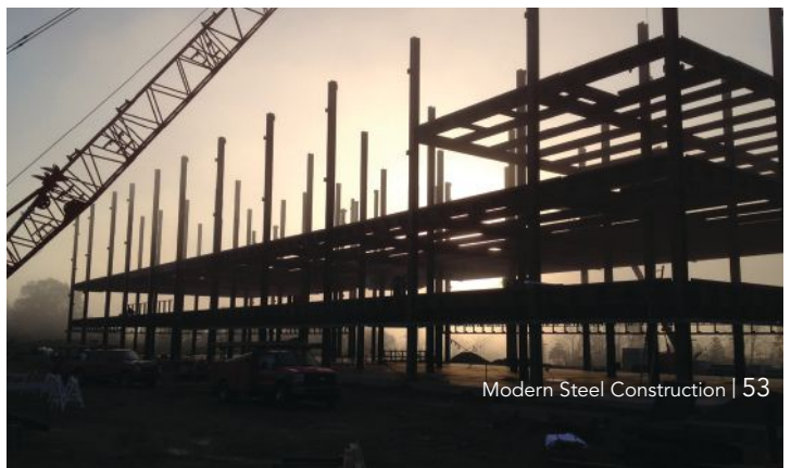
below: Another recent Standard project, a 100,000-sq.-ft Geisinger office building in Danville, Pa.
