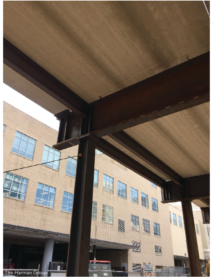
A typical transfer girder at the second floor.
