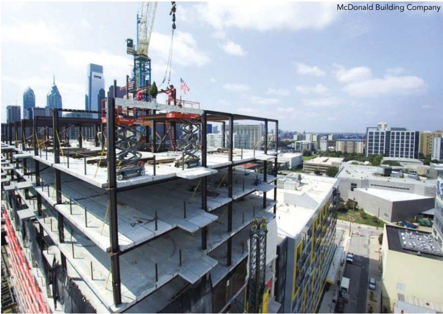
Placing of the final steel beam.
