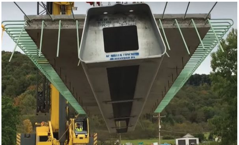
above: The first FSPG bridge installed in Pennsylvania employs a full-depth deck, integral abutment, and prefabricated railing.
