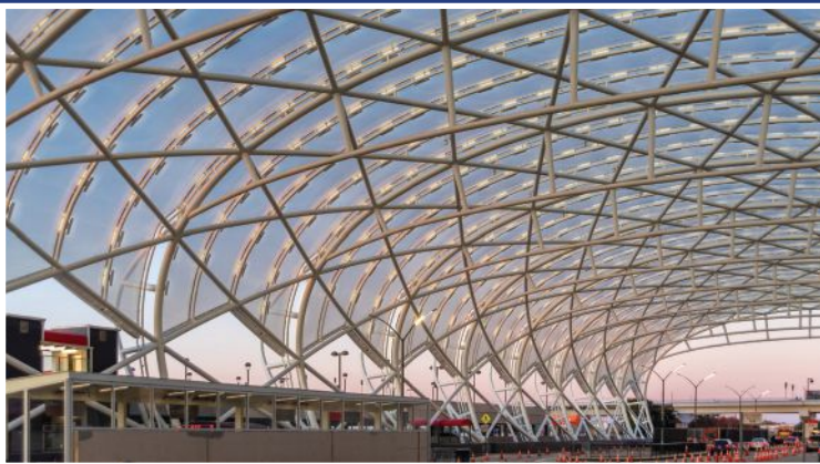
2020 IDEAS 2 National Winner - 920 pipe members rolled from 1300 tons of 14" pipe creating 38 super-trusses for the iconic canopy at Hartsfield-Jackson Atlanta Intl Airport. Atlanta, GA
