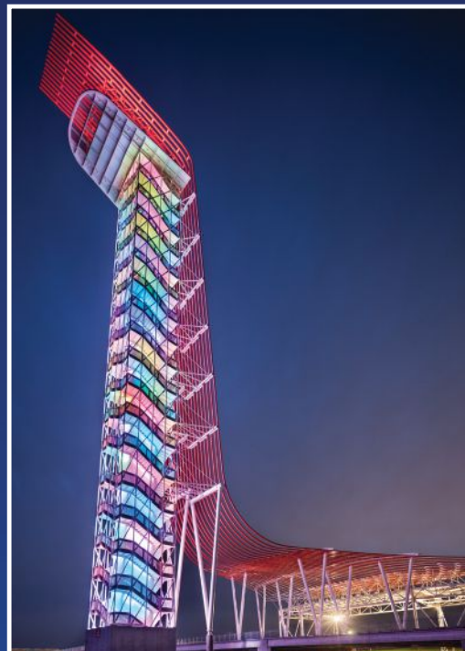
2015 IDEAS 2 Merit Award - 73 pieces of curved 8" sch 40 pipe totaling 35 tons for Circuit of the America Observation Tower. Austin, TX
