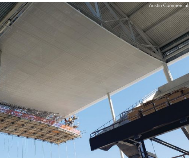
above: Installing a soffit on the underside of a portion of the roof canopy.
