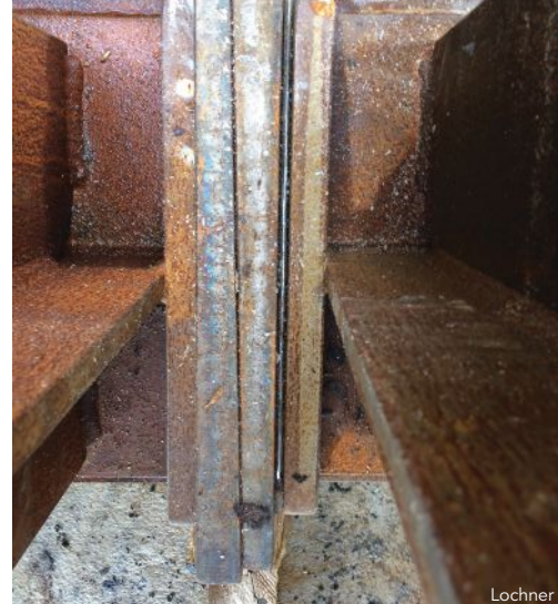
above: A plan view of the girder ends at the centerline of the pier, with wedges and shim plates placed for a SDCL detail, for the Potter School Road bridge.
