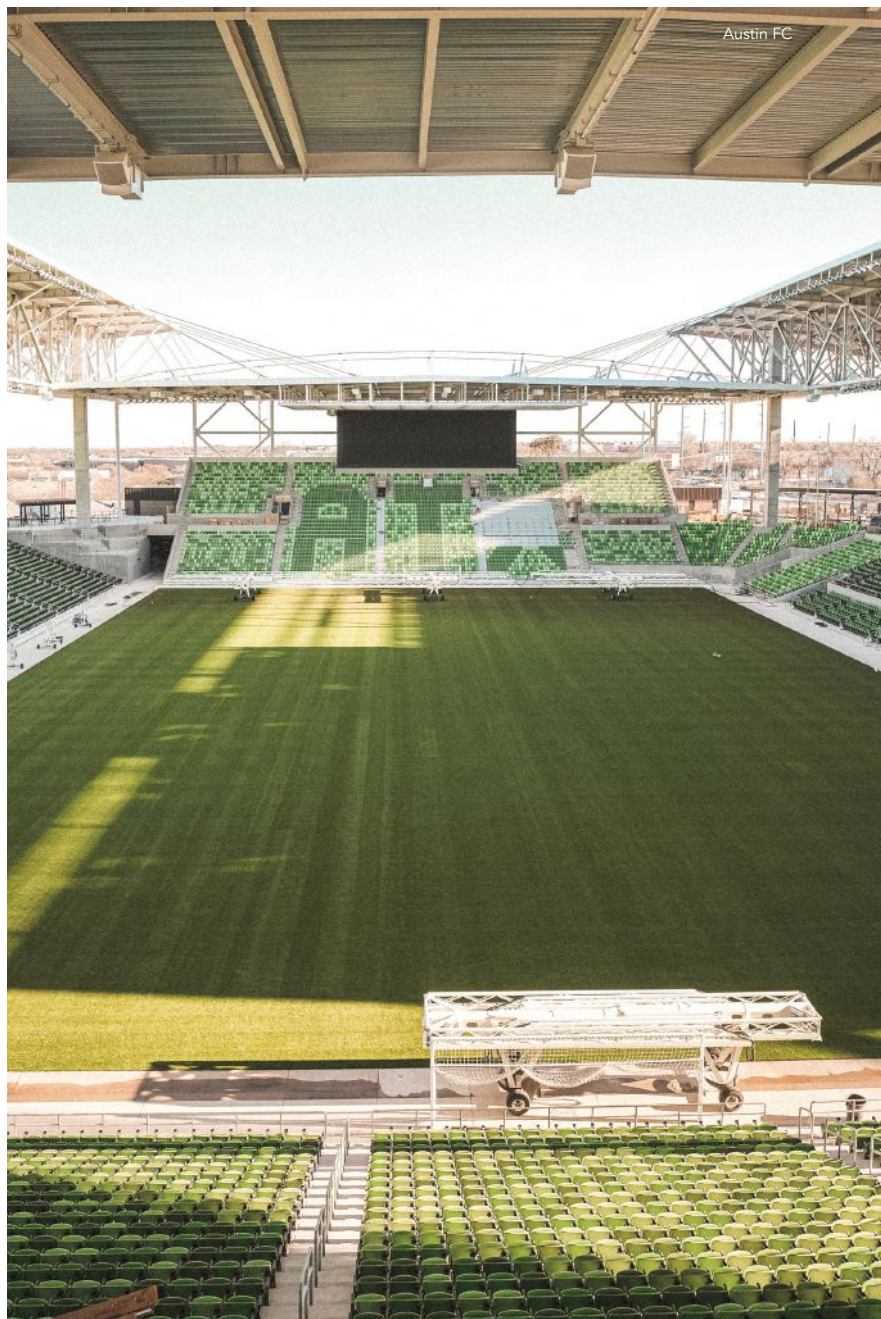
above and right: The cable-supported roof is held aloft by four 100-ft-tall columns.
