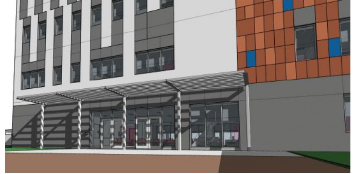
above and below: Along the front of each building, HSS posts support a 9-ft-wide pergola that parallels the courtyard walkways.
