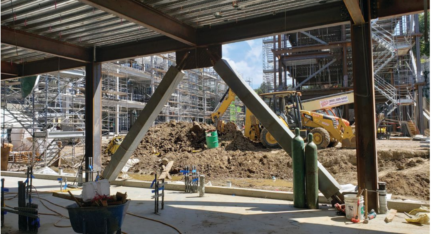
above and right: The buildings all incorporate buckling-restrained braces for the lateral force-resisting system.
