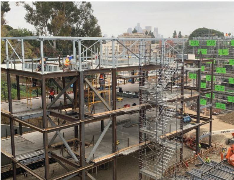
above and below: The village collectively uses 550 tons of steel framing.
