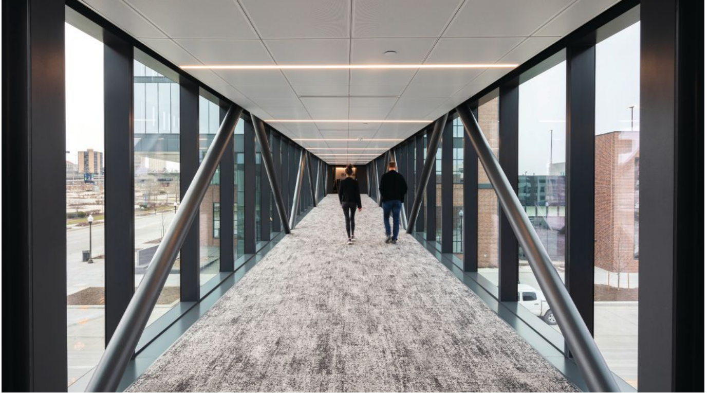
above: The steel-framed pedestrian skywalk between the headquarters building and the adjacent training facility spans 94 ft over a city street.
