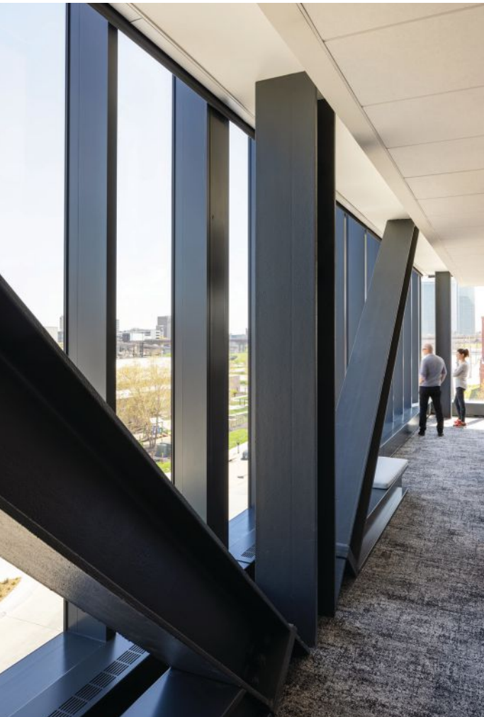
above and below: A section of one of the two-story V-shaped trusses during construction and following project completion.
