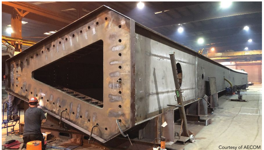
Courtesy of AECOM
