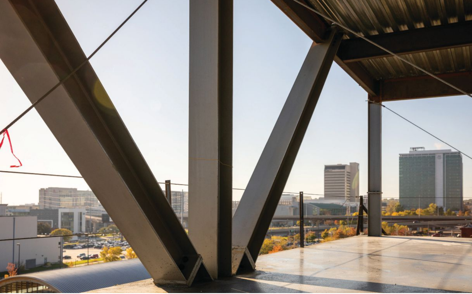
above and below: A section of one of the two-story V-shaped trusses during construction and following project completion.
