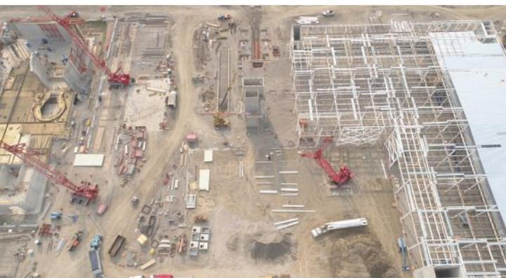
above and below: Ford presented significant redesign plans during steel fabrication, and Aristeo was able to quickly and efficiently revise its fabrication and erection sequences to allow for the changes to be made while maintaining the project schedule and limiting cost impacts.
