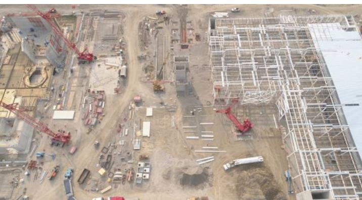
above and below: The majority of the more than 1,800 tons of structural steel was incorporated into the two-story battery lab building and attached support facility, one of the largest steel projects ever for steel fabricator Aristeo.
