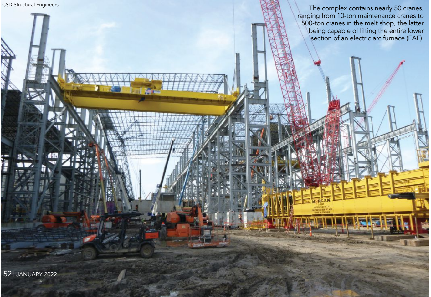
CSD Structural Engineers
