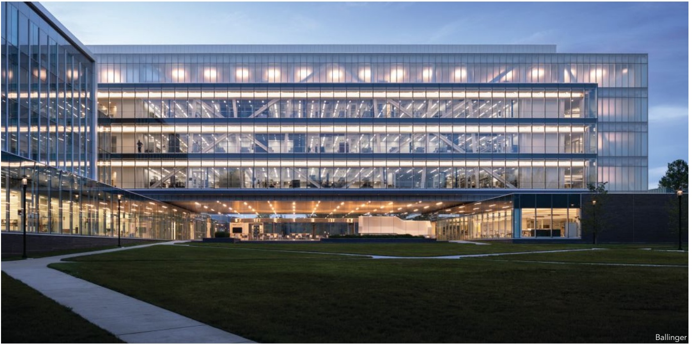
above and below: The central “bar” of the building is supported by three 260-ft-long by 55-ft-tall (four-story) exposed structural steel trusses, each with 160-ft center spans plus cantilevers at each end.
