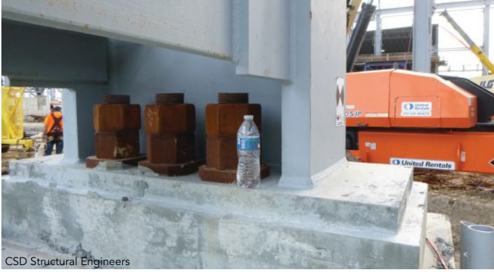
CSD Structural Engineers
