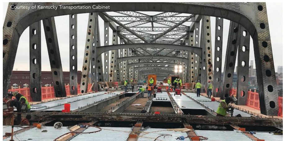
Crews work to repair the Brent Spence Bridge.
