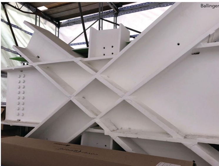
above and left: A node connection detail and an actual node. below: The project incorporates approximately 2,200 tons of structural steel.
