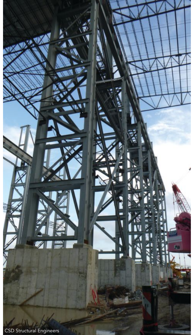
CSD Structural Engineers
