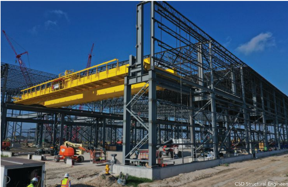
The entire mill is framed by more than 36,000 tons of structural steel.
