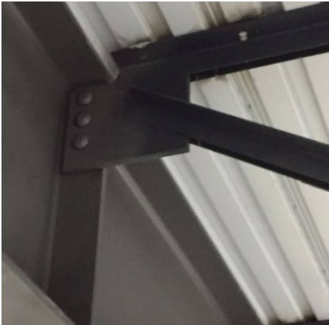
left: Fig. 2. This connection requires coordination of design aspects between the EOR and the open-web joist manufacturer's engineer.
