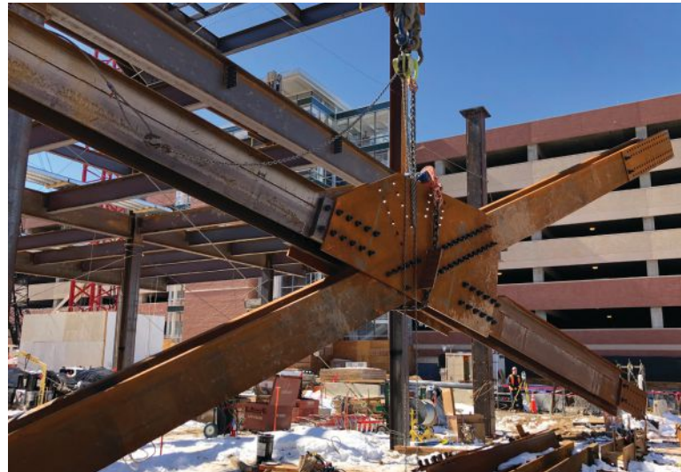
Steel for Tower 3 of the UHealth University of Colorado Hospital on the Anschutz Medical Campus in Aurora, Colo., topped out this past October, and the addition is expected to open this year. Bringing fabricator and detailer Puma Steel on board early in the project helped optimize connection design and keep things on schedule.
