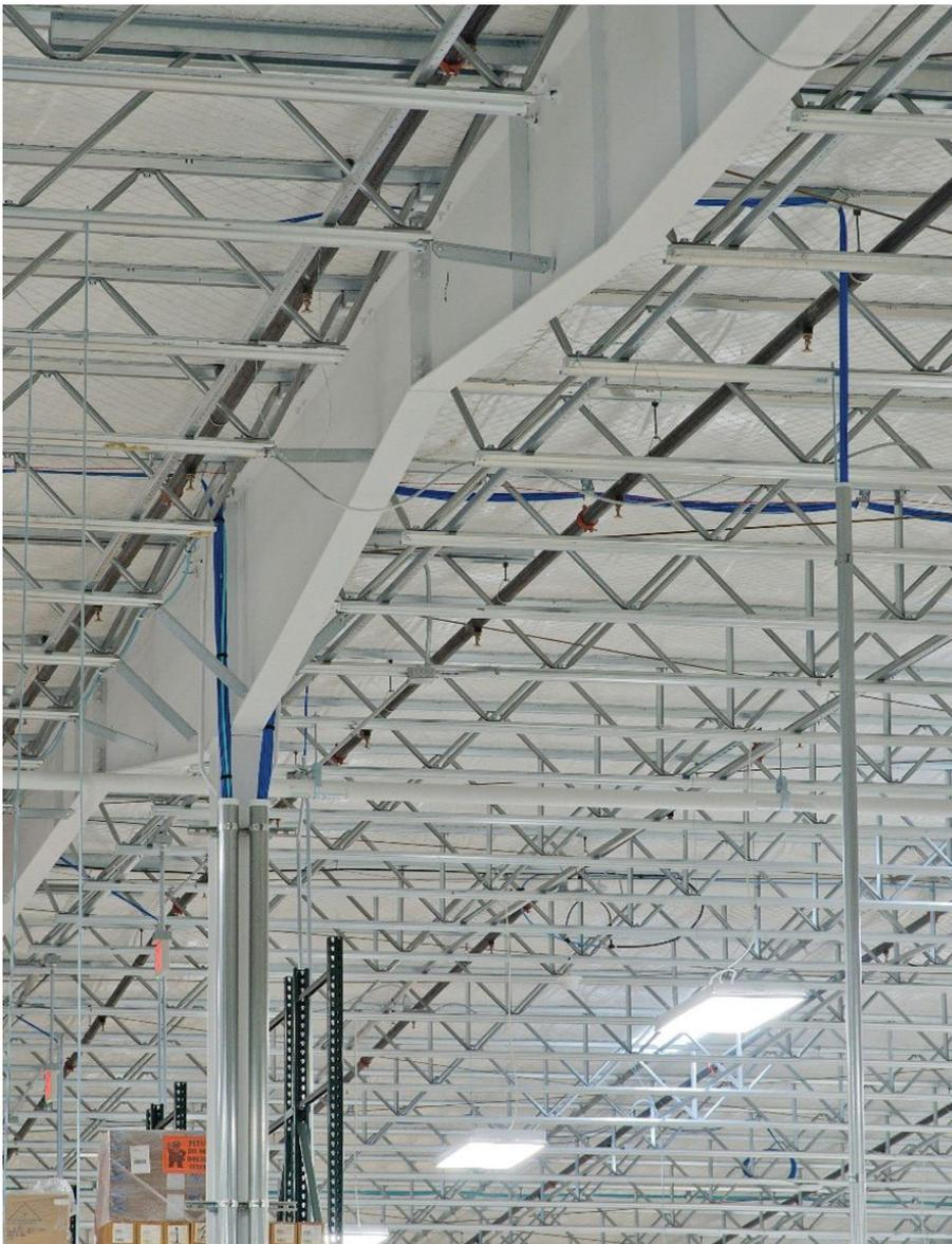
Interior column and roof girders of a modular frame.
