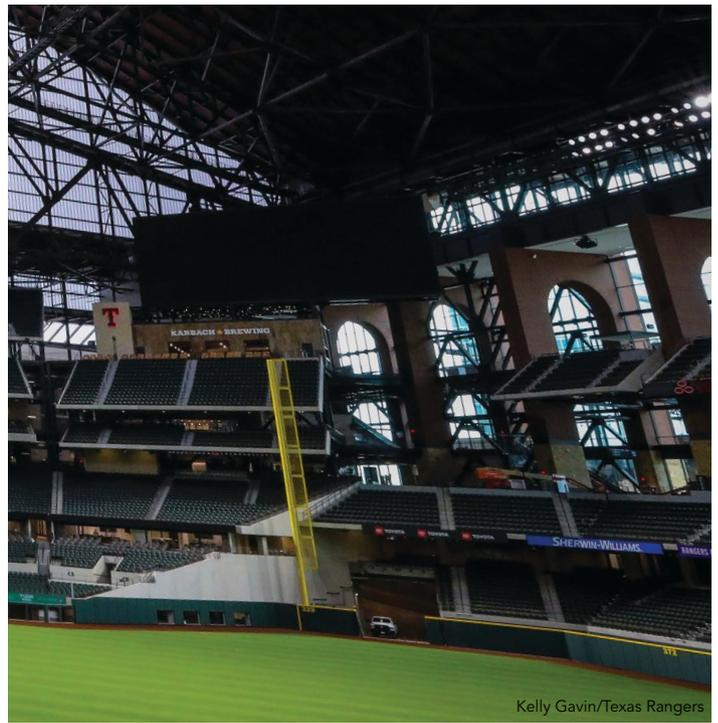
above and left: While much of the steel is left exposed, it also frames elements like the historic brick-clad arches, as shown in the photo above and REVIT model at left.
