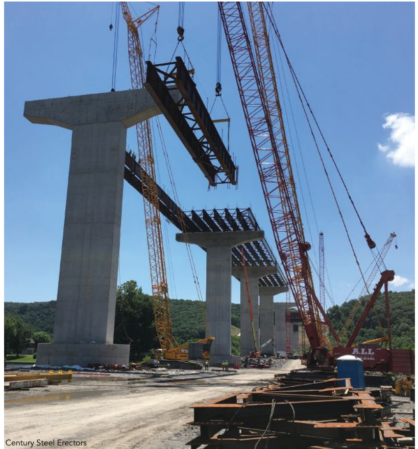
Century Steel Erectors
