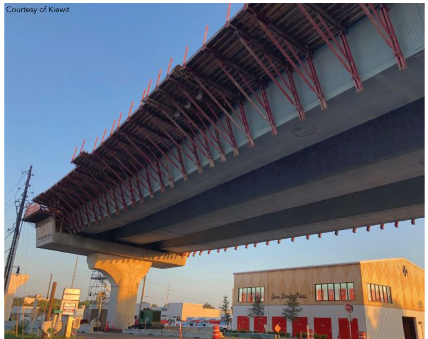
Lateral bracing and bottom flange stiffeners for Ramp D.
