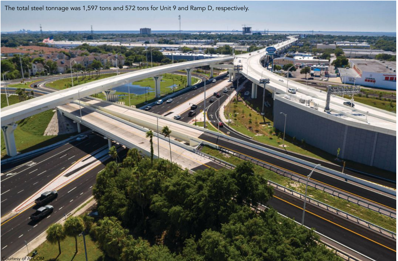
Courtesy of AECOM
