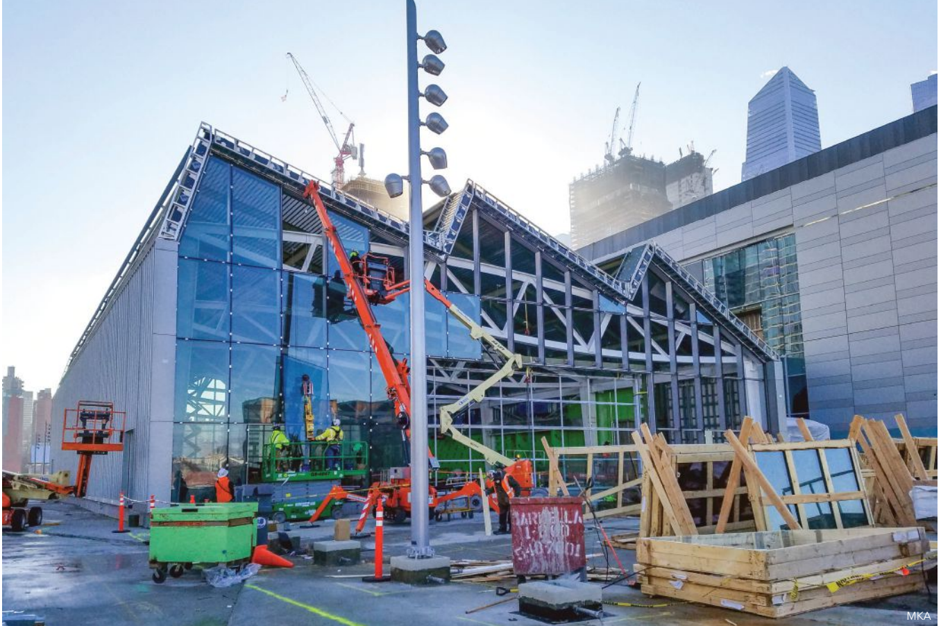
above: Steel framing for the rooftop pavilion.
