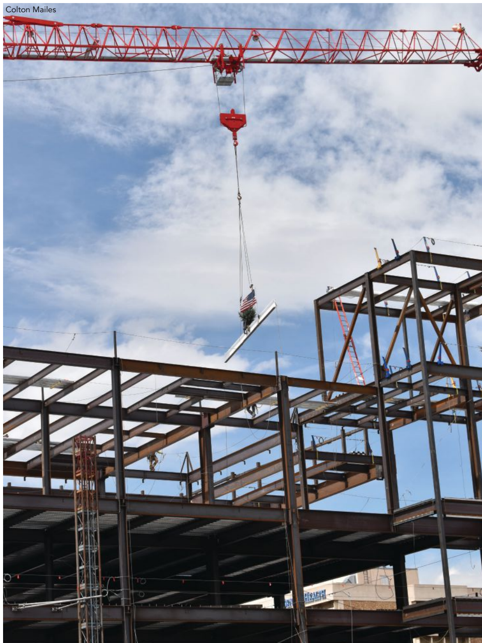
below: Topping out!
