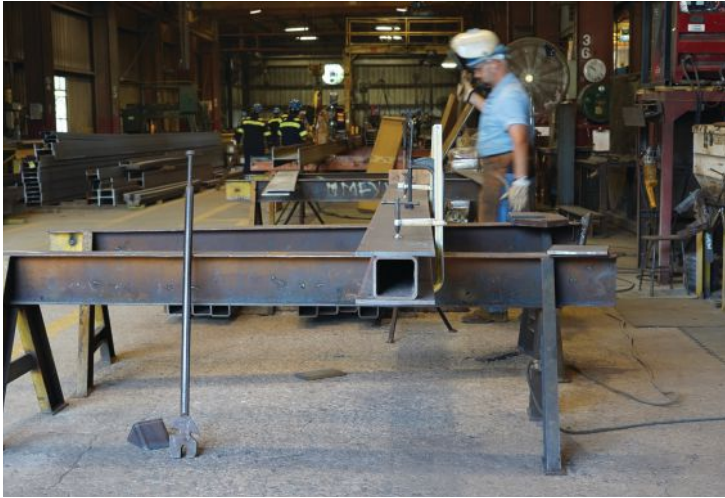
above: Custom truss chord fabrication.
