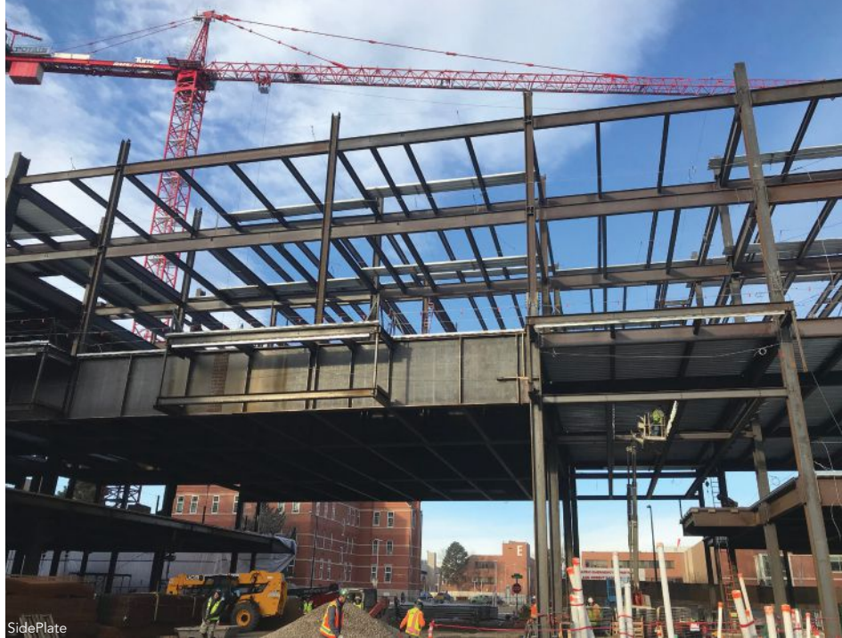
above: The project includes nearly 2,400 tons of structural steel in all.
