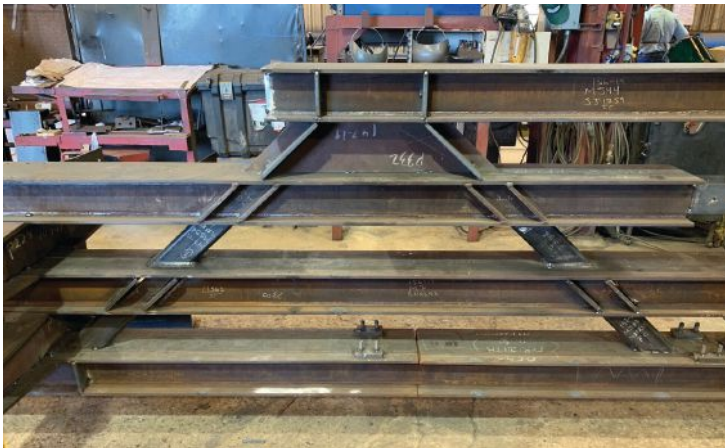
below: Fabricating a diagonal member with multiple overlapping truss members.
