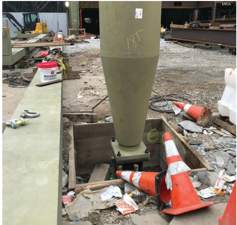
above and below: The two columns visible within the lobby space that support the halo beams above were designed to go above and beyond the call of duty. These 30-in.-diameter round HSS columns soar to heights of nearly 120 ft while simultaneously supporting the roof loads, eccentric façade loads, and wind loads. Custom tapered steel castings from Cast Connex were used at the top and bottom of each column.
