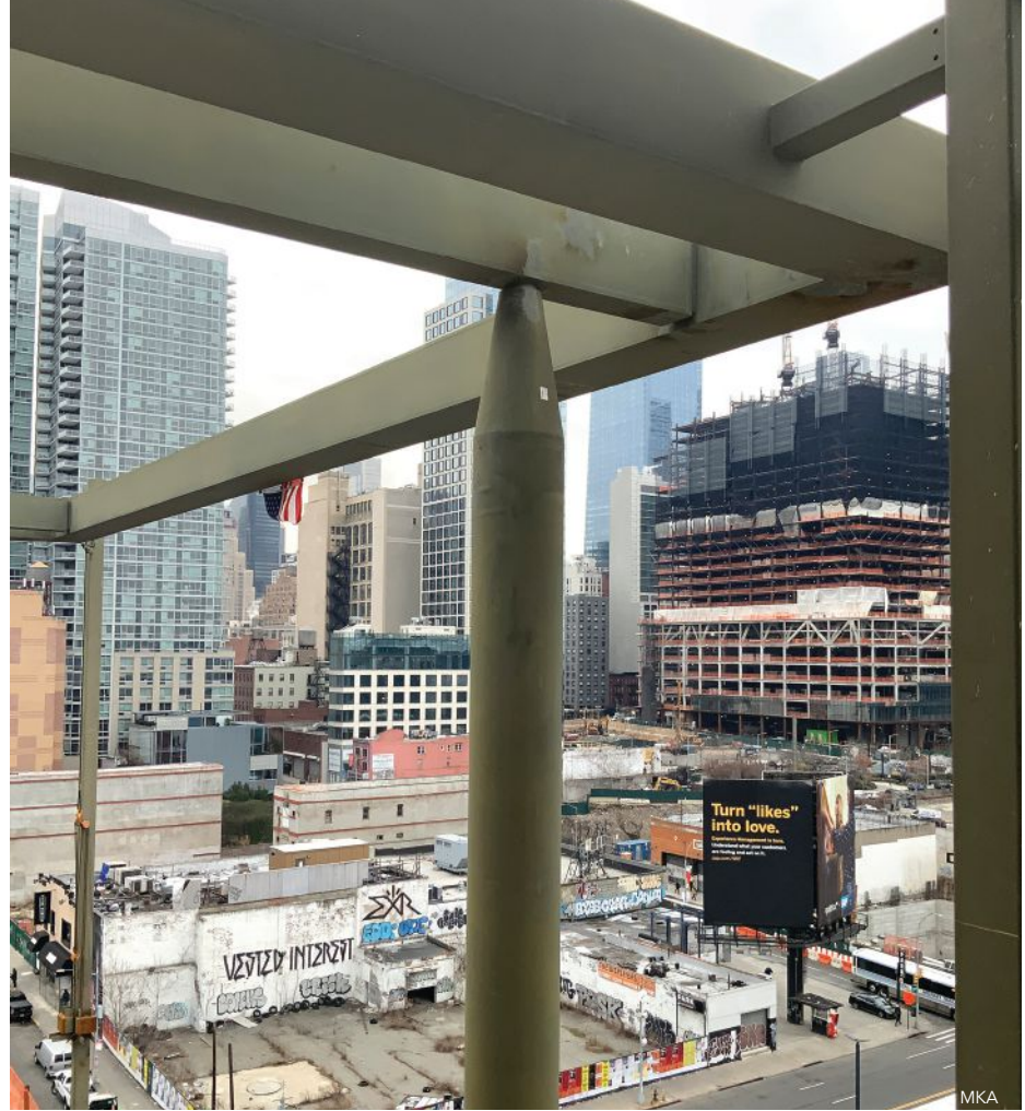
above and below: The two columns visible within the lobby space that support the halo beams above were designed to go above and beyond the call of duty. These 30-in.-diameter round HSS columns soar to heights of nearly 120 ft while simultaneously supporting the roof loads, eccentric façade loads, and wind loads. Custom tapered steel castings from Cast Connex were used at the top and bottom of each column.
