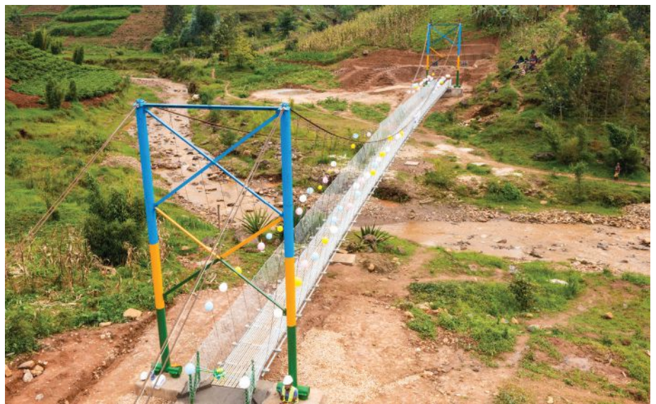
above: The completed Munini I Bridge just prior to inauguration, outfitted with balloons for the celebration with local community members.
