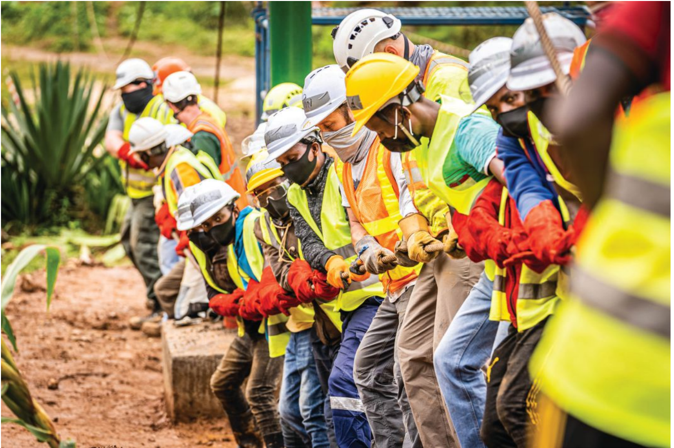
above: Local community members and the NSBA build team join hands to pull the heavy suspension cables into place.
