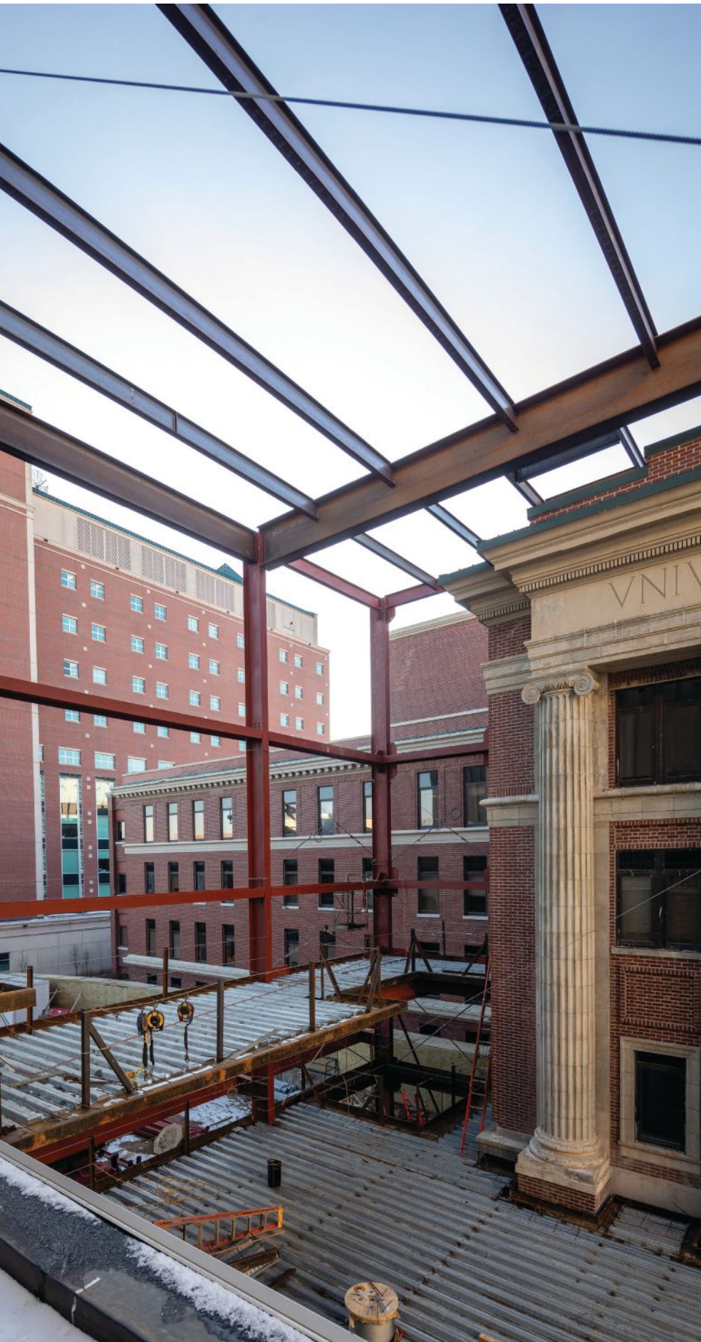
above and below: The tension-only X-bracing system became the preferred system for the design team.
