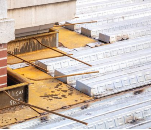
above and below: The team coordinated the slab conditions such that the transition between the existing and new floors of the two buildings fit together seamlessly.
