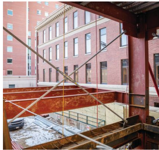
above and below: The tension-only X-bracing system became the preferred system for the design team.
