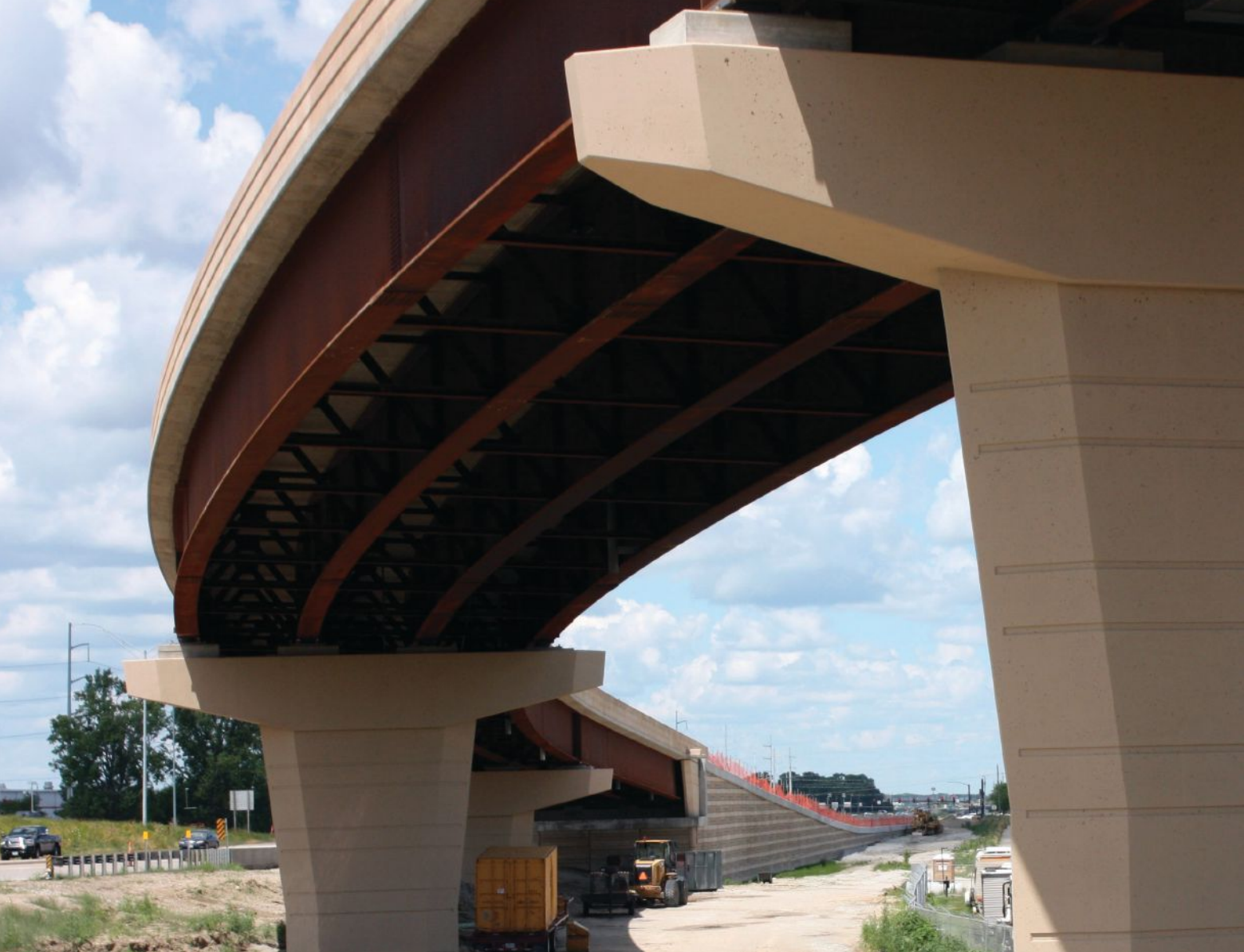
above: The project included developing aesthetic features to match other bridge projects in the corridor as well as using MSE walls to shorten the bridge as much as possible and limit right-of-way needs.
