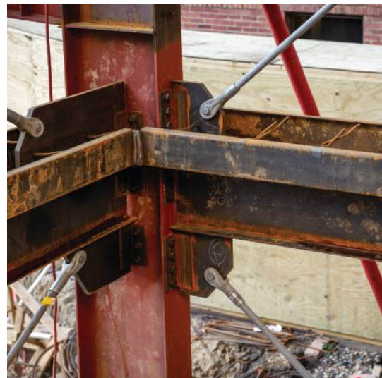
above and below: The tension-only X-bracing system became the preferred system for the design team.
