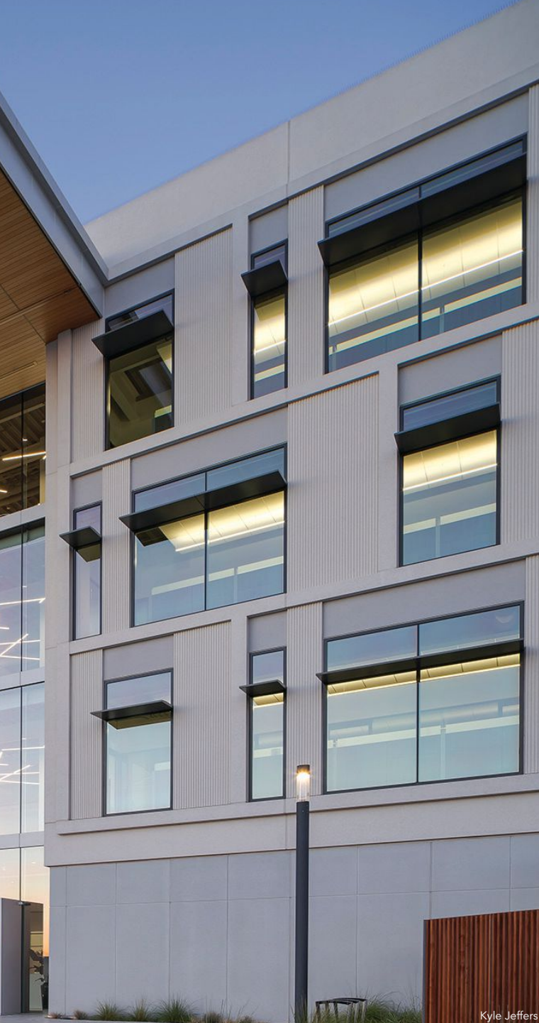
left: The new four-story structure at 1951 Harbor Bay Parkway serves as the headquarters for a growing oncology-focused life sciences company and sits on a rectangular footprint measuring 384 ft by 141 ft.
