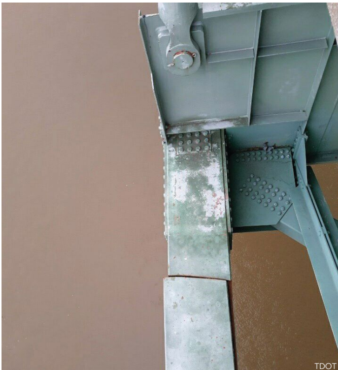
below: The cracked member discovered in the Hernando De Soto bridge in May 2021.
