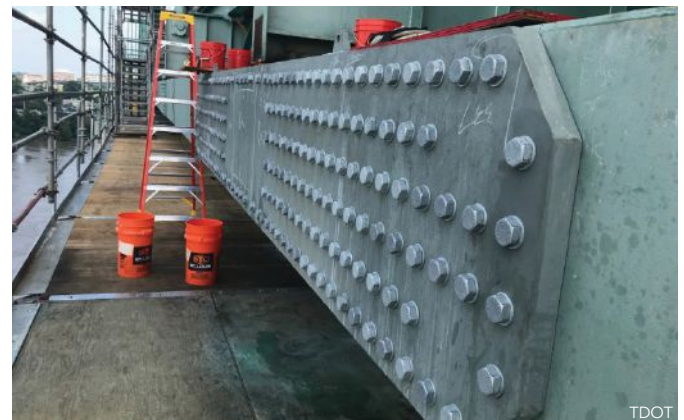
below: A newly installed plate after the last phase of the repair.
