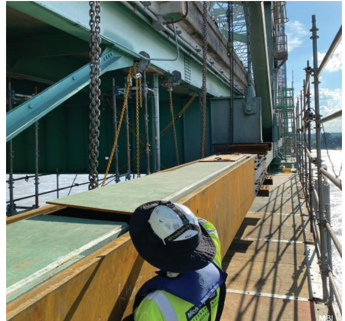
above: The temporary plate over the fractured member.
