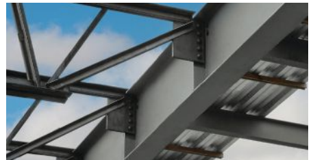
Joist reaction point occurs at beam centerline
