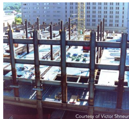
Fig. 2. Photograph of a frame with end-plate moment connections for the Mayo Clinic in Rochester, Minn.
