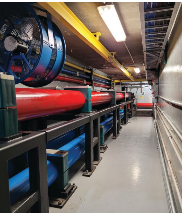
left: A look inside the tunnel under the hydraulic power building, following the high pressure (large red pipes) and return pipes (large blue pipes) from the hydraulic power building to the shake table. The bracing system and anchorage for the main pressure pipes (required to mitigate vibrations and excess stress on piping connections) are shown.
