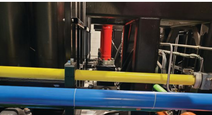
below and right: The view when standing at the base of the accumulation system looking in between the bottles. These photos show the congestion and complexity of the piping required for this system. The large (12-in. diameter) blue pipes return low pressure hydraulic fluid from the actuators back to the surge tank.
