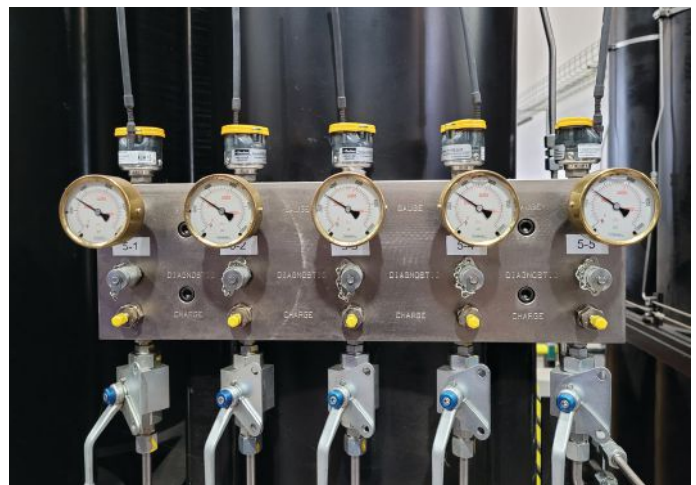
below: Manifold for one bank (of 15) of the accumulation system showing the analog and wireless pressure sensors of each bottle.
