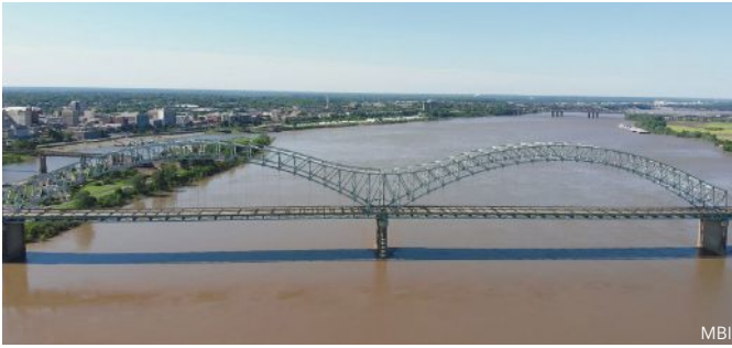
above: The repaired Hernando De Soto bridge.
