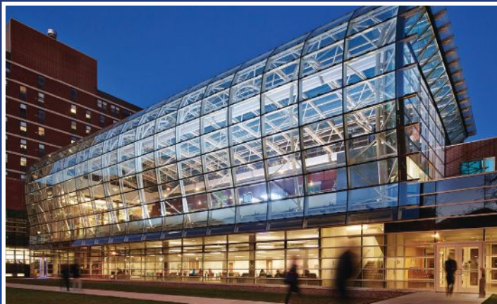
2014 SEAIO Best Project - Elliptically curved trusses rolled from 5" and 8" diameter AESS pipe for Institute of Environmental Sustainability at Loyola University. Chicago, IL
