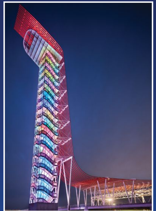
2015 IDEAS 2 Merit Award - 73 pieces of curved 8" sch 40 pipe totaling 35 tons for Circuit of the America Observation Tower. Austin, TX
