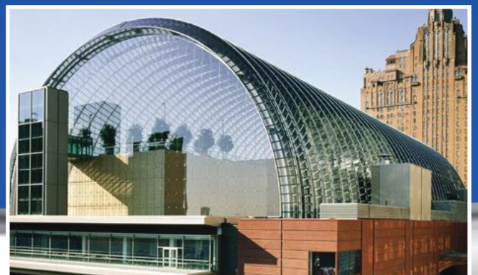
2003 IDEAS 2 National Winner - 300 tons of 5" square tubing curved 45° off-axis for the Kimmel Center. Philadelphia, PA
