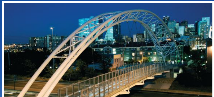
2007 NSBA Special Purpose Prize Bridge Award - 152 tons of 18" pipe curved in our Kansas City plant for the Highland Bridge. Denver, CO
