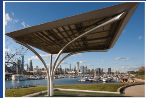
2013 IDEAS 2 Merit Award - 3600 pounds of pipe each curved with multiple radii for a solar canopy to recharge batteries on electrical vehicles. Chicago, IL
