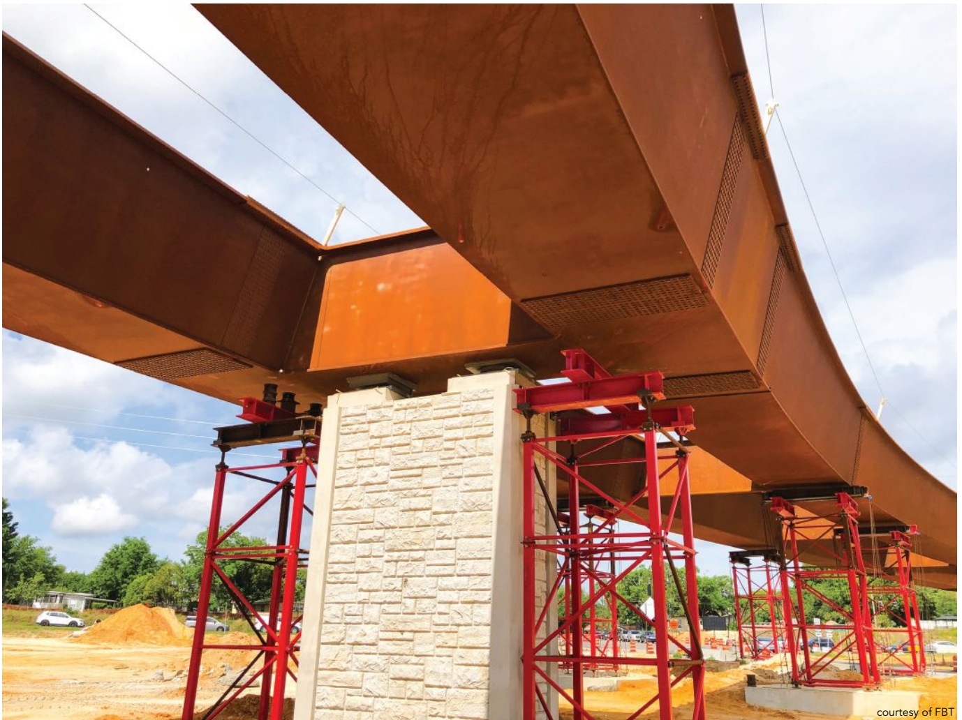
above: A typical pier segment supported by a single concrete column.
