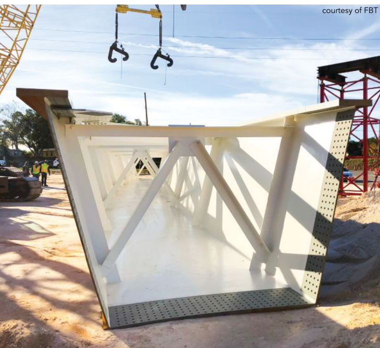
The white interior coating provides improved inspectability.
