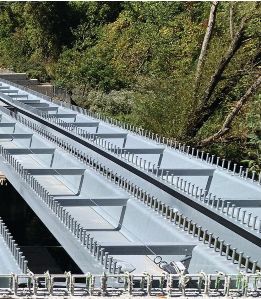
Crews setting formwork in place.
