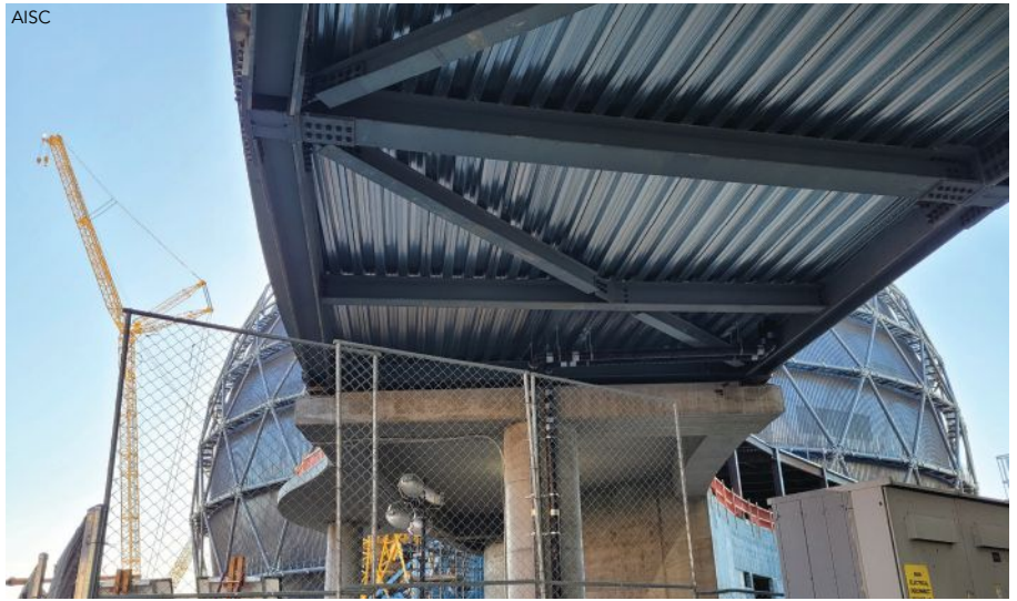
above: A steel-framed pedestrian bridge connects the Sphere to the Sands Convention Center.
