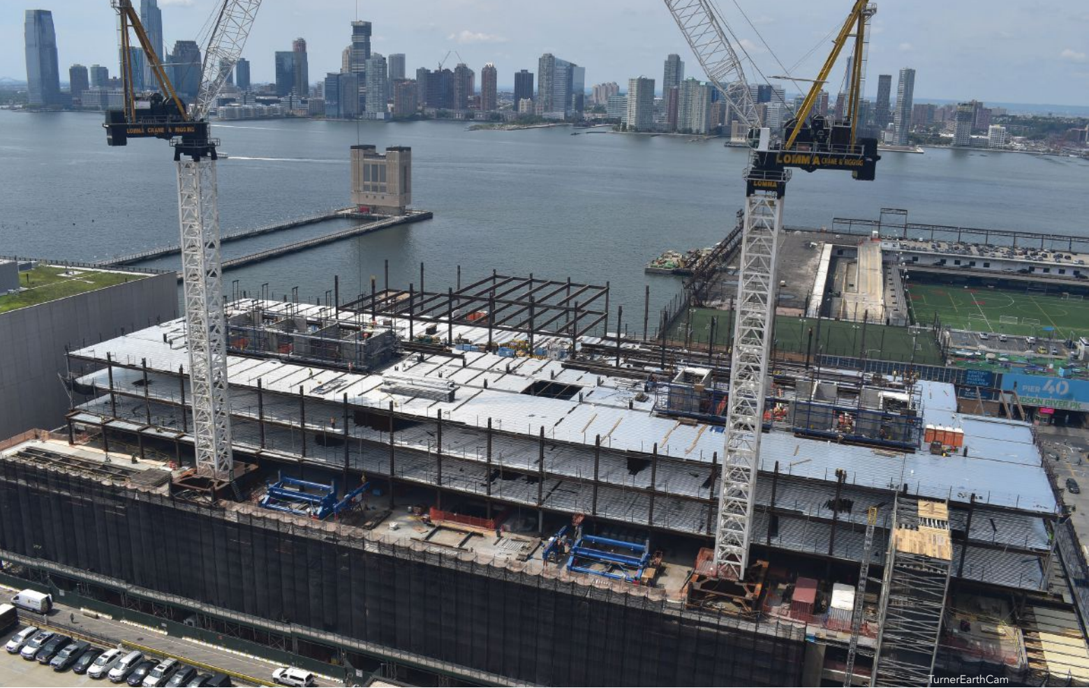
above and below: New steel framing being erected above the existing building.
