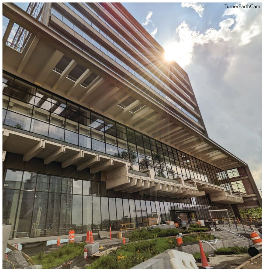
New building framing was erected at the same time existing steel was being reinforced.
