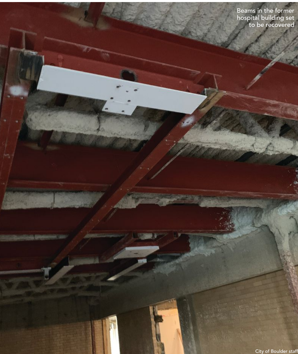
Beams set for reuse in Fire Station 3.
