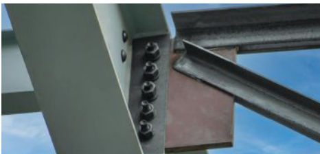
Flush-frame connection designed for efficiency
