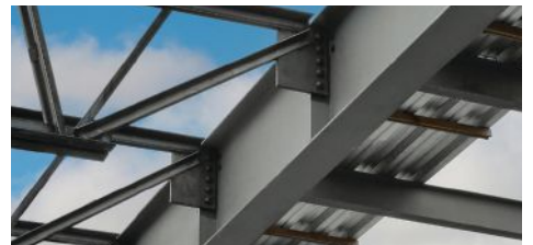
Joist reaction point occurs at beam centerline
