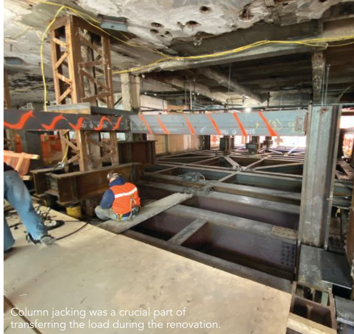
Second-floor framing was removed to create a double-height lobby.
