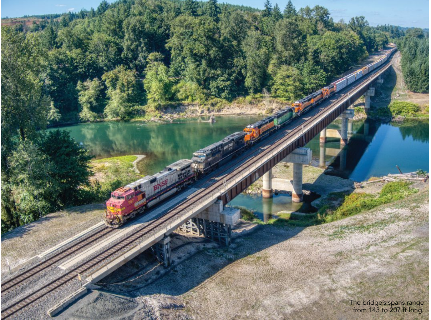
The spans are supported on large-diameter drilled shafts with rock sockets and box beam approach spans supported on H-piles.
