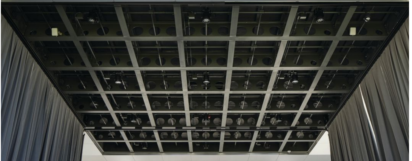
Perforated beams reduce the roof weight.
