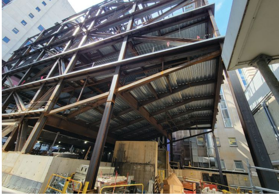
above: Temporary columns supported the 50-ft cantilever during steel erection.
