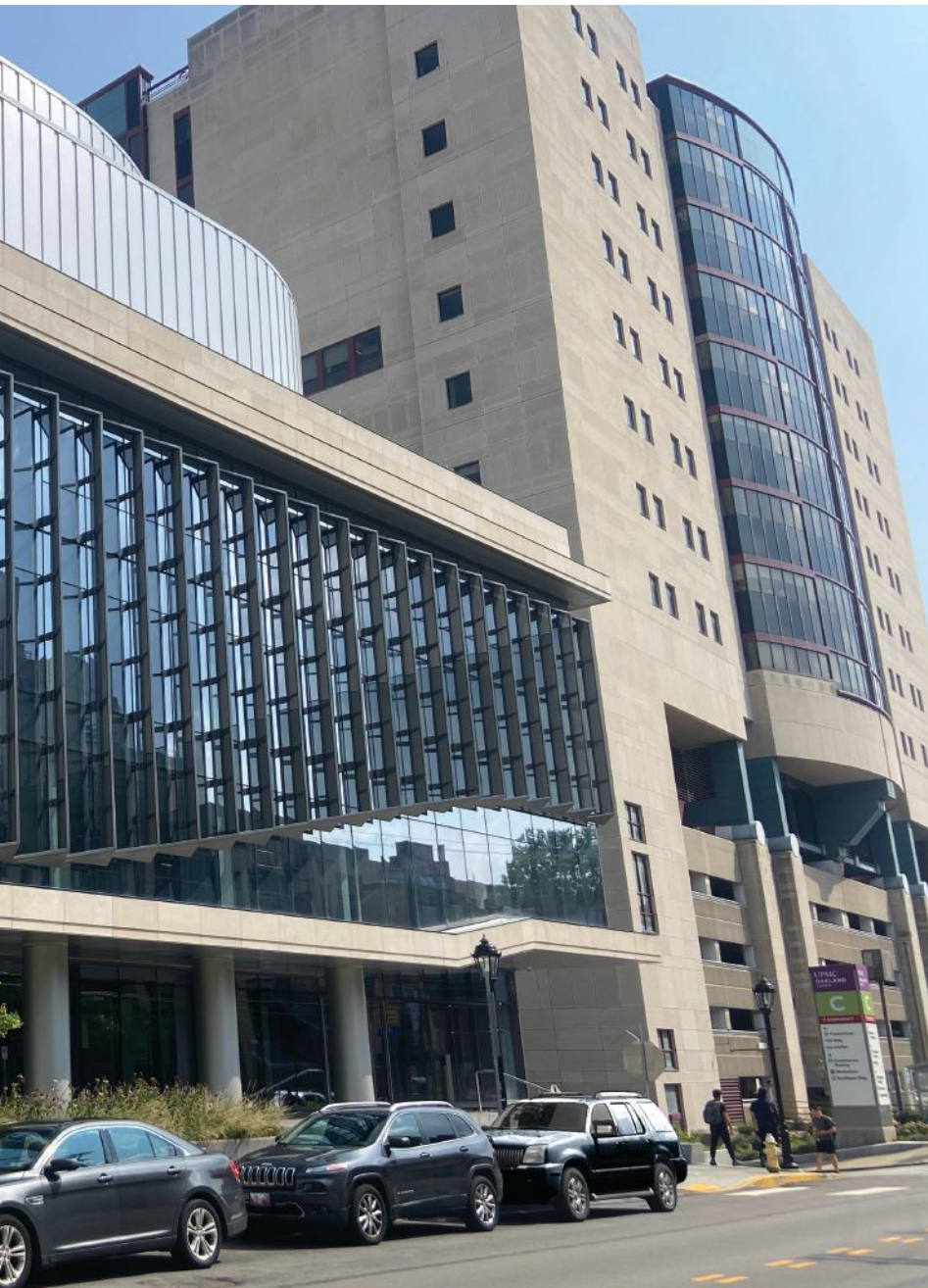
The cantilever extends over the adjacent hospital's generator vault and loading dock.
