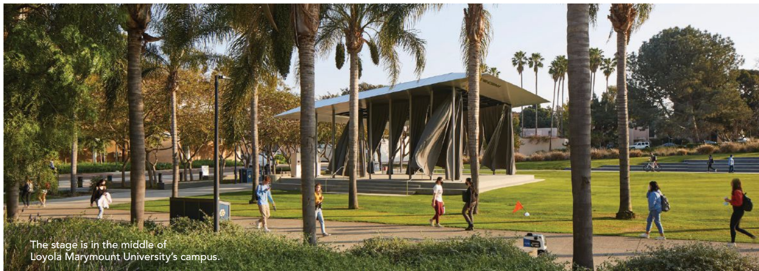
The roof has 10-ft typical cantilevers and a 12½-ft corner cantilever.
