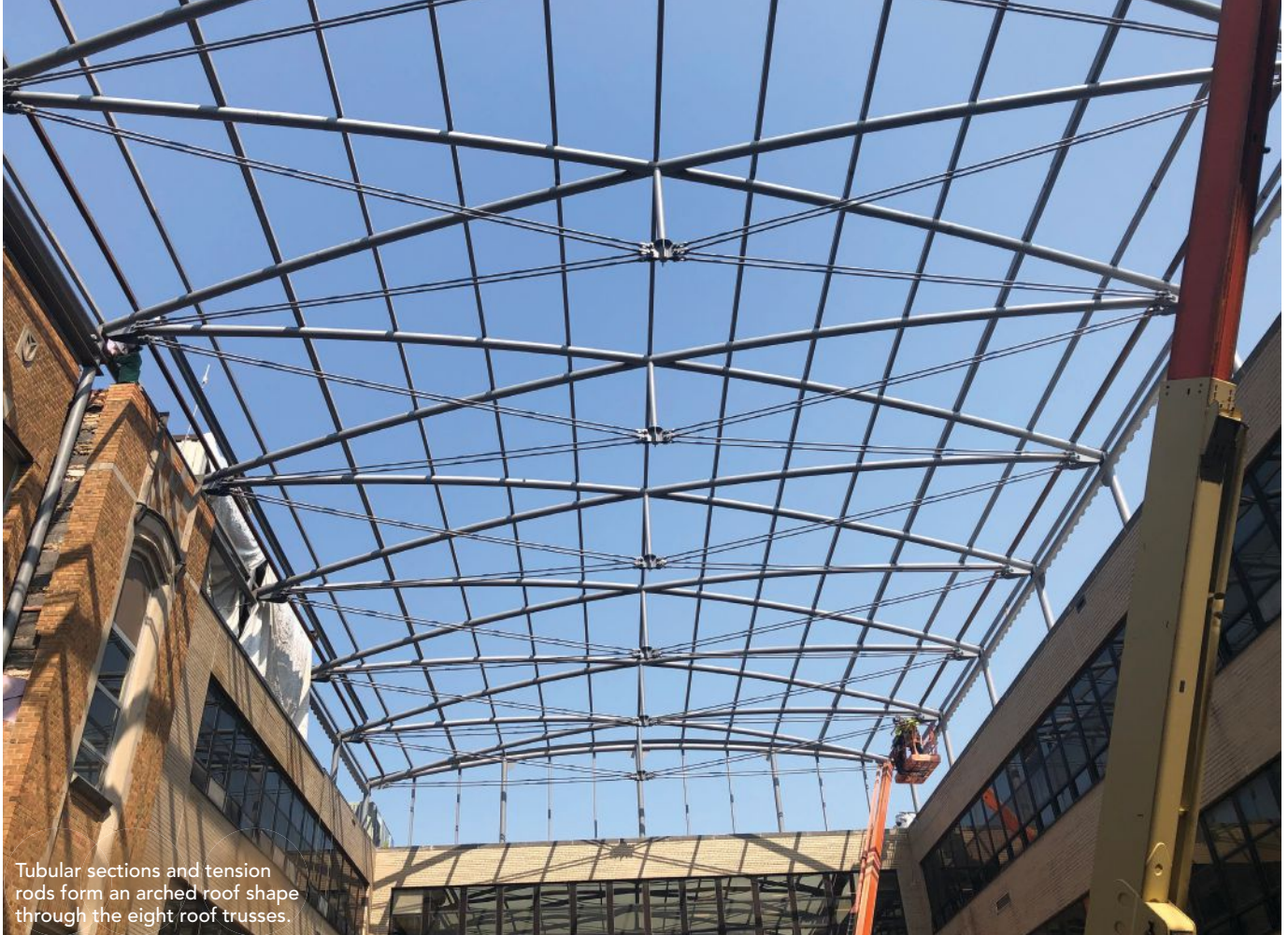
The trusses are specified to AESS Category 2.
