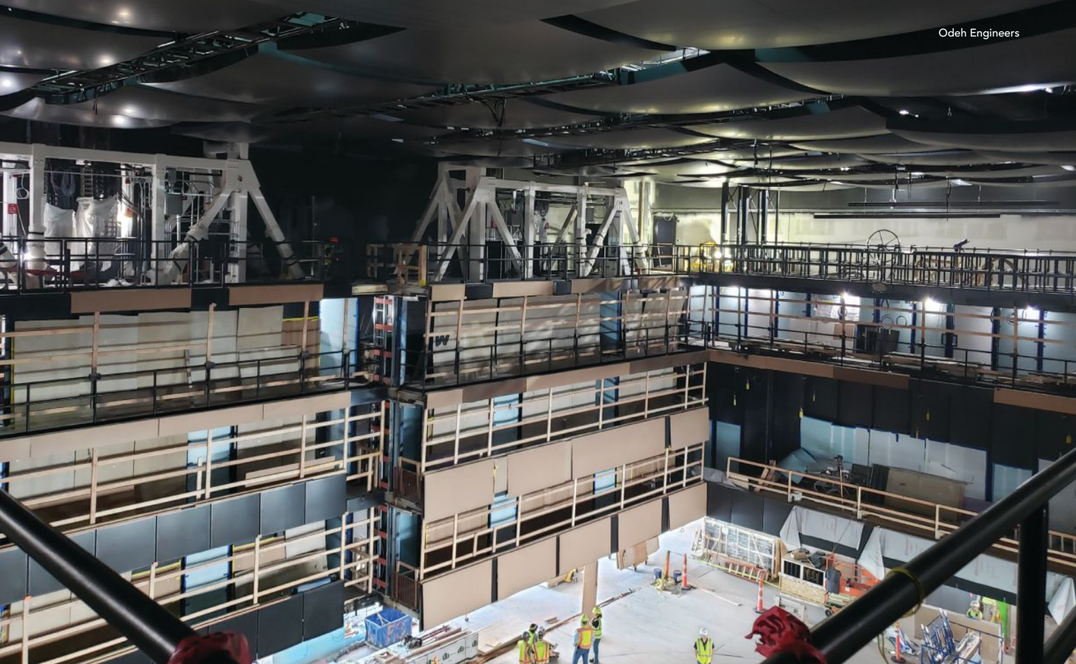
above: The side gantries can move 10\frac{1}{2} ft toward the center of the hall, and the rear gantries can move up to 44\frac{1}{2} ft toward the stage.
