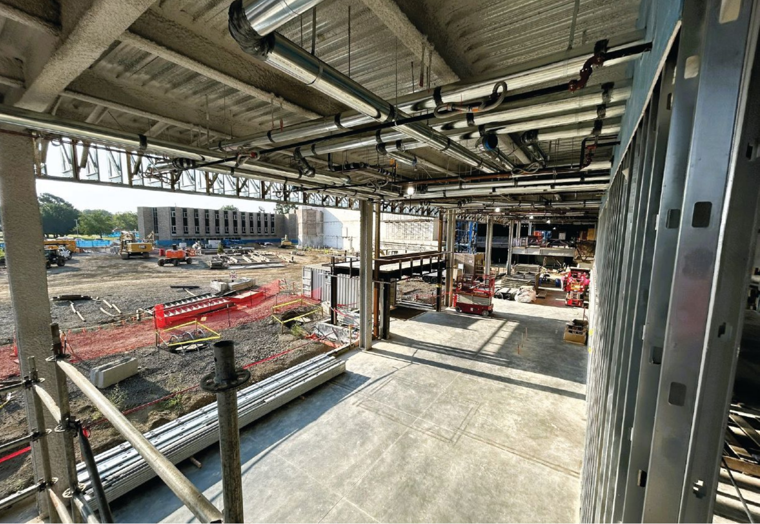
above: The two-story lobby framing under construction.
