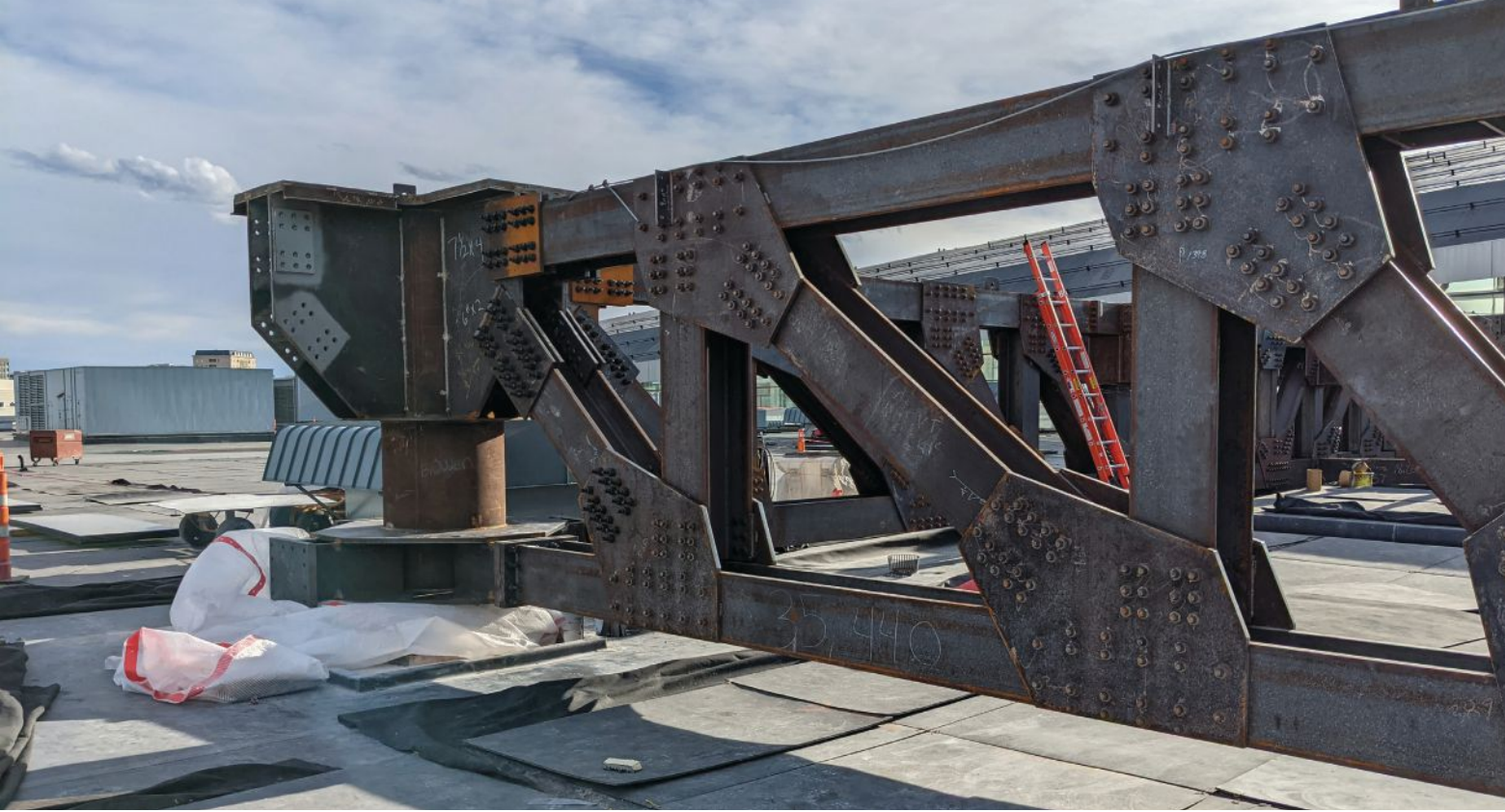
above: A floor truss attached to a column node.
