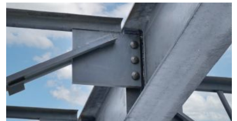
Joist reaction point occurs at beam centerline
