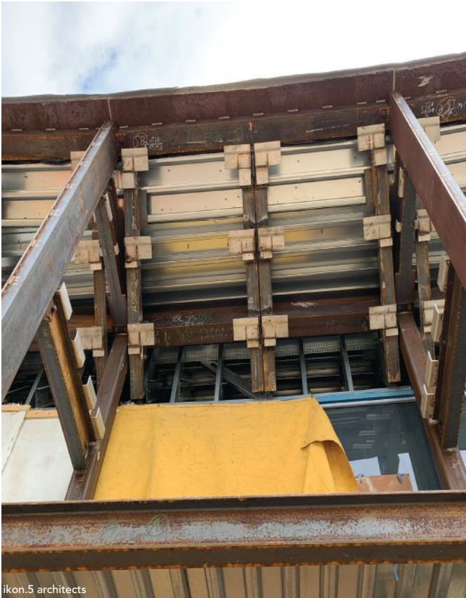
The stainless steel Z-clips awaiting weathering steel panels.
