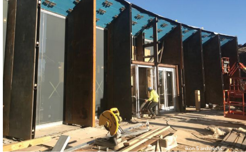
above: The panels are ASTM A588 weathering steel.
