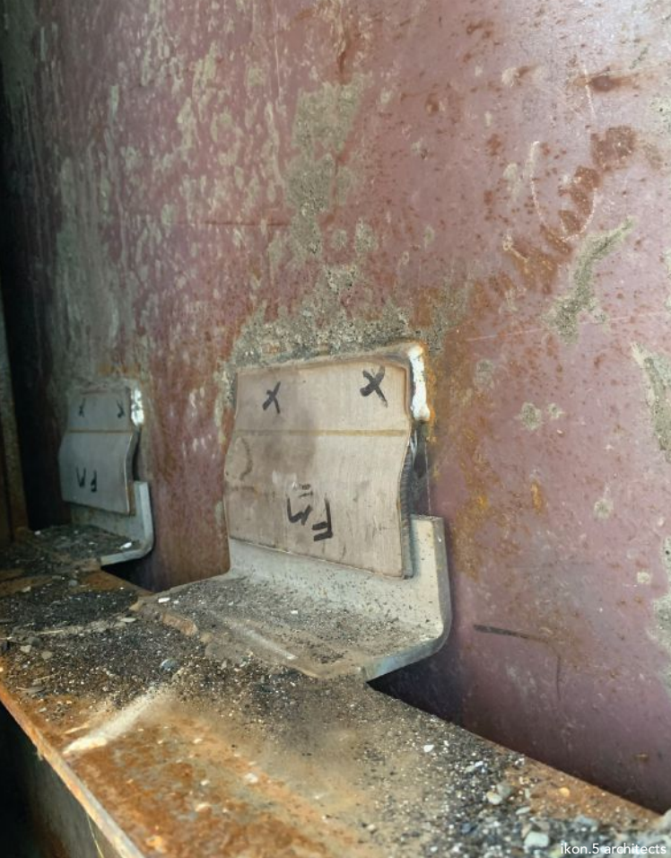
above: The Z-clips are welded to the back of the panels and framing.
