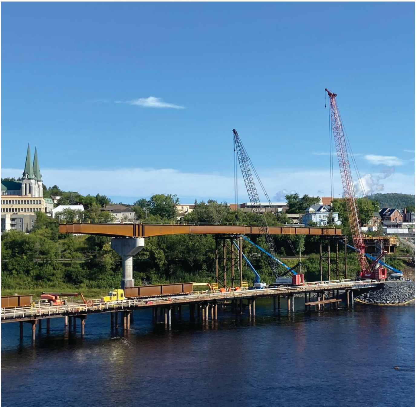
The I-shaped plate girders are made of Grade 50W and 70W uncoated weathering steel.
