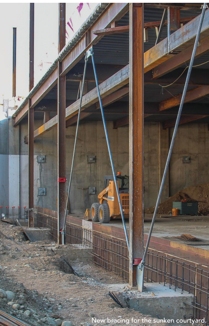
Soil anchors for the sunken courtyard.
