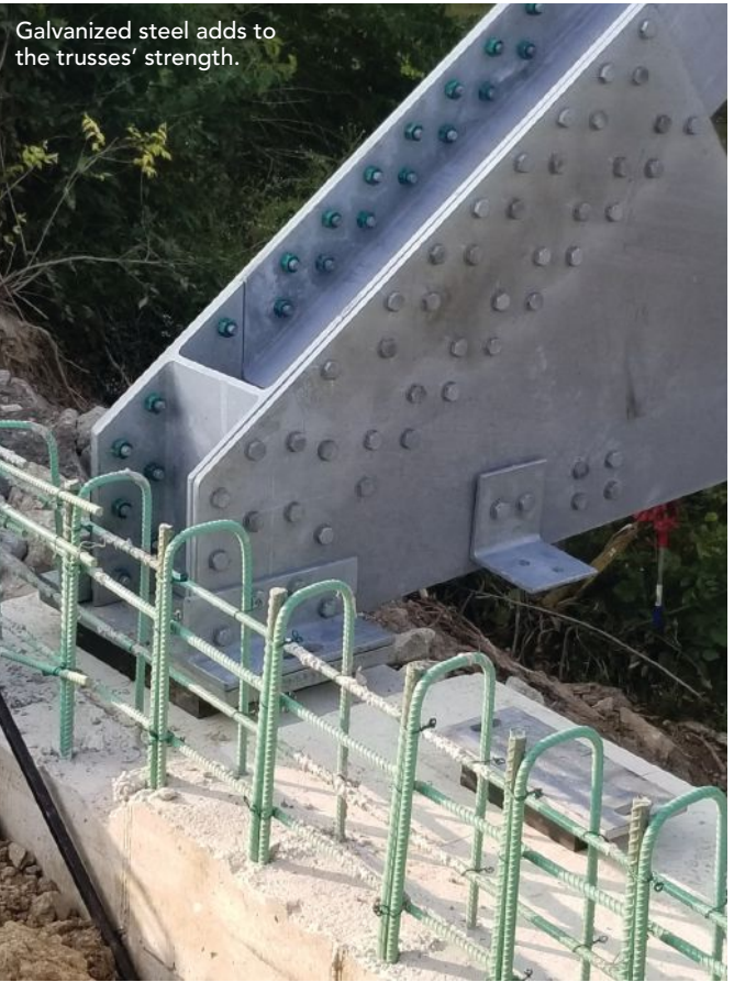
The galvanized members are expected to provide corrosion protection for up to 100 years.
