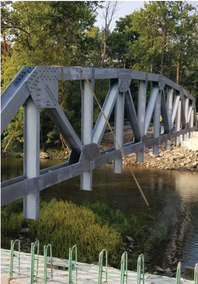
The galvanized members are expected to provide corrosion protection for up to 100 years.
