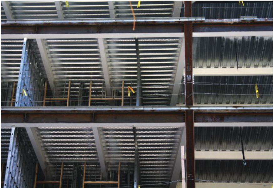
below: Upper floors have 28-ft column bays in each direction.
