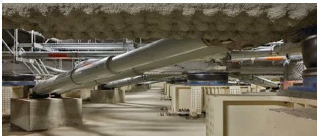
The base isolation used in the Loma Linda University Medical Center separates dangerous seismic ground motion from the critical structure above.
