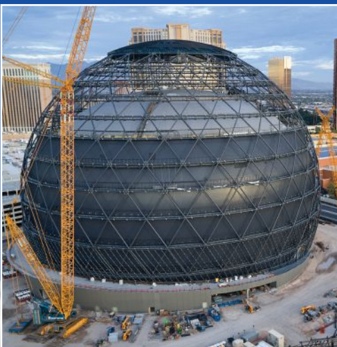
2025 IDEAS 2 Presidential Award Winner - 690 tons of curved 8" pipe and 7.5" tube, totaling 1,160 pieces for the MSG Sphere. Las Vegas, NV
