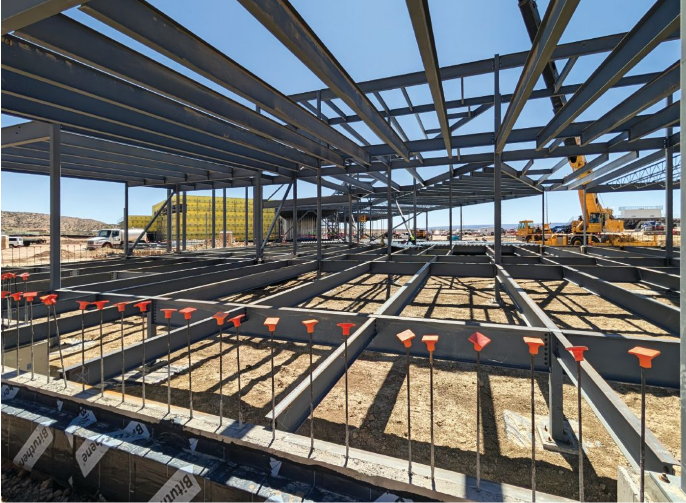
above: The building transitions to steel braced frames above Level 1 to resist lateral loads.
