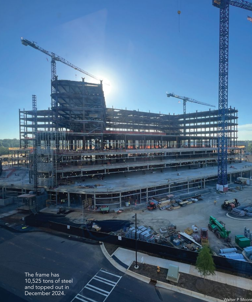
The moment frame system enabled maximum functional flexibility for initial and future architectural planning of spaces.
