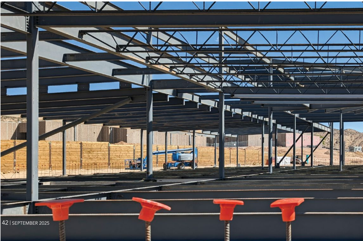
above: The building transitions to steel braced frames above Level 1 to resist lateral loads.
