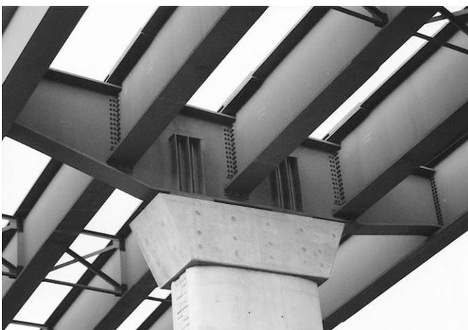
**Figure 3.15.1-5.** An integral steel pier cap used to avoid a conventional concrete rectangular cap (concrete drop cap). This allows the use of a radial cap while still maintaining adequate vertical clearances over traffic below the bridge. This is a single steel pier cap; some designers and some owner agencies prefer using a double I-beam cap to address redundancy issues.
