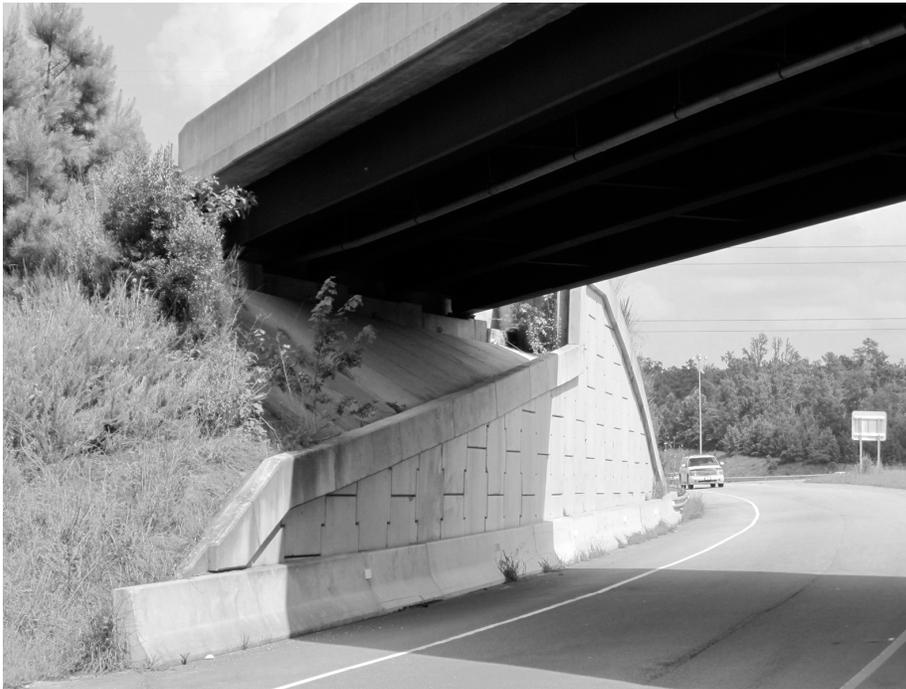
**Figure 3.15.1-4.** A steel girder bridge where a small mechanically stabilized earth (MSE) retaining wall was used to reduce the severity of skew without significant increase in span length.
