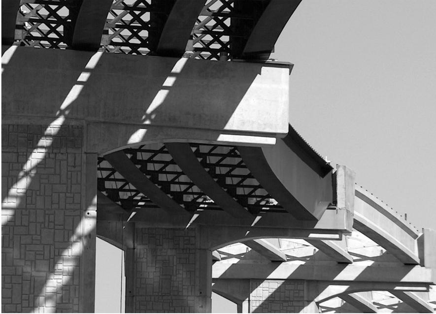
**Figure 3.15.1-7.** Dapped ends on curved steel plate girders resting on an inverted-tee bent cap on a bridge in Texas. In this case, the dapped girder ends were used to match the depth of the precast girders in the next span; but this same concept could be used to allow use of a radial bent cap the same depth as the girders, providing an effect similar to that of an integral bent cap.
