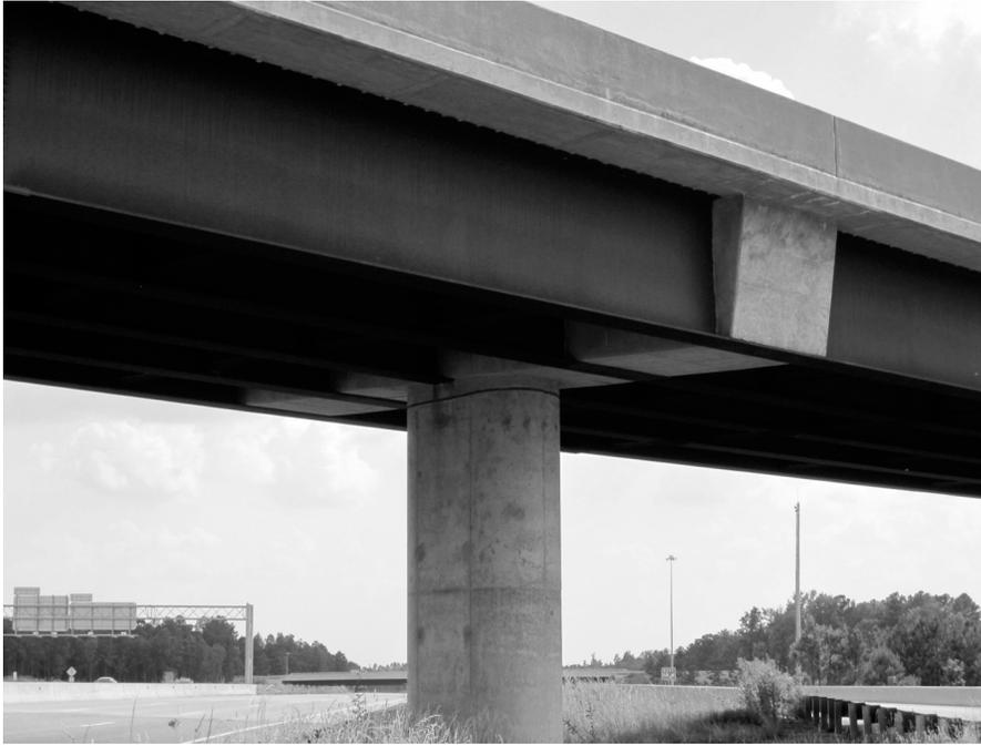
**Figure 3.15.1-6.** An integral post-tensioned concrete pier cap used in an interchange in Raleigh, NC to avoid a conventional concrete rectangular cap (concrete drop cap). This allows the use of a radial cap while still maintaining adequate vertical clearances over traffic below the bridge.
