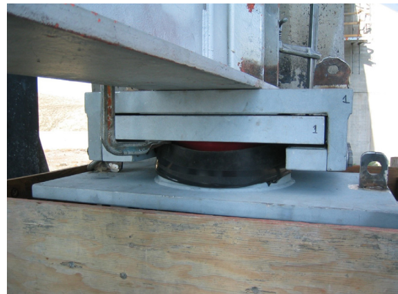
Figure C3.7-1. Field Welding of Disc Bearing
