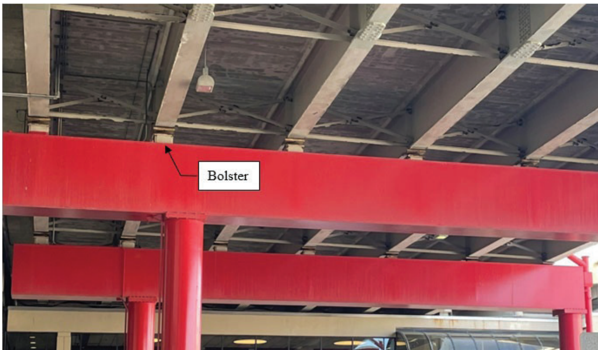
Figure 2.3.2-2—Example of bolsters
