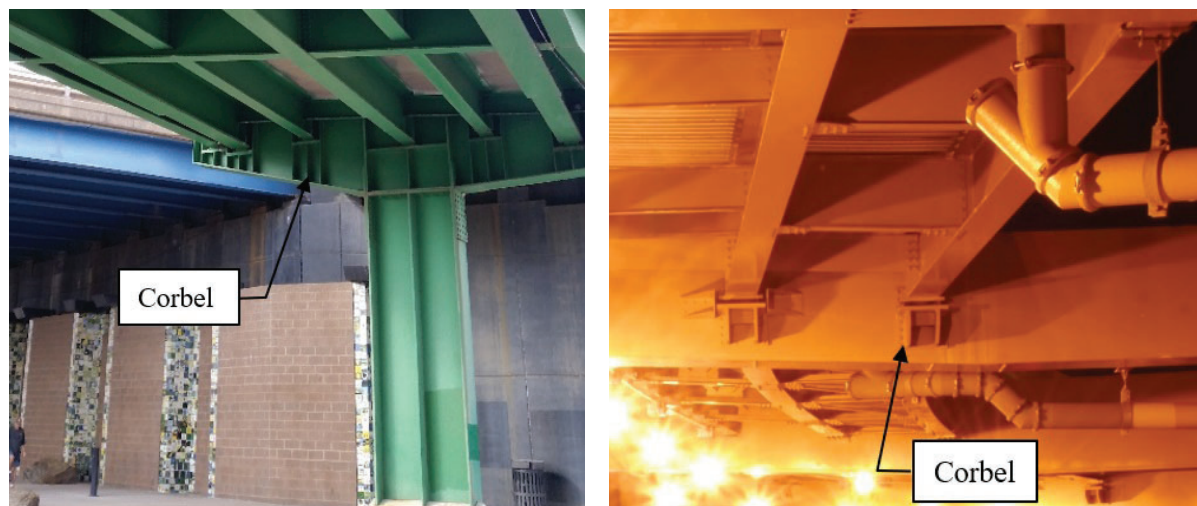
Figure 2.3.3-1—Examples of corbels
