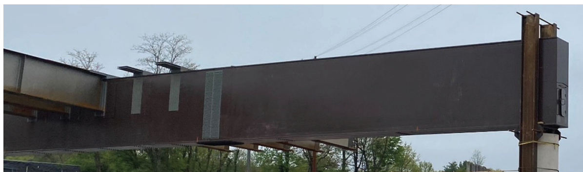
Figure 5.4-5—Erection of steel bent cap
