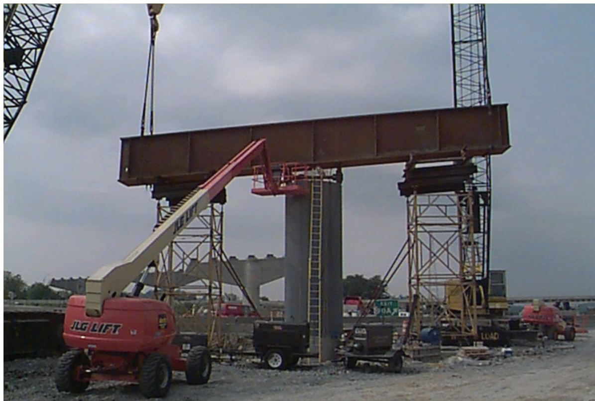
Figure 3.9.1-2—Hinged hammerhead steel bent cap
