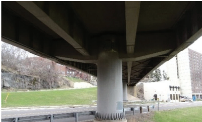
Figure 2.2-2—Examples of integral straddle and hammerhead bent caps with tapered webs
