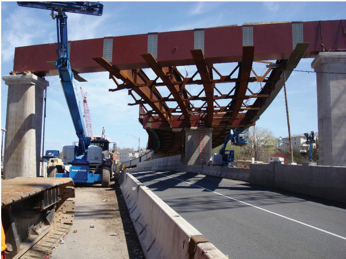
Figure 5.4-1—Erection of a steel bent cap
