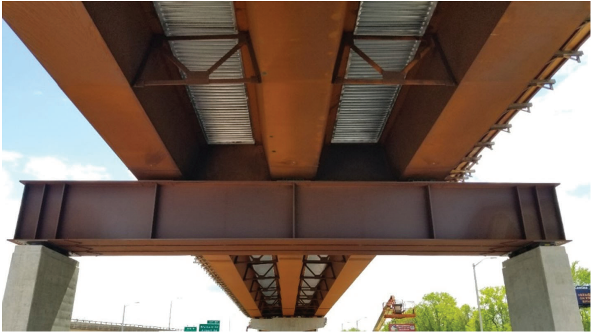
Figure 3.15-1—Triple I-girder steel bent cap with longitudinal tub girders
