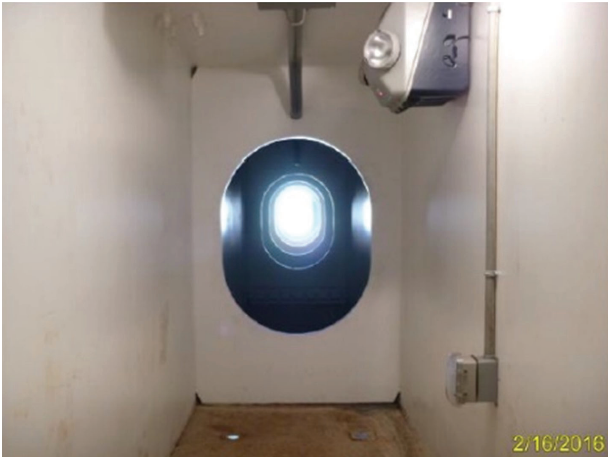
Figure 4.8-1—Interior of steel box-shaped bent cap
