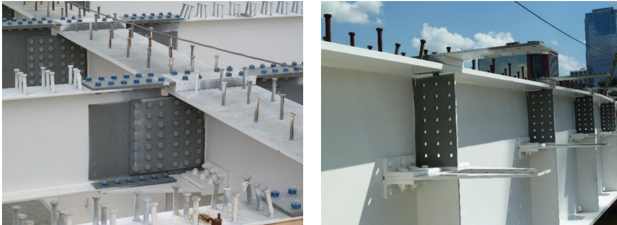
Figure 3.12.1-1—Integral longitudinal girder connections
