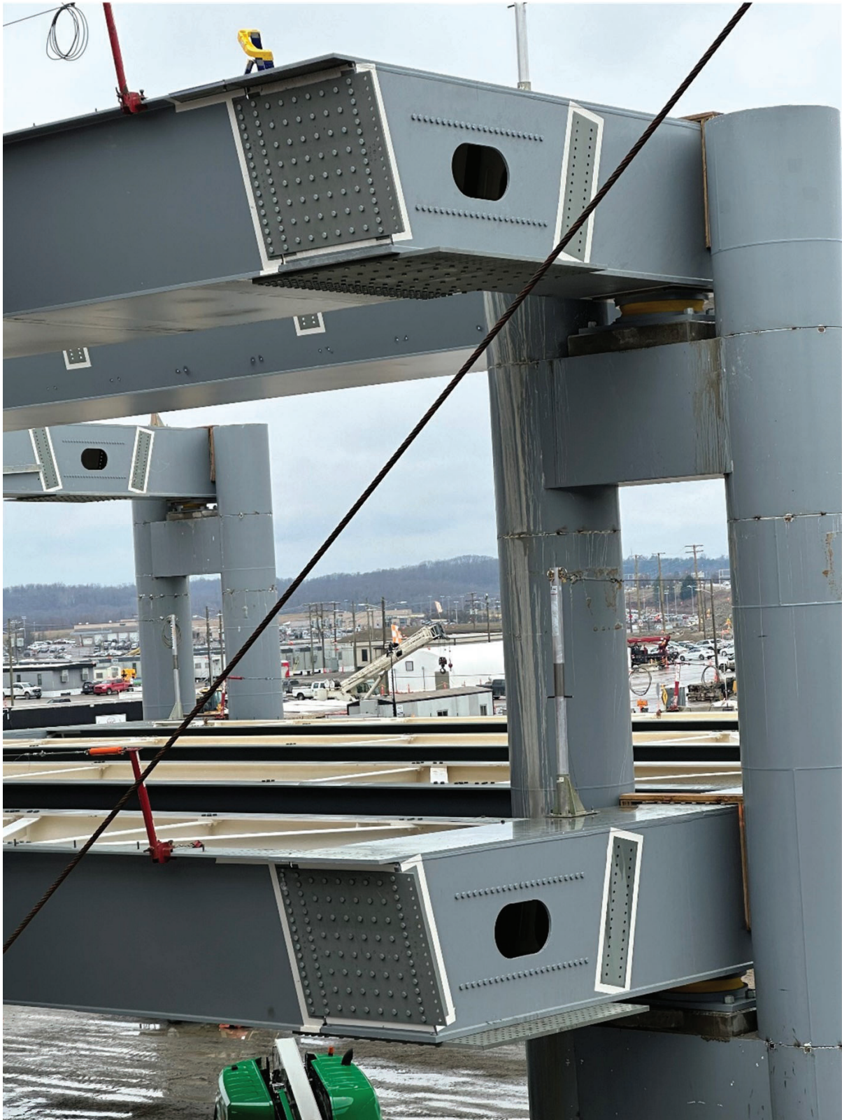
Figure 5.4-2—Geometry control of a steel bent cap
