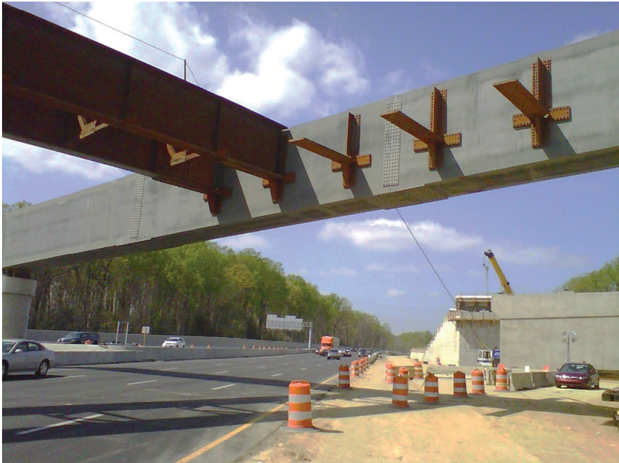
Figure 5.4-3—Supports for longitudinal girders at integral steel bent cap
