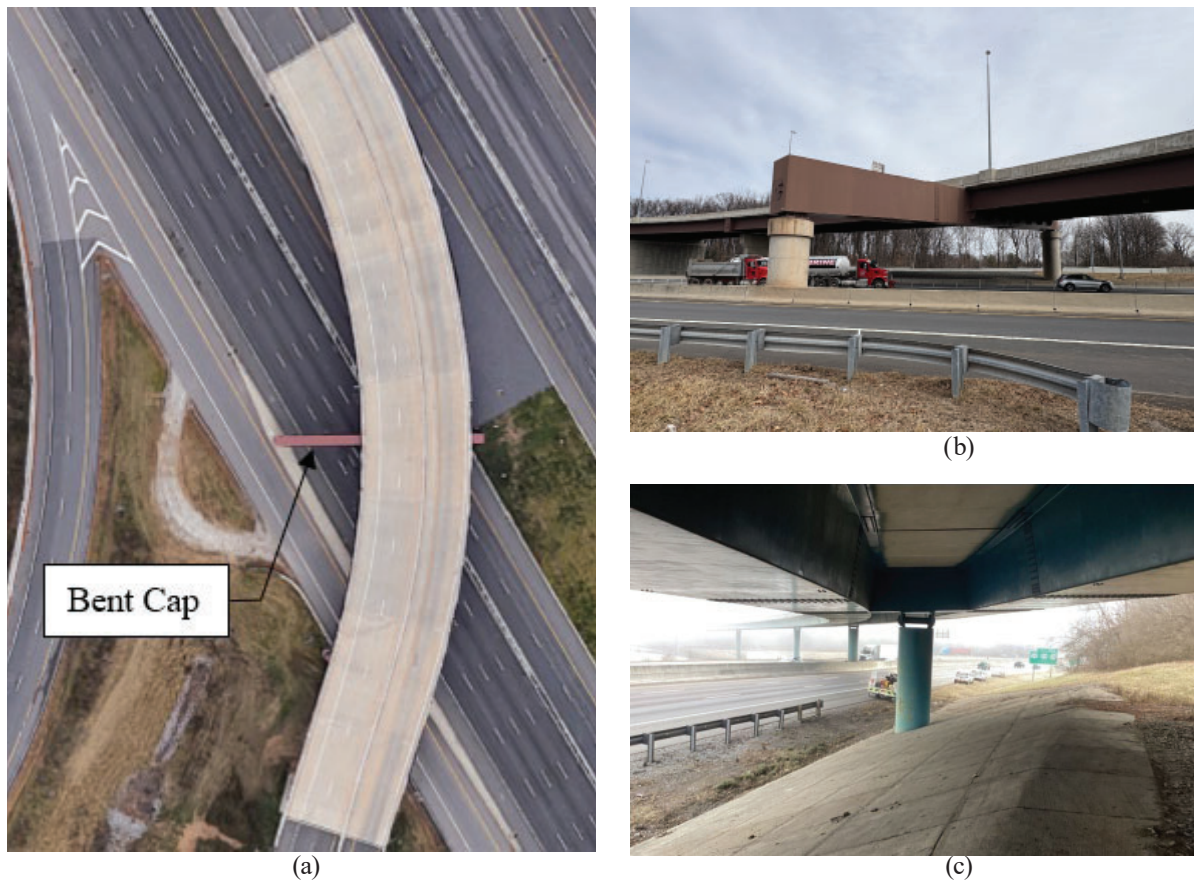
Figure 2.1-1—Example of roadway geometry requiring a simple-span bent cap supported on two columns (a and b) and a single-column hammerhead bent cap (c)
