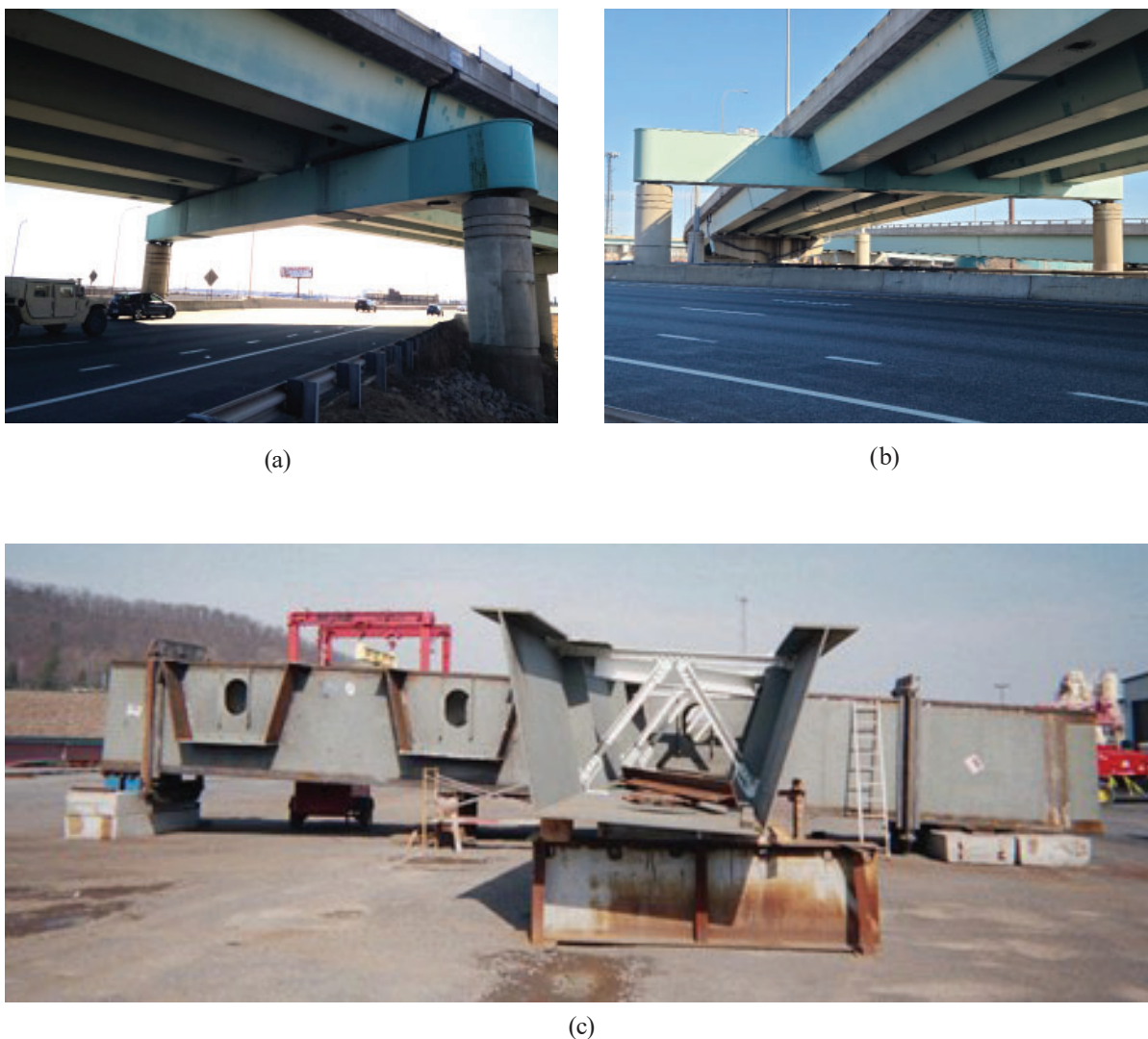
Figure 5.1-1—Bent caps, with (a) in-line, integral bent cap, (b) stacked bent cap, and (c) integral cap in shop assembly
