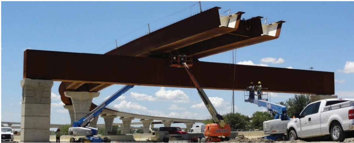
Figure 2.3.2-1—Non-integral, stacked connection
