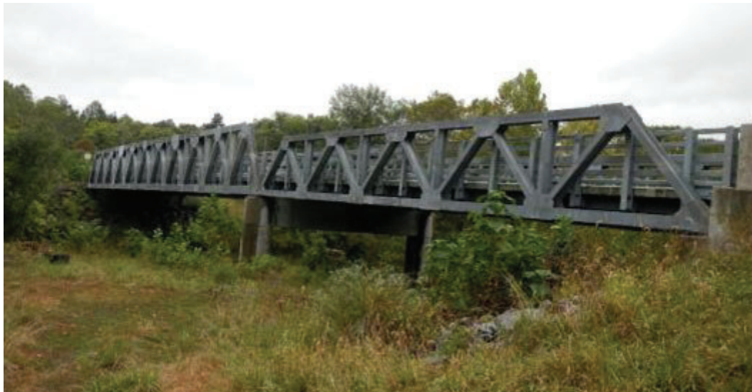
Figure A1.2-1—Virginia Albemarle County pony truss.
