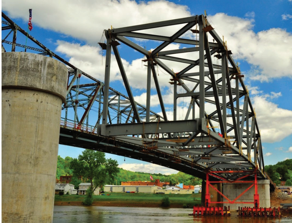
Figure A2.2.6-1—Cantilever truss during erection.
