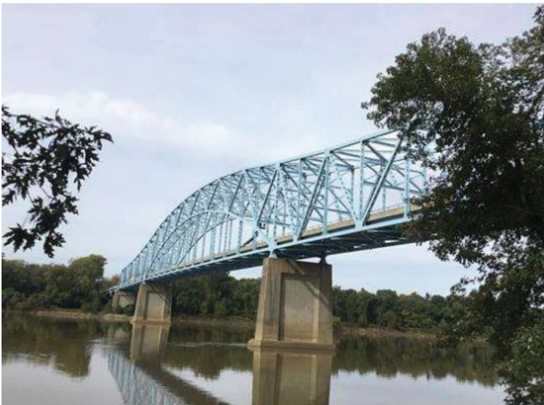
Figure A1.3-1—Overall view of Wabash Memorial Bridge.
