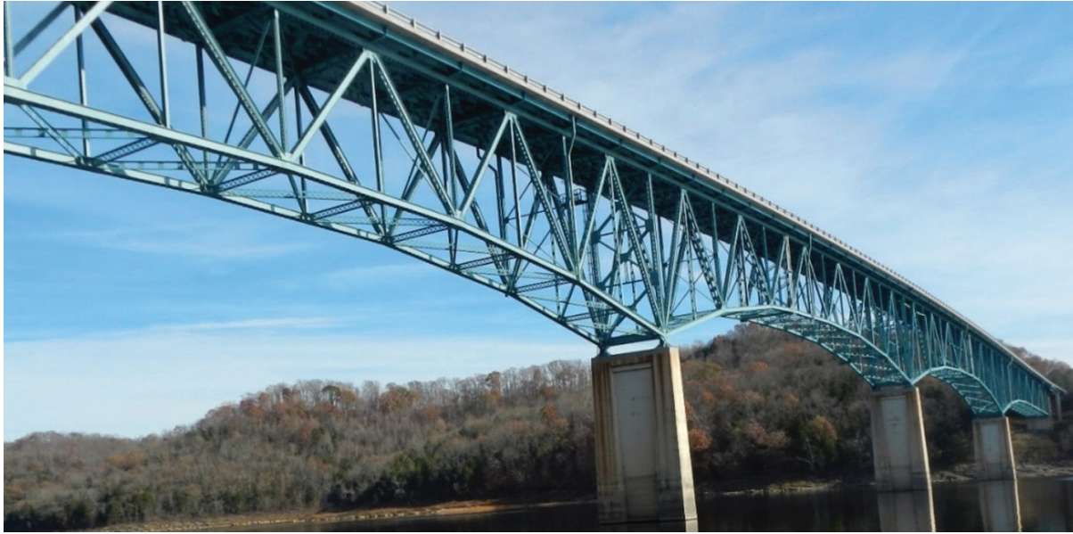
Figure A3.1-1—Hurricane Bridge photograph.
