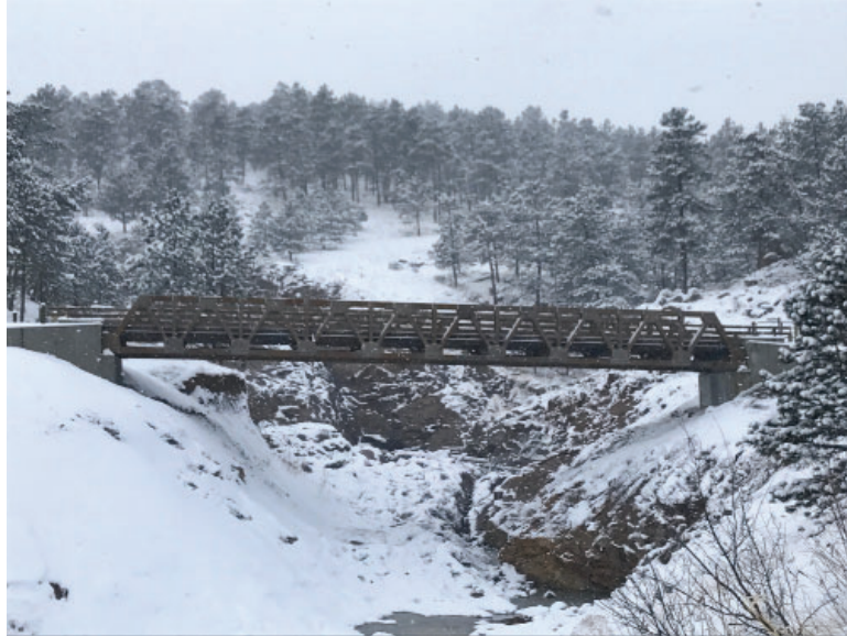
Figure 1.1-4—Simple-span pony truss.
