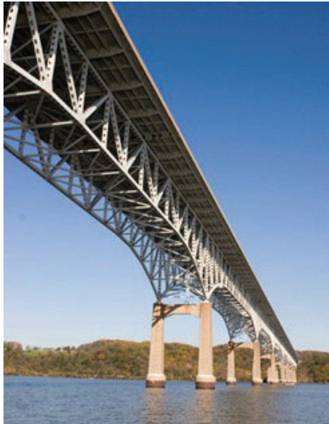
Figure A1.4-1—Perspective view of Tydings Bridge, MD.
