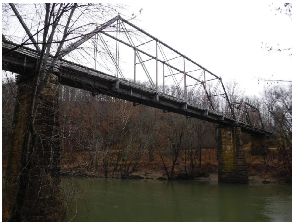
Figure A1.1-1—KY-644 Bridge over Levisa Fork of the Big Sandy River, KY.
