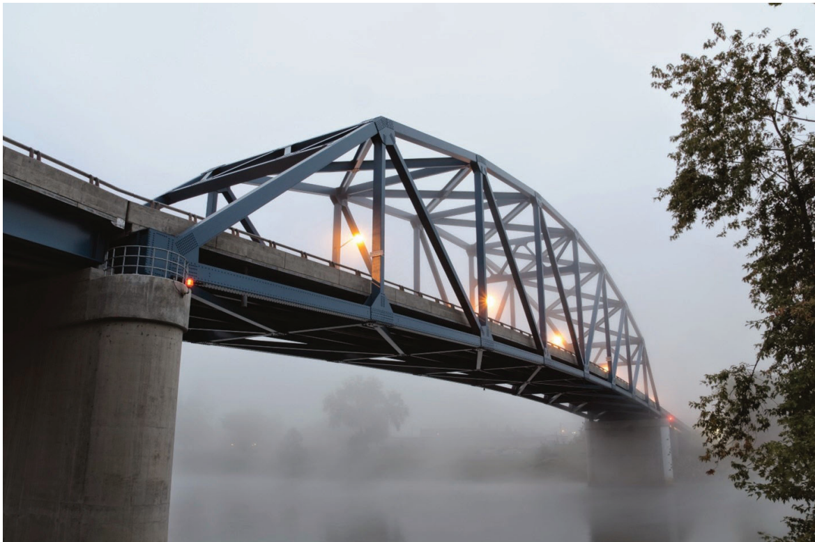
Figure A2.2-1—Point Marion Bridge, PA.
