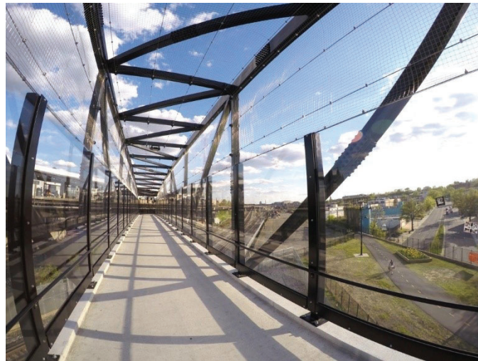
Figure A3.2-1—Rhode Island Avenue Pedestrian Bridge, Washington, D.C.
