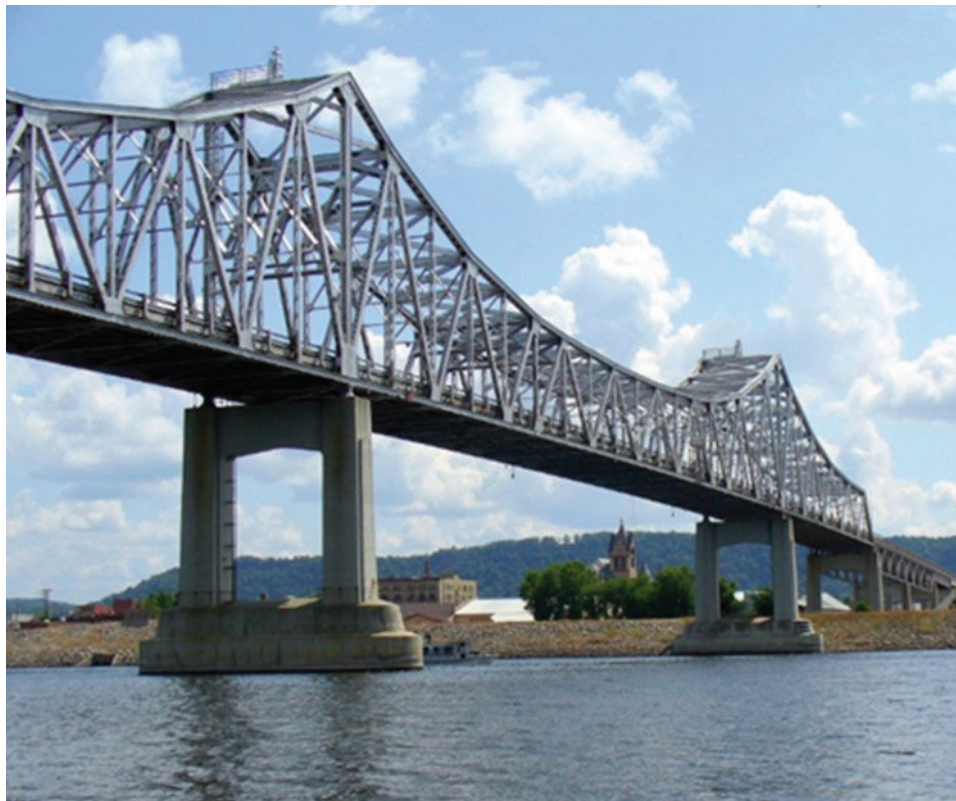
Figure A3.5-1—Winona Bridge 5900 through-truss bridge in Winona, MN.
