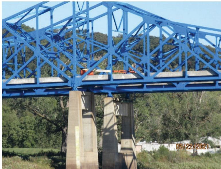
Figure 1.1-5—Continuous through-truss bridge.
