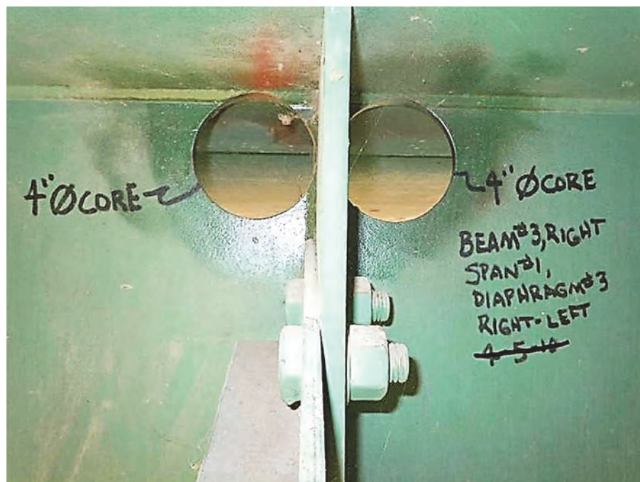
Figure 5-11. Large-Hole Retrofit—Note Interception of Horizontal and Vertical Weld Toes (Photograph courtesy of Iowa DOT)
