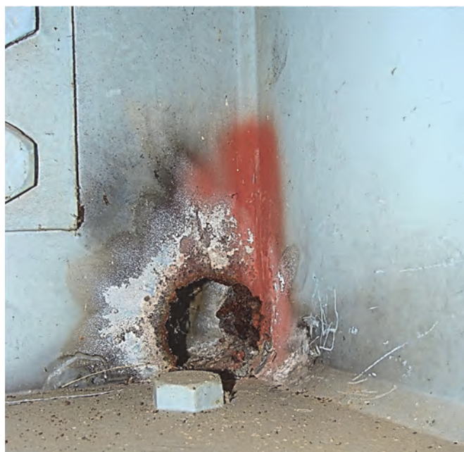
Figure 4-34. Poor Quality Flame-Cut Hole That is Prone to Fatigue and Fracture
