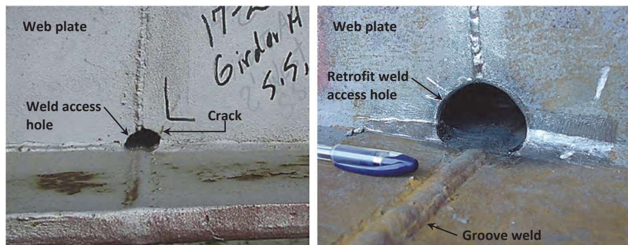
Figure 4-35. Repair of a Cracked Weld Access Hole Showing before (Left) and after (Right) (Photographs courtesy of Kansas DOT)
