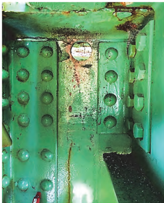
Figure 5-19. Drilled Hole Prior to Sanding Edges
