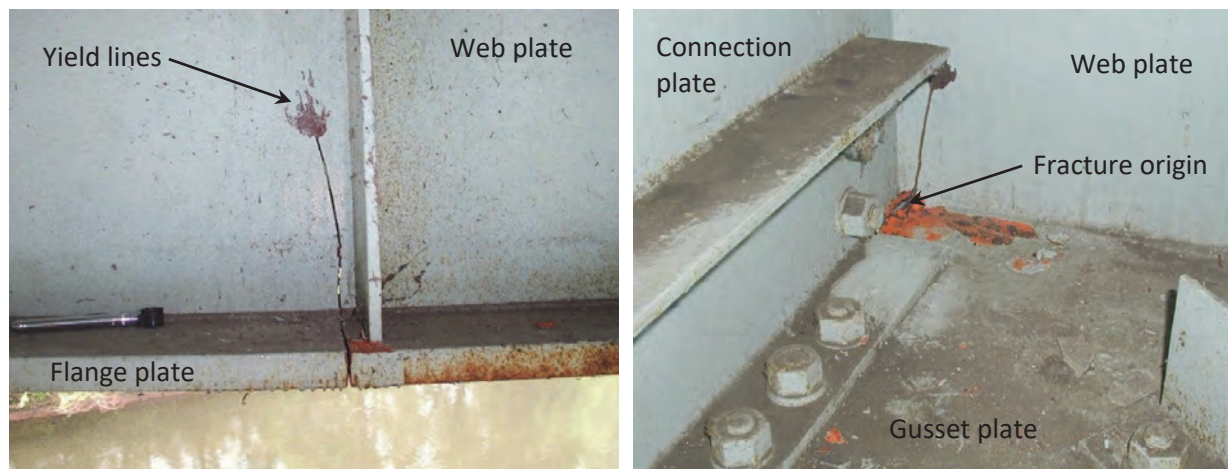
Figure 6-2. U.S. 422 Bridge Fracture That Arrested in the Web
