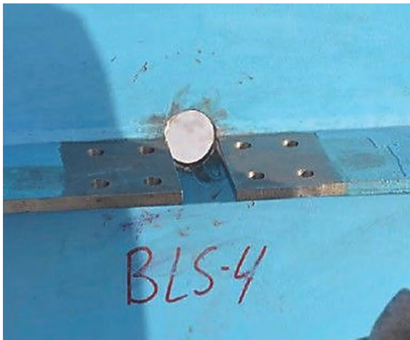
Figure 6-29. Finished Retrofit with Drilled Holes for Optional Bolted Splice
