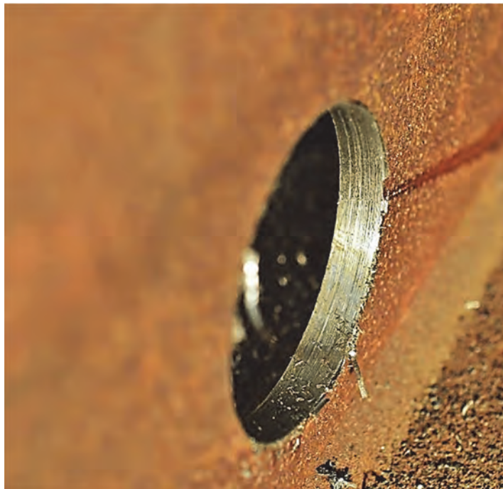
Figure 3-6. Drilled Hole Showing Rough Edges and Burrs
