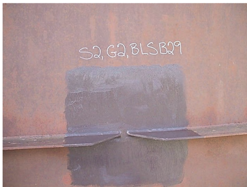
Figure 6-25. Alternate Version of the Longitudinal Stiffener Core Retrofit with the Stiffener Plates Cut Back in Addition to the Drilled Hole
