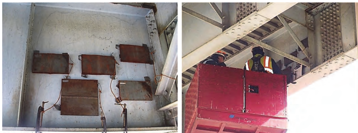
Figure 3-20. (Left) Welded Steel Test Specimen Hung on a Bridge, (Right) Performance Testing of an Inspector Prior to Beginning NDT on Bridge Welds
