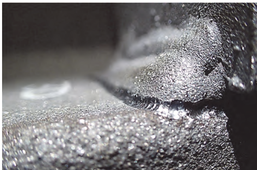
Figure 3-17. Appearance of Properly Treated Weld Toe Using UNP Method
