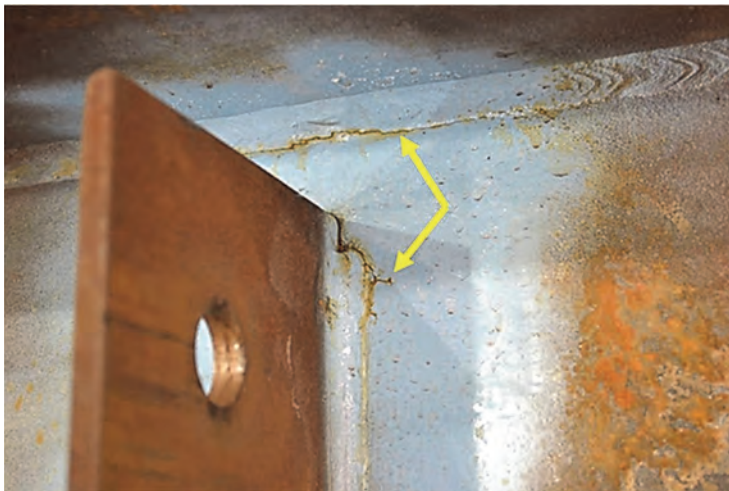
Figure 5-3. Example of Web Gap Cracking Resulting from Distortion
