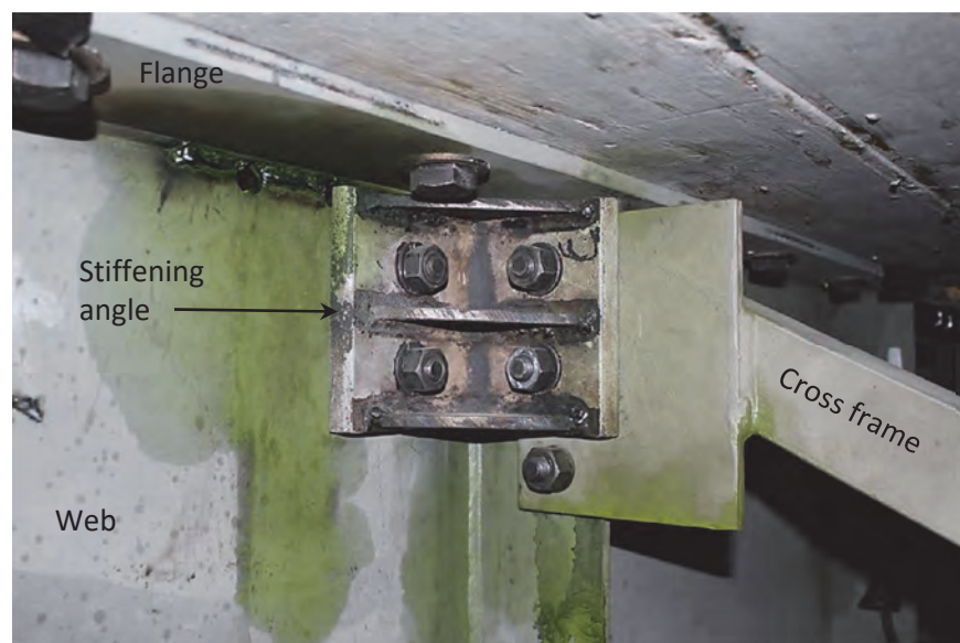
Figure 7-2. Stiffened-Angles-with-Plate Retrofit (Taken From Bennet Et Al., 2014)
