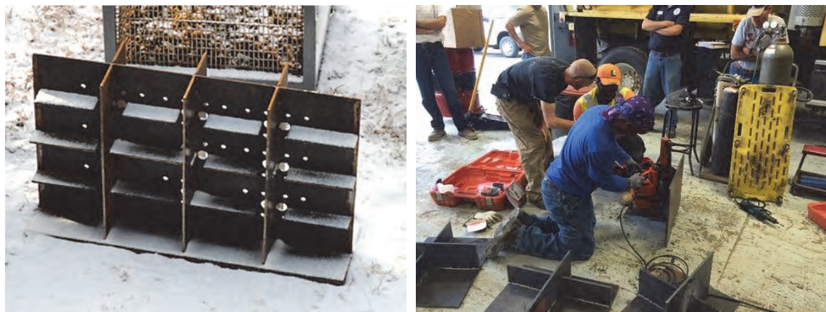
Figure 3-19. (Left) Example of Used Mockup, (Right) Performance Testing of a Contractor Prior to Implementation of a Repair Project
