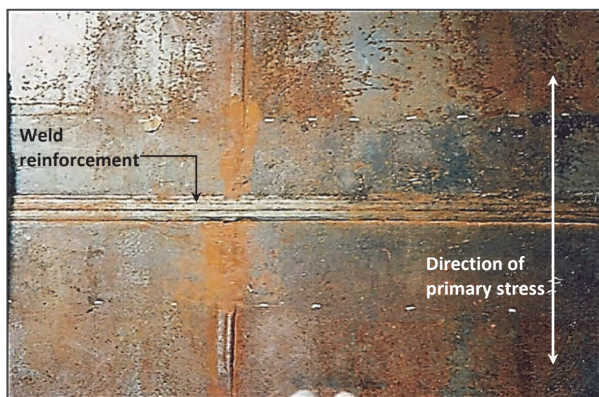
Figure 4-31. Category C Transverse Groove Weld
