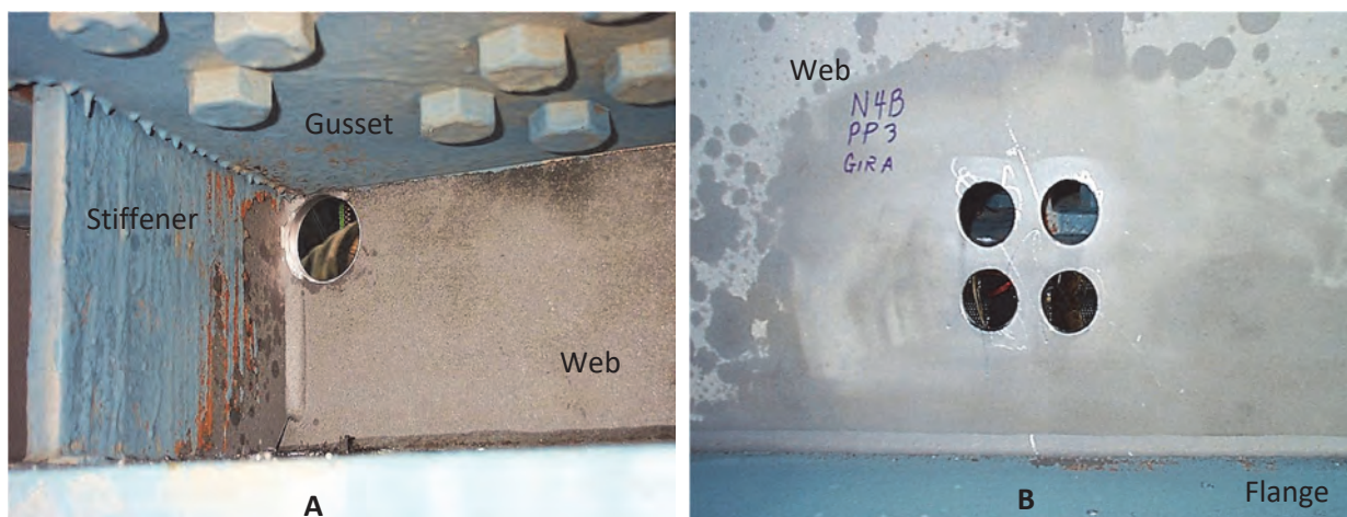
Figure 6-13. Web Isolation Holes Retrofit on the Hoan Bridge (A) beneath the Gusset, (B) Opposite Side of Gusset (Photographs courtesy of Phil Fish)
