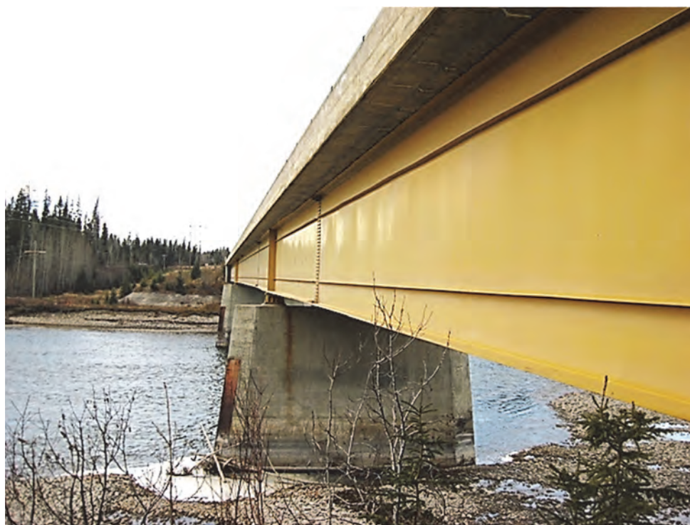
Figure 4-20. Example of Longitudinal Stiffeners Located in Tension and Compression Zones
