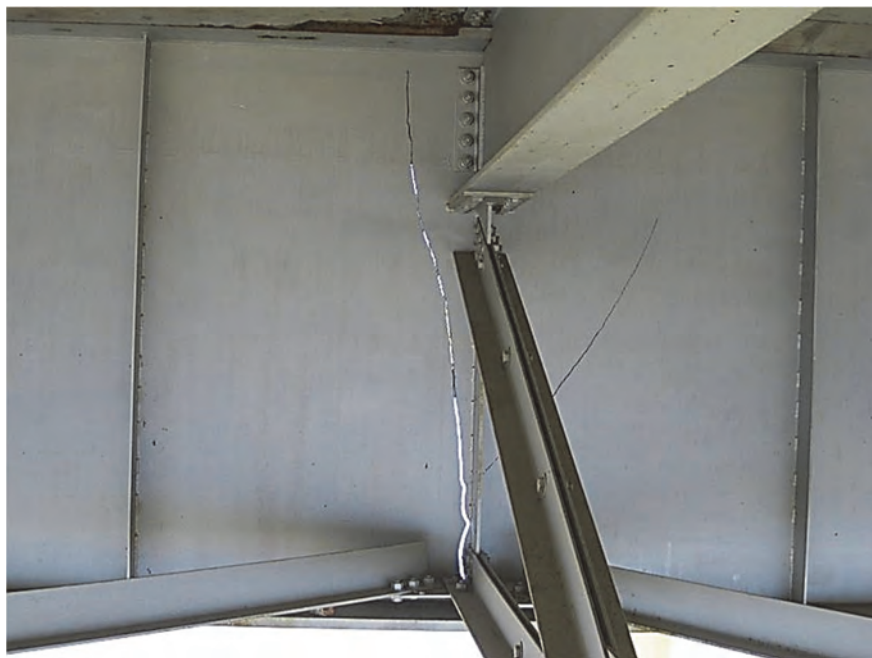
Figure 6-14. Diefenbaker Bridge Fracture Originated at CIF-Prone Detail
