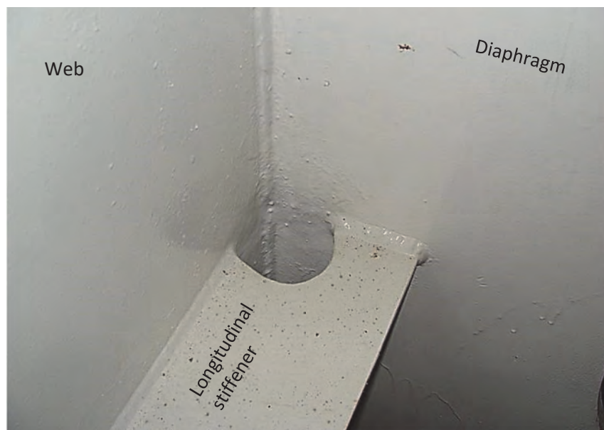
Figure 6-19. Hoan Bridge Longitudinal Stiffener CIF Retrofit
