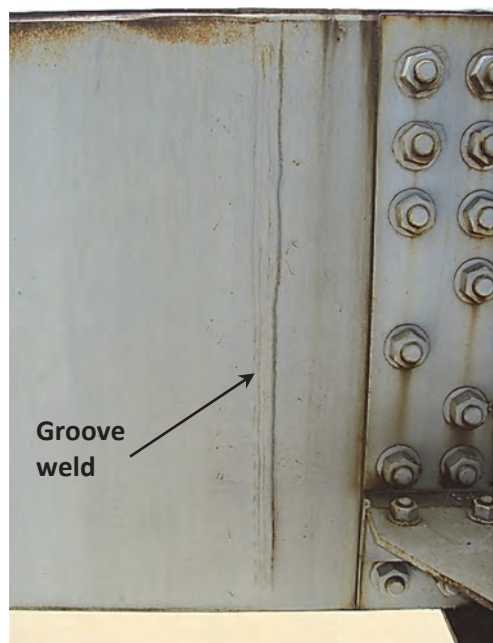
Figure 4-30. Transverse Groove Weld with Reinforcement Left in Place (Category C)
