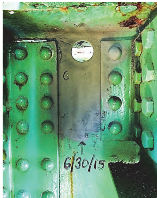
Figure 5-20. Finished Repair with Zinc-Rich Paint
