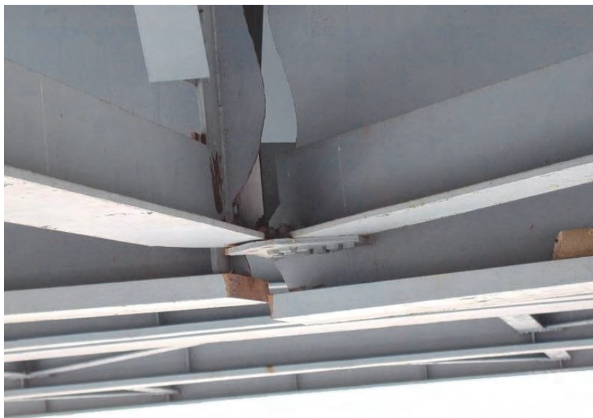
Figure 6-6. Hoan Bridge Fracture Showing the Gusset Detail of the Interior Girder
