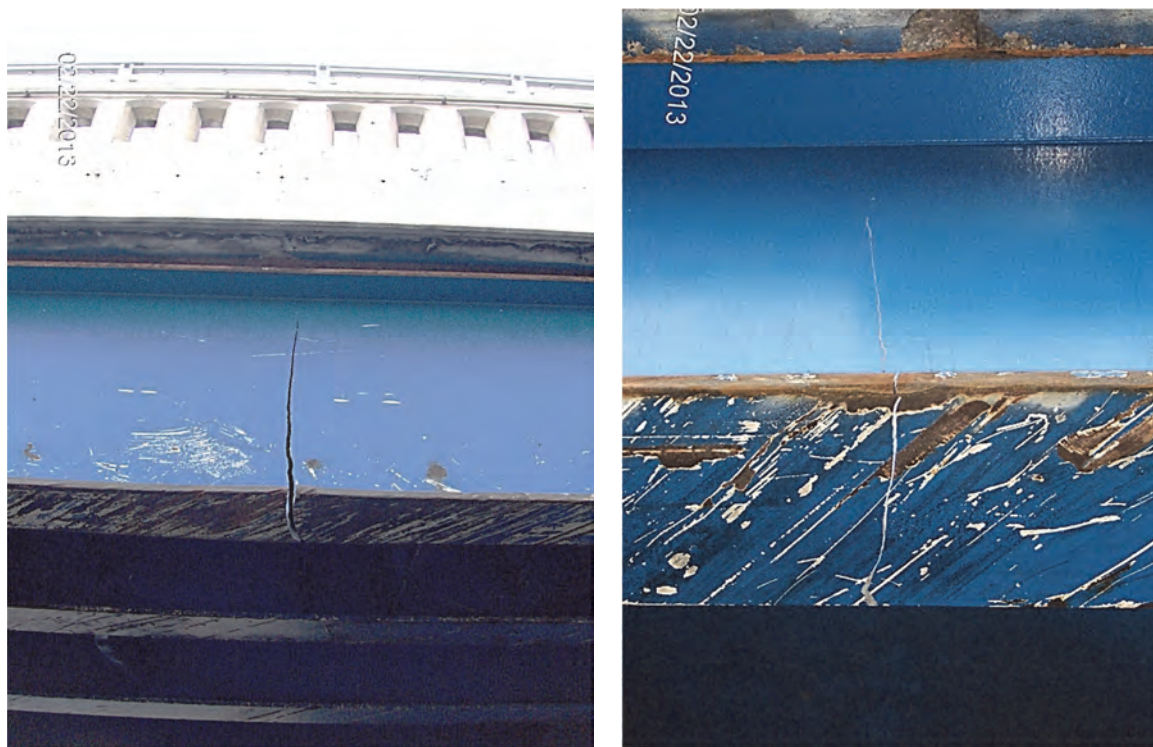
Figure 4-47. Fractures on the Same Girder Resulting from a Single Impact Event
