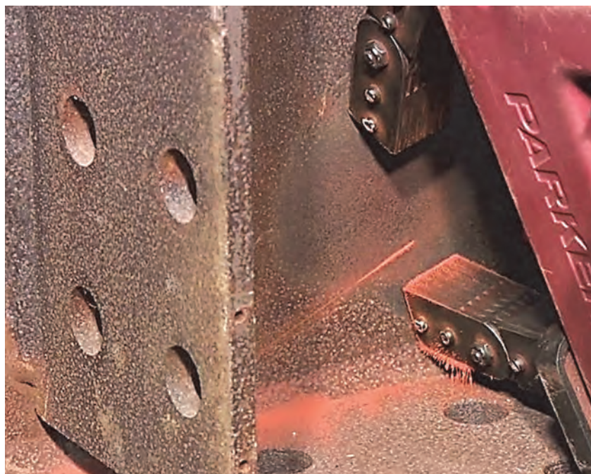
Figure 3-7. Magnetic Particle Test Performed Before Drilling Crack Arrest Hole in Order to Locate the Crack Tip
