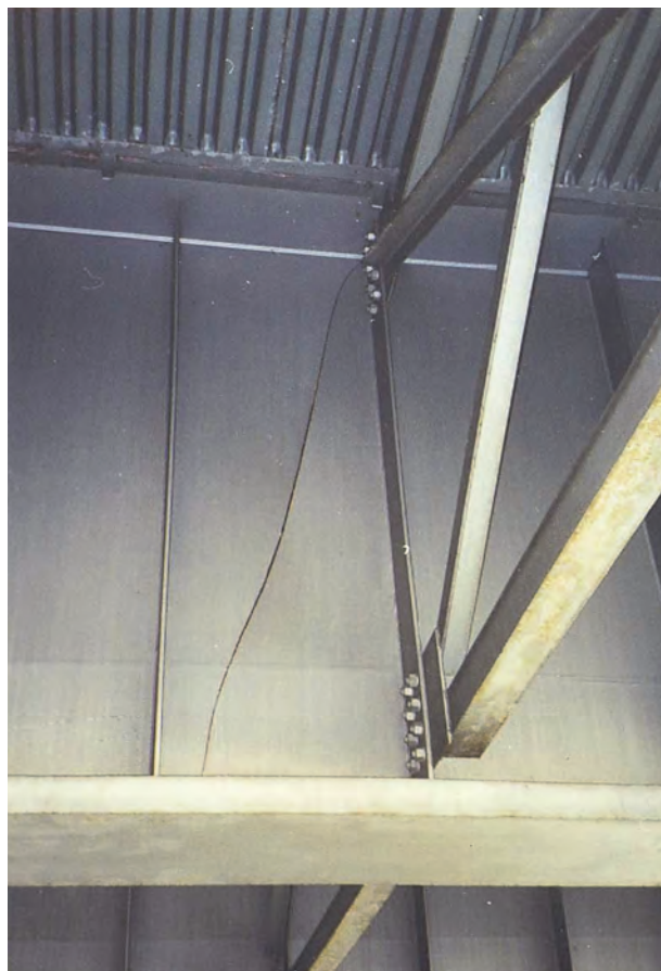
Figure 6-32. Fracture Initiated at Stiffener in Negative Moment Region (Photograph courtesy of Y. Edward Zhou)
