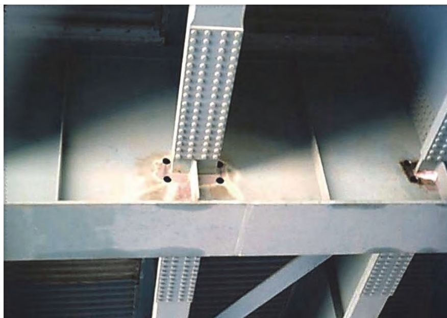
Figure 5-38. Completed Dog-Bone Retrofit on a Web Penetration Detail
