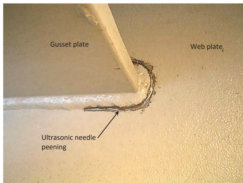
Figure 4-23. Weld Toe Peening at Gusset Plate Termination (Photograph courtesy of Iowa DOT)
