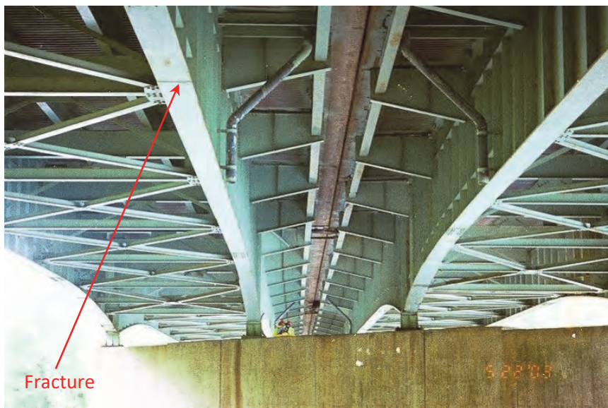
Figure 6-1. U.S. 422 Bridge Fracture Discovered in 2003 During Retrofitting
