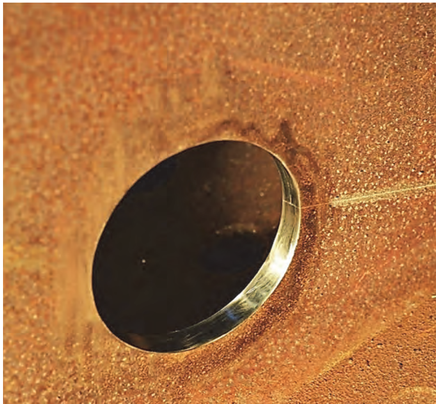
Figure 3-9. Example of Finished Crack Arrest Hole Prior to Painting
