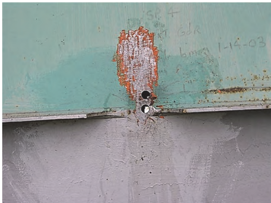
Figure 6-26. Longitudinal Stiffener Core Retrofit Showing Drilled Holes in the Web Plate for Crack Arrest (Photograph courtesy of Kansas DOT)
