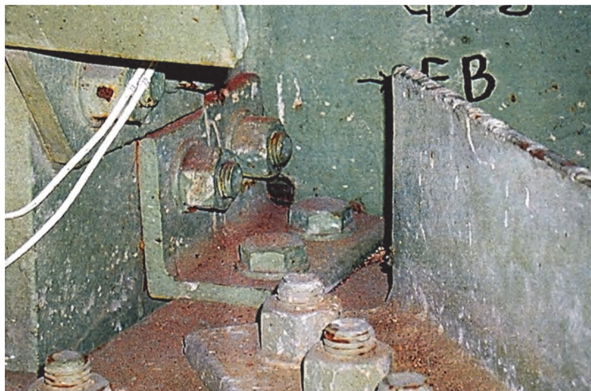
Figure 5-6. Insufficiently Stiff Splice Angle Shown Installed on Gusset–Connection Plate Web Gap
