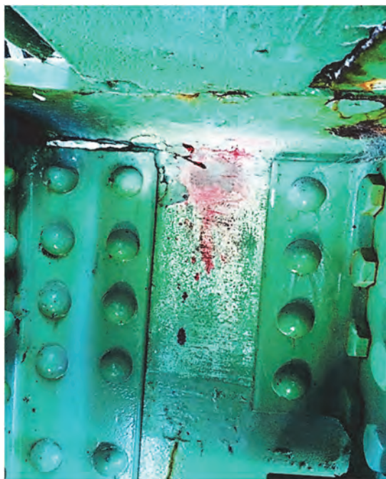
Figure 5-18. Results of PT Revealing Extent of Crack
