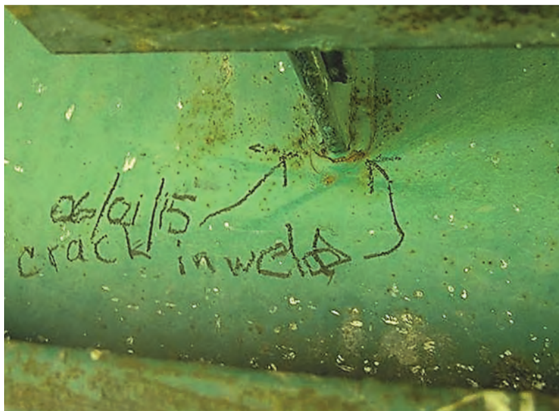
Figure 3-22. Distortion-Induced Fatigue Crack Growing out of the Throat of the Weld
