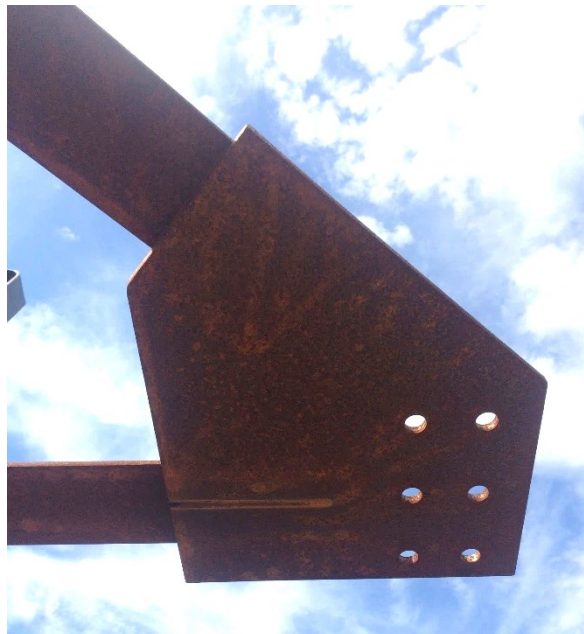
Figure C2.2.6.4-2: Photo of a cross frame where the gusset plates have clipped corners.
