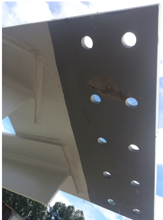
Figure C2.2.6.4-6: Photo of a cross frame where the gusset plates have non-clipped corners.
