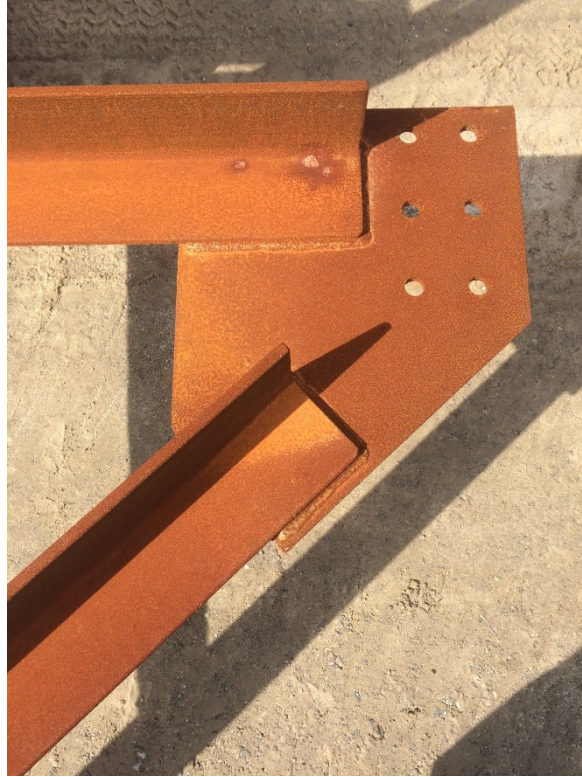
Figure C2.2.6.4-3: Photo of a cross frame where the gusset plates have clipped corners.
