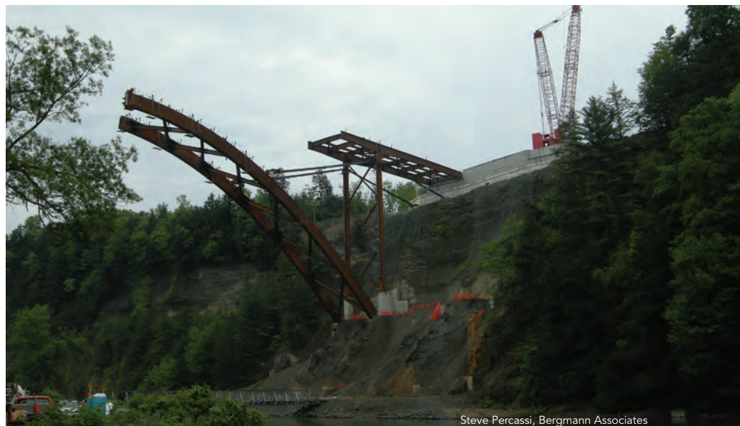
▲ ▼ The flow of wind around a completed structure is fundamentally different than it is around an open frame during construction.
