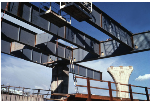
Figure 7 - Straddle Bent With Integral Steel Pier
