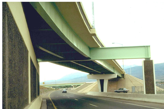
Figure 8 - Straddle Bent With Integral Steel Pier
