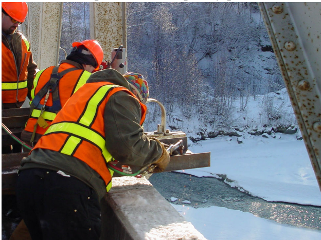
Figure 21: Slotting Holes in Temporary Portals
