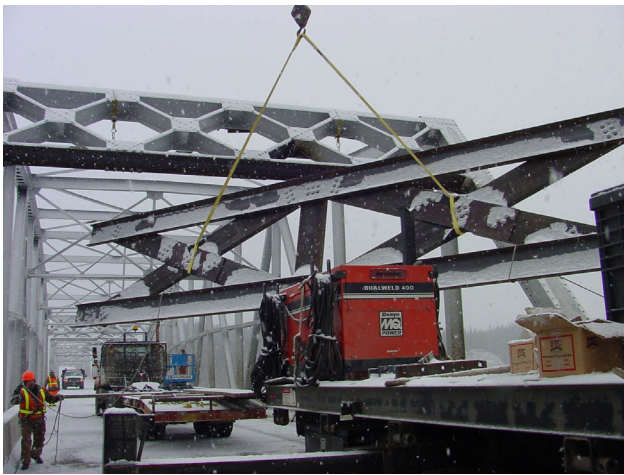
Figure 19: Removing a Temporary Portal
