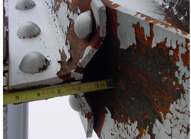
Figure 6: Deformed Connection Angles
