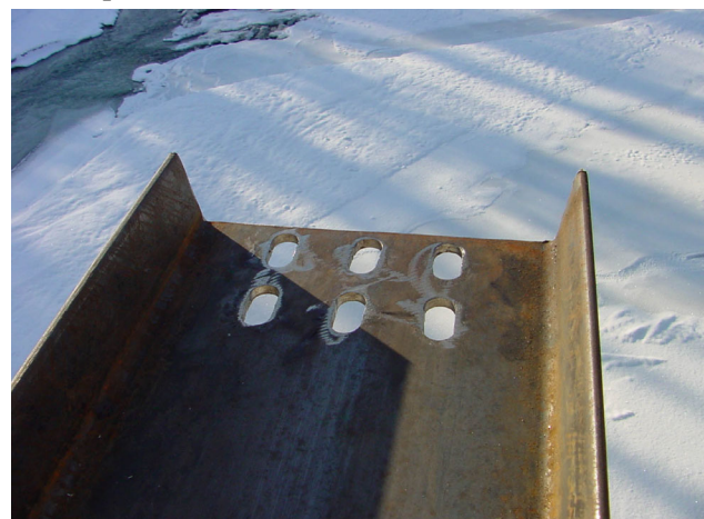
Figure 22: Finished Slots in Temporary Portals
