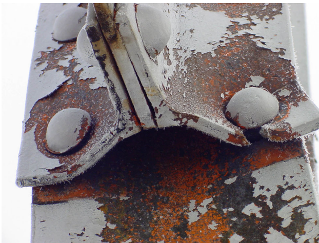
Figure 7: Torn Connection Angle
