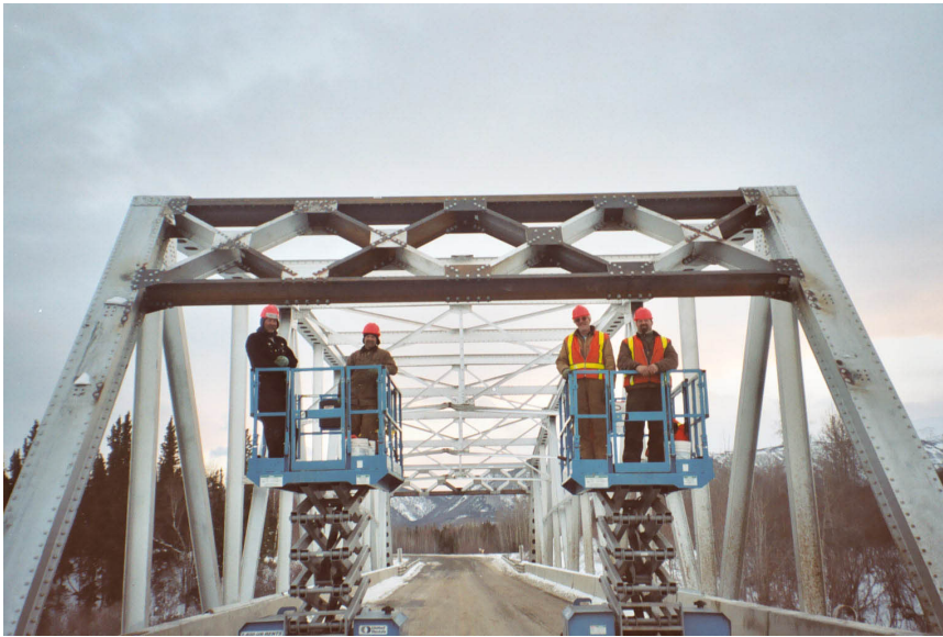
Figure 24: Bridge Maintenance Crew and Completed Portal
