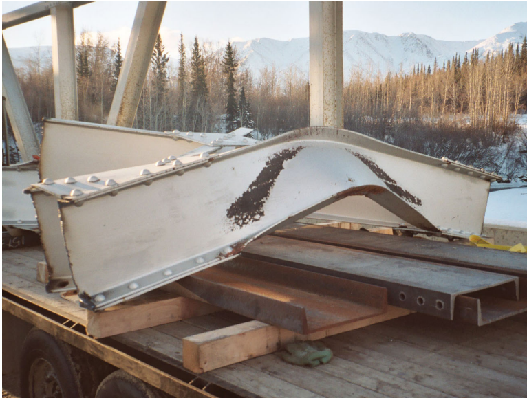
Figure 10: Damaged Span 4 Near End Portal Removed
