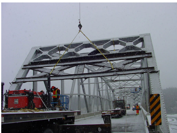
Figure 18: Rigging to Remove a Temporary Portal
