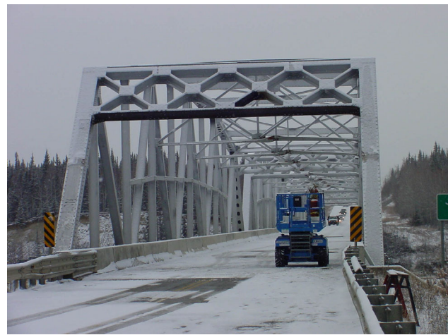
Figure 20: Completed Portal Repair
