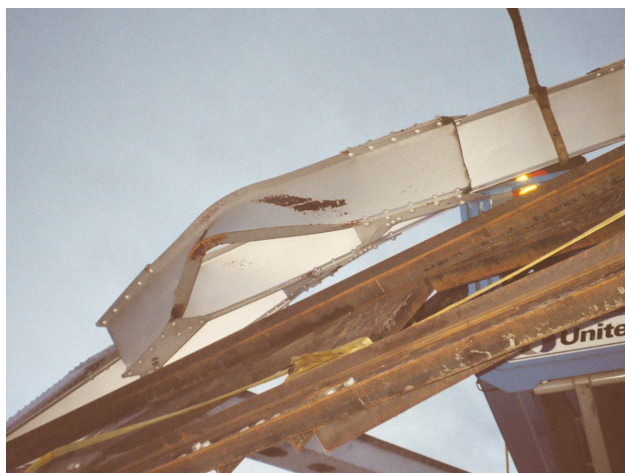
Figure 9: Damaged Span 4 Near End Portal In Place
