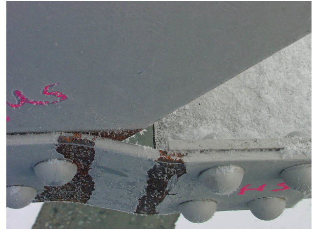
Figure 8: Buckled Connection Plates
