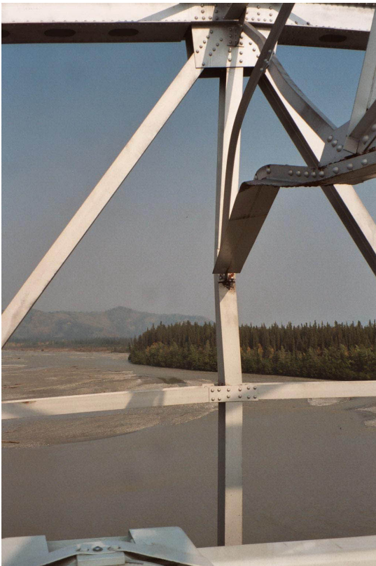
Figure 4: Damaged Sway Bracing
