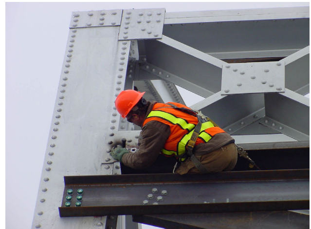
Figure 17: Aligning Bolt Holes
