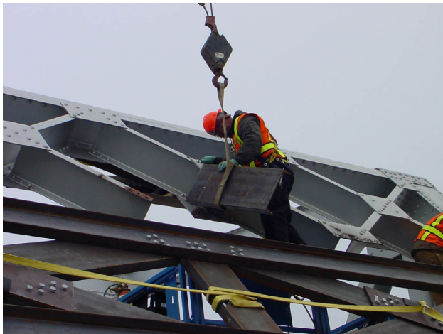
Figure 16: Installing New Member
