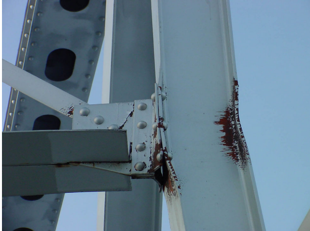
Figure 5: Connection of Sway Bracing to Truss
