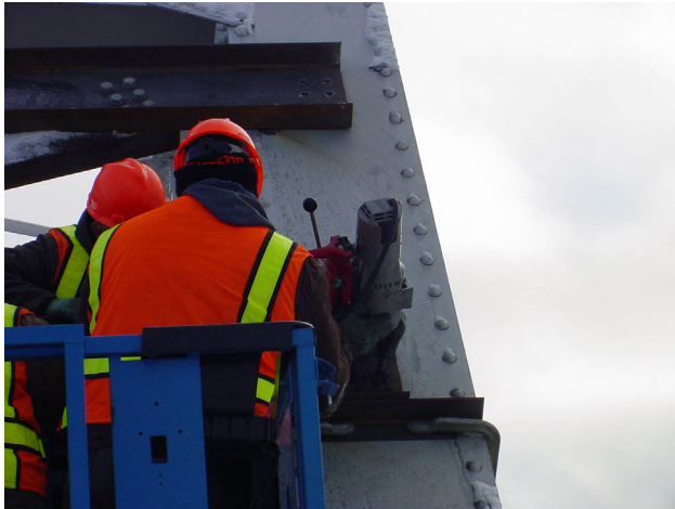
Figure 14: Drilling to Attach Temporary Portal to Truss
