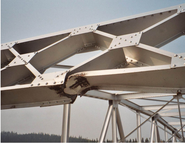
Figure 2: Severed Lower Chord in Span 4 Far End Portal
