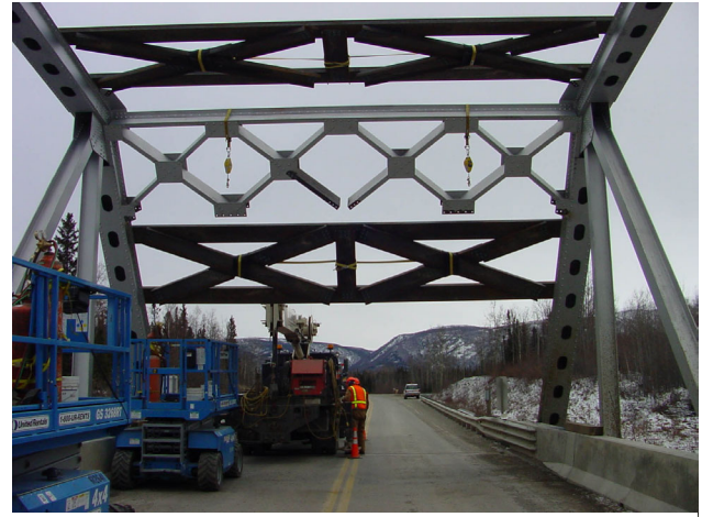
Figure 15: Damaged Section Removed
