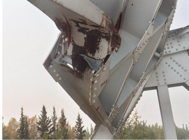
Figure 3: Severed Lower Chord in Span 5 Far End Portal
