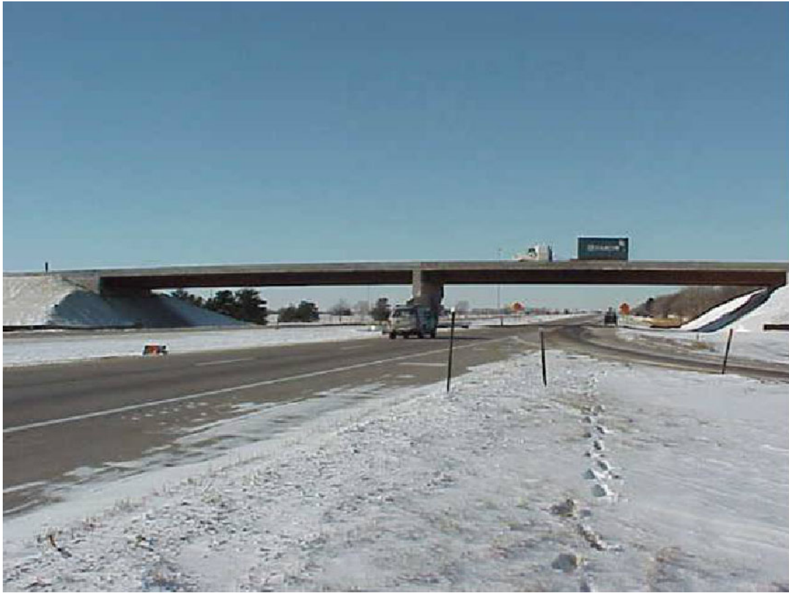
Figure 8- Picture of Completed Bridge
