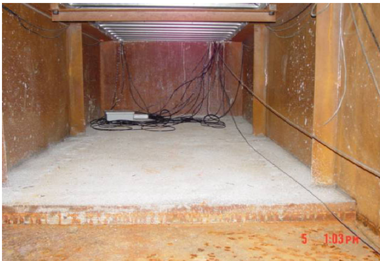
Figure 7– Inside the Box Girder near Pier
