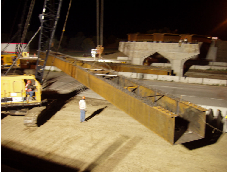
Figure 6- One of the Girders During Placement over the
