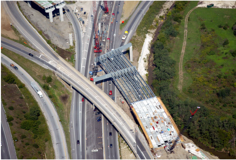
Figure 4. Steel capbeams over U.S. 71 (Bridge A6249)
