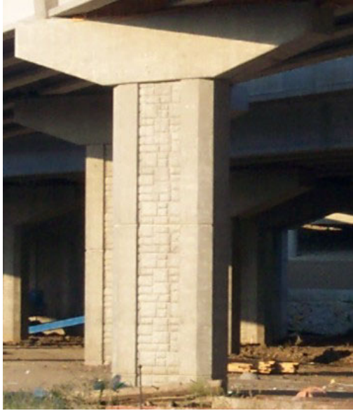
Figure 5. Aesthetic treatments of pier
