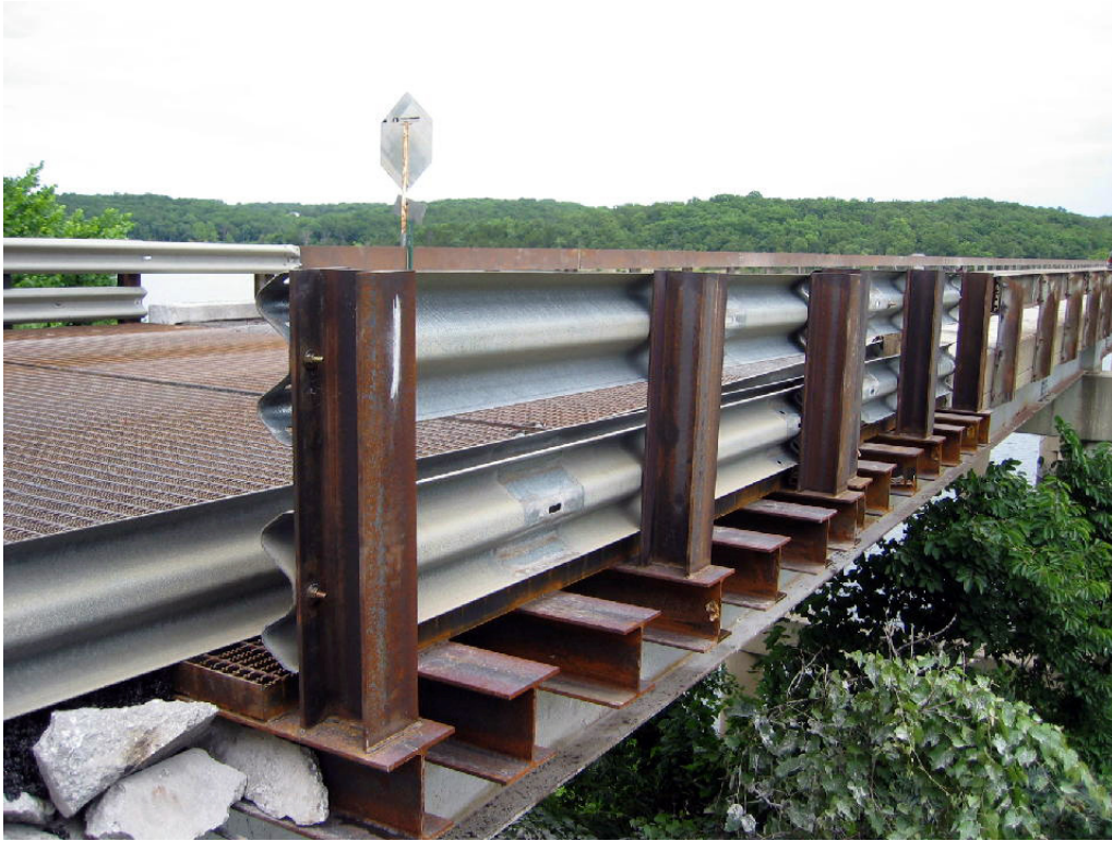
Figure 4. Temporary Deck Panel
