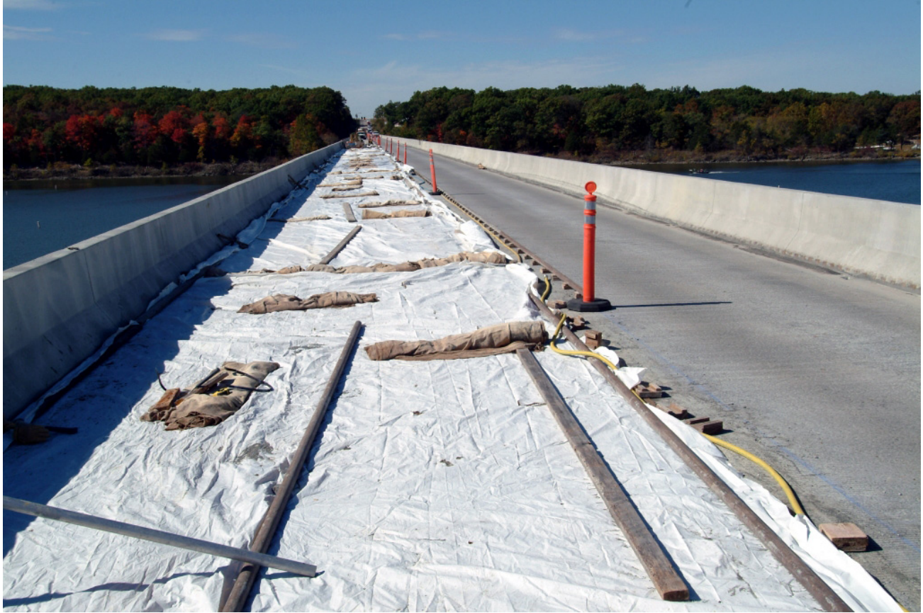
Figure 5. Stage Construction at End of Project
