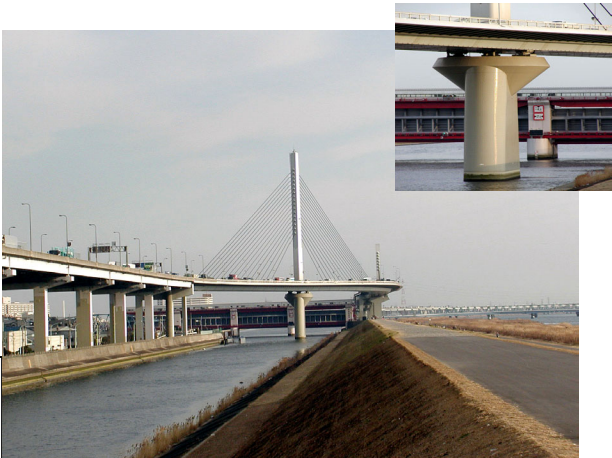
Katsushika Harp Bridge Tokyo, Japan is fluoropolymer protected. Steel coated 1985; Concrete coated 1987.
