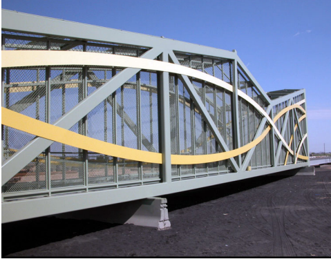
Maryland Avenue Pedestrian Bridge over I-17, Phoenix, AZ coated with Fluorourethane finish to preserve the color scheme in the intense Arizona sun.
