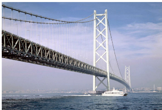
Akashi – Kaikyo Bridge, Kobe, Japan protected with inorganic zinc primer, epoxy intermediate coat and fluoropolymer finish. This is routine system for bridges in Japan.
