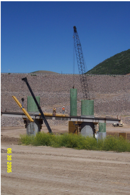
Photo 4: Splicing column cage
