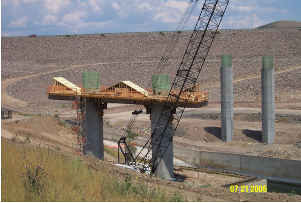
Photo 5: Forming Pier 2 cap.
