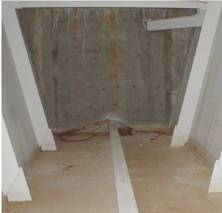
Figure 5. Lateral bracing and longitudinal stiffeners cast into the diaphragm.
