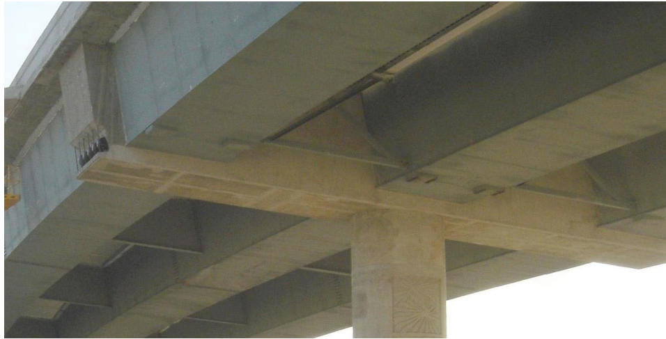
Figure 2. Integral concrete diaphragm at Pier No. 3
