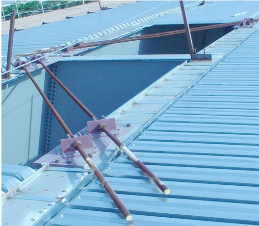
Figure 8. Temporary horizontal bracing.
