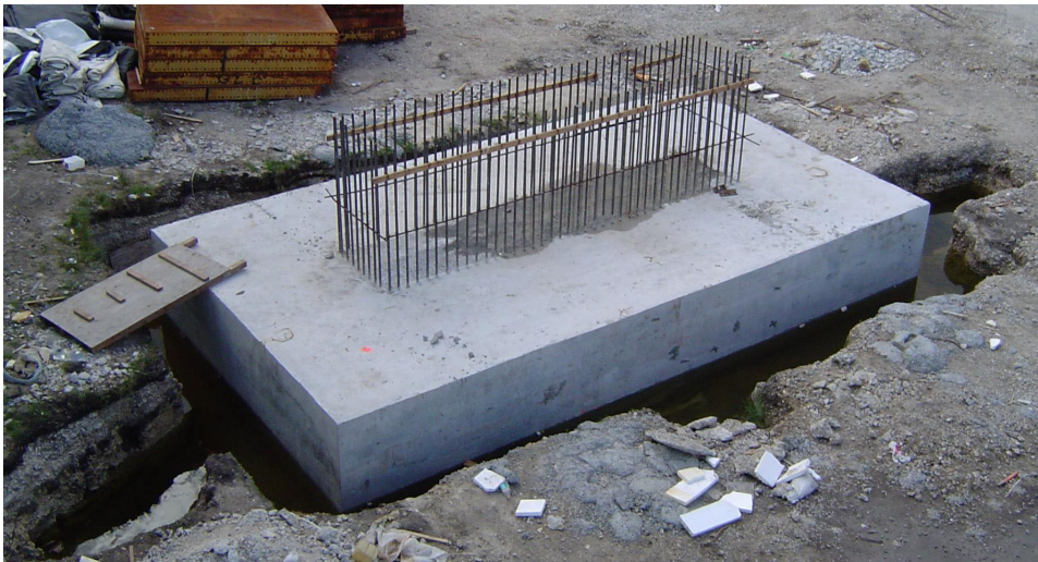
Figure 12. Spread footing at Pier No. 2.
