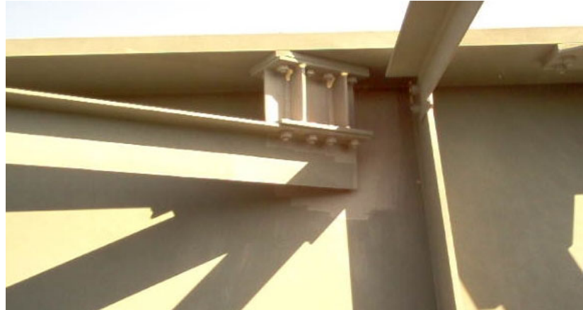
Figure 6. Lateral bracing bolster at the integral diaphragm.
