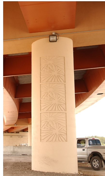
Figure 9. Surface texture on pier column.
