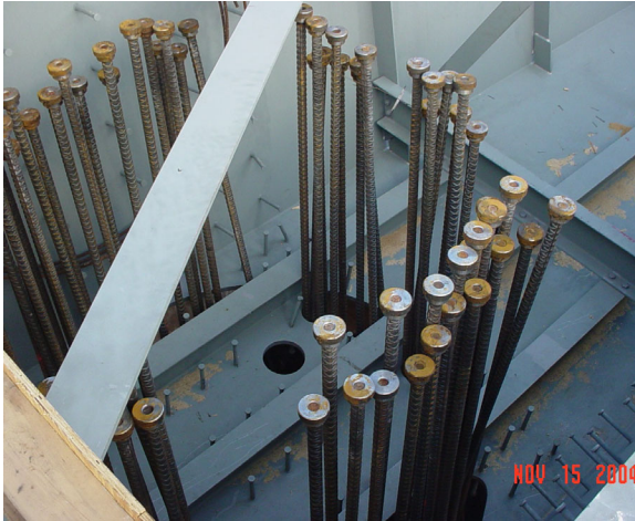
Figure 4. Pier reinforcing extending into integral diaphragm.
