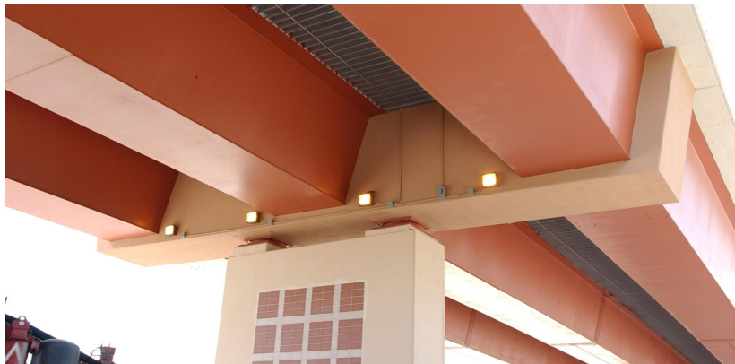
Figure 11. Integral diaphragm at Pier No. 2.
