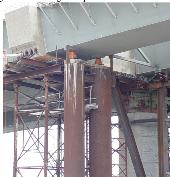
Figure 7. Temporary shoring at pier.
