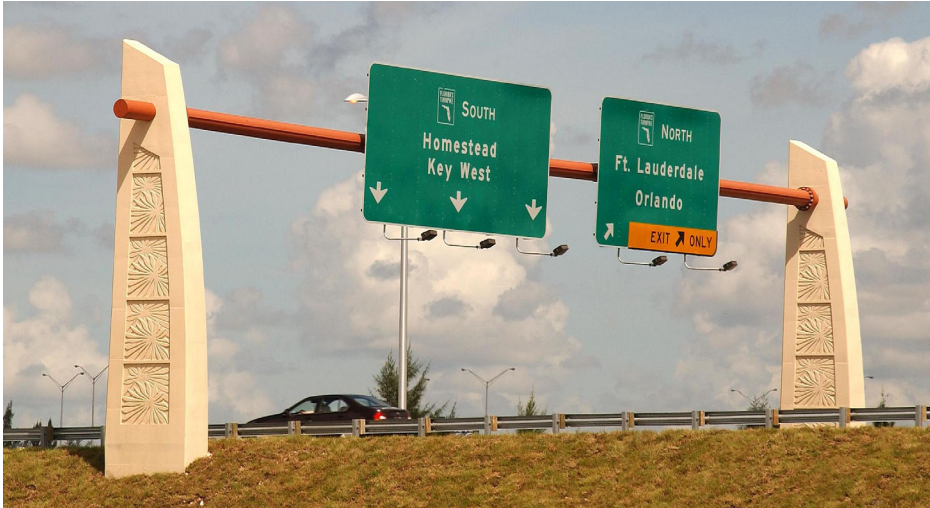
Figure 13. Typical span-type sign structure.
