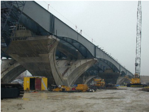
FIGURE 5: Construction of the Virginia Spans Showing Completed V-Piers and Girders
