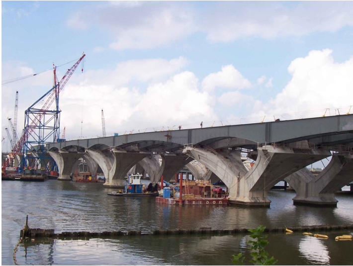
FIGURE 4: Construction of the Woodrow Wilson Memorial Bridge.
