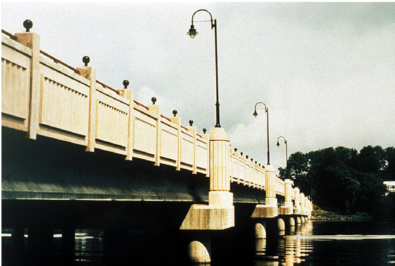
Fig. 2. Adding historical detail to an ordinary bridge
