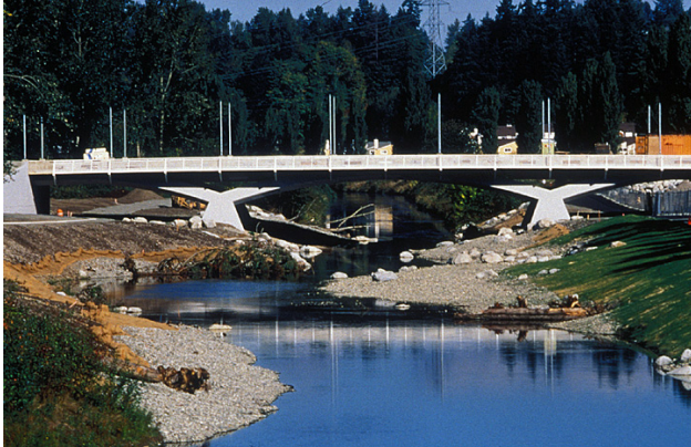
Fig. 16. 95 th Street Bridge
