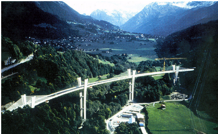
Figure 10. Menn's Sunniberg Bridge
