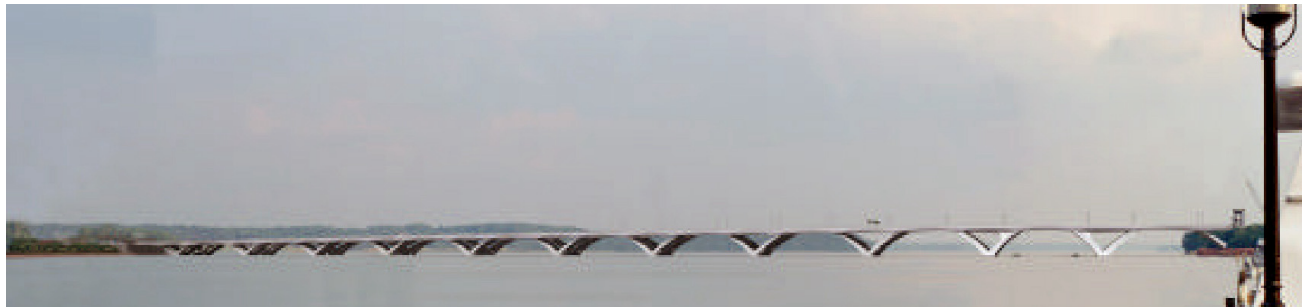
Figure 20. Woodrow Wilson Bridge
