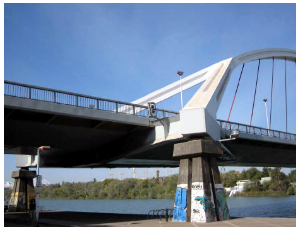
Fig. 19. Tie Details at the Piers
