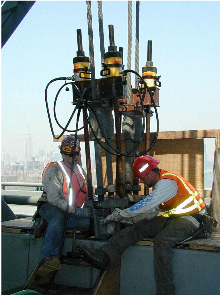
Figure 5. Suspender adjustment showing the two cable suspenders with tension rods being jacked.
