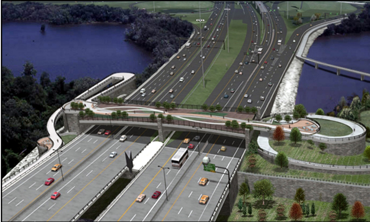
Figure 6: Rosalie Island, Group 4 Bridges, looking Northeast
