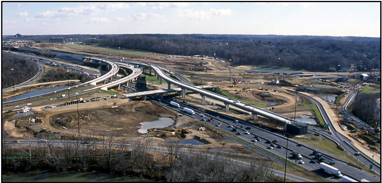
Figure 3: I-95/I-295 Interchange Under Construction, looking Southeast
