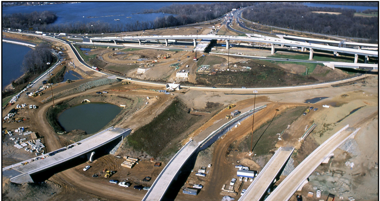
Figure 5: I-95/I-295 Interchange Group 3 Bridges, looking North
