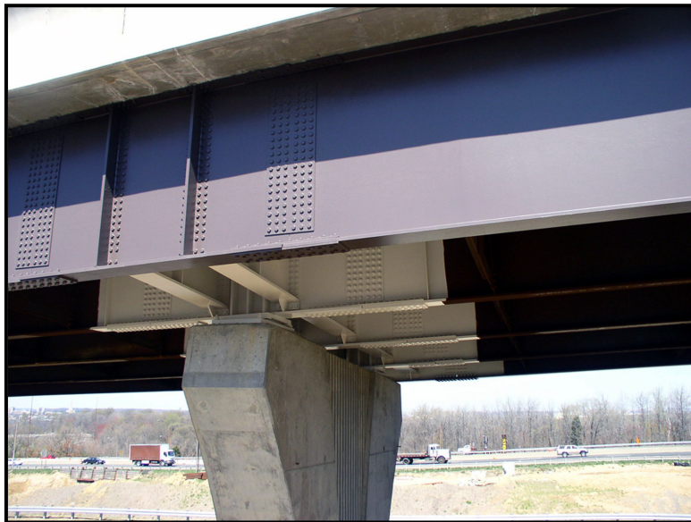
Figure 8: Steel Integral Pier Cap
