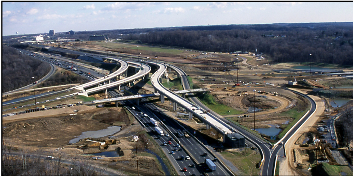
Figure 4: I-95/I-295 Interchange Group 1 Bridges, looking East
