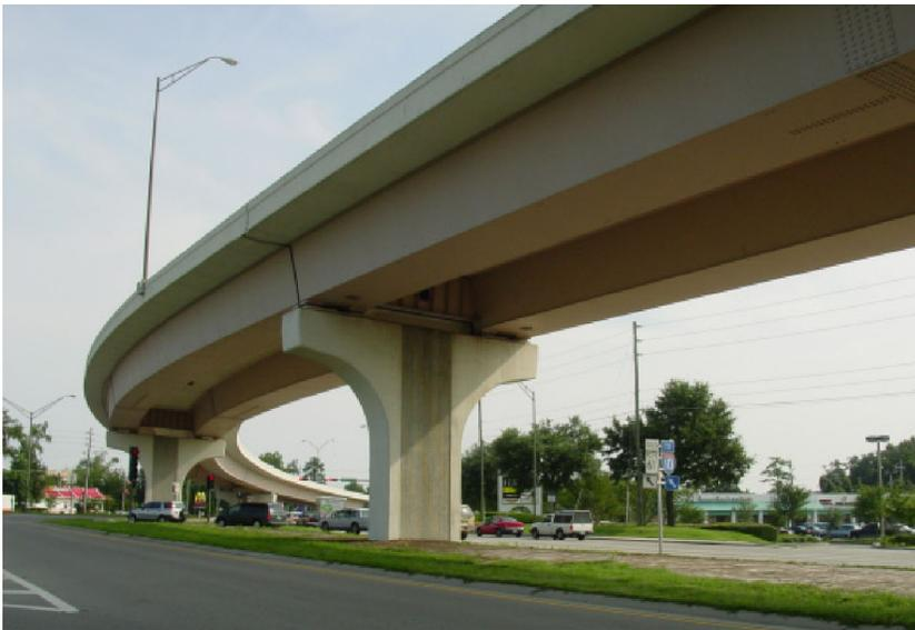
Figure 1: Curved Steel Box Girder Bridge
